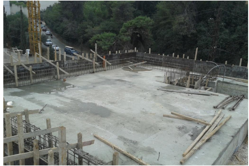
SLAB ROOF BLOCK B
