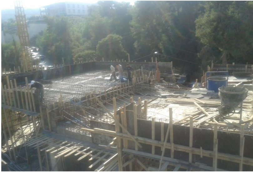
SLAB ROOF BLOCK B
