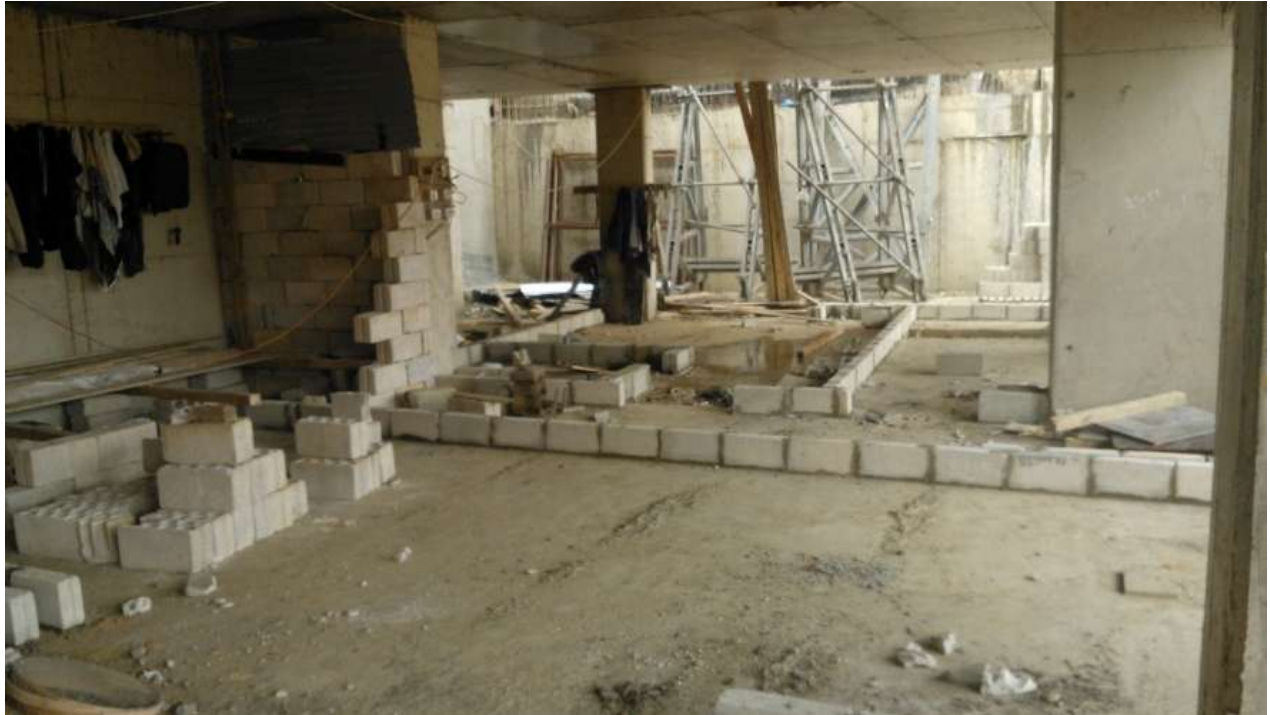
Figure 6-Block work for level 1
