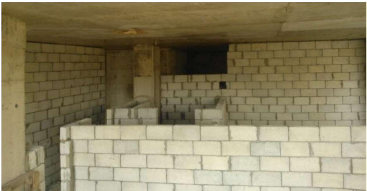
Figure 3-Block work for level 2
