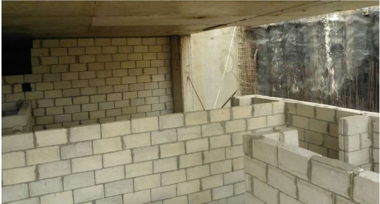
Figure 2-Block work for level 2
