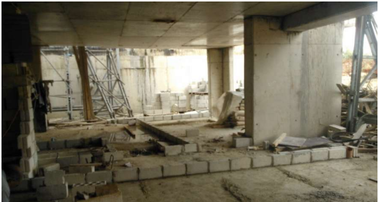
Figure 5-Block work for level 1
