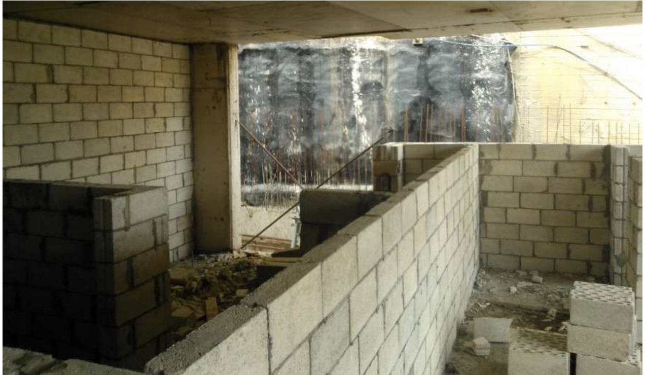
Figure 4-Block work for level 2
