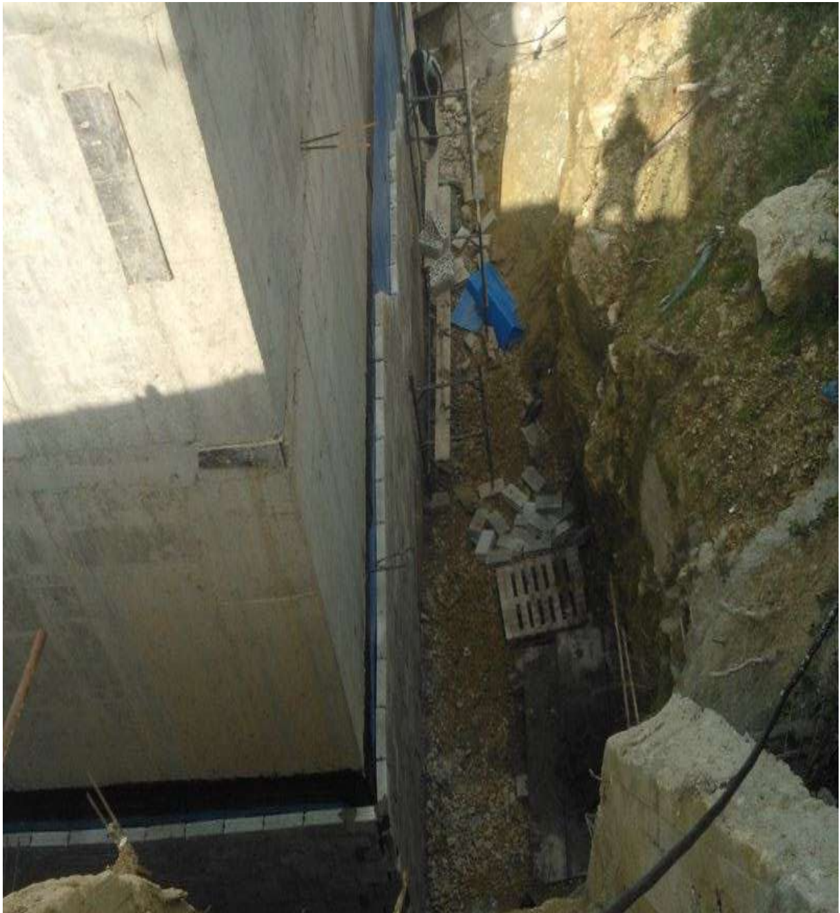
Figure 4-Waterproofing for basement walls
