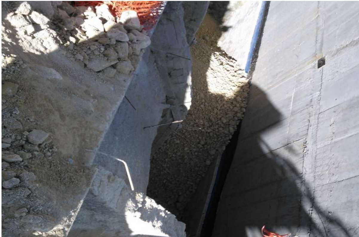
Figure 5-Backfill
