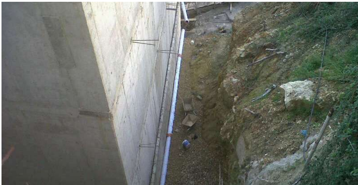
Figure 3-Installation of drainage pipe
