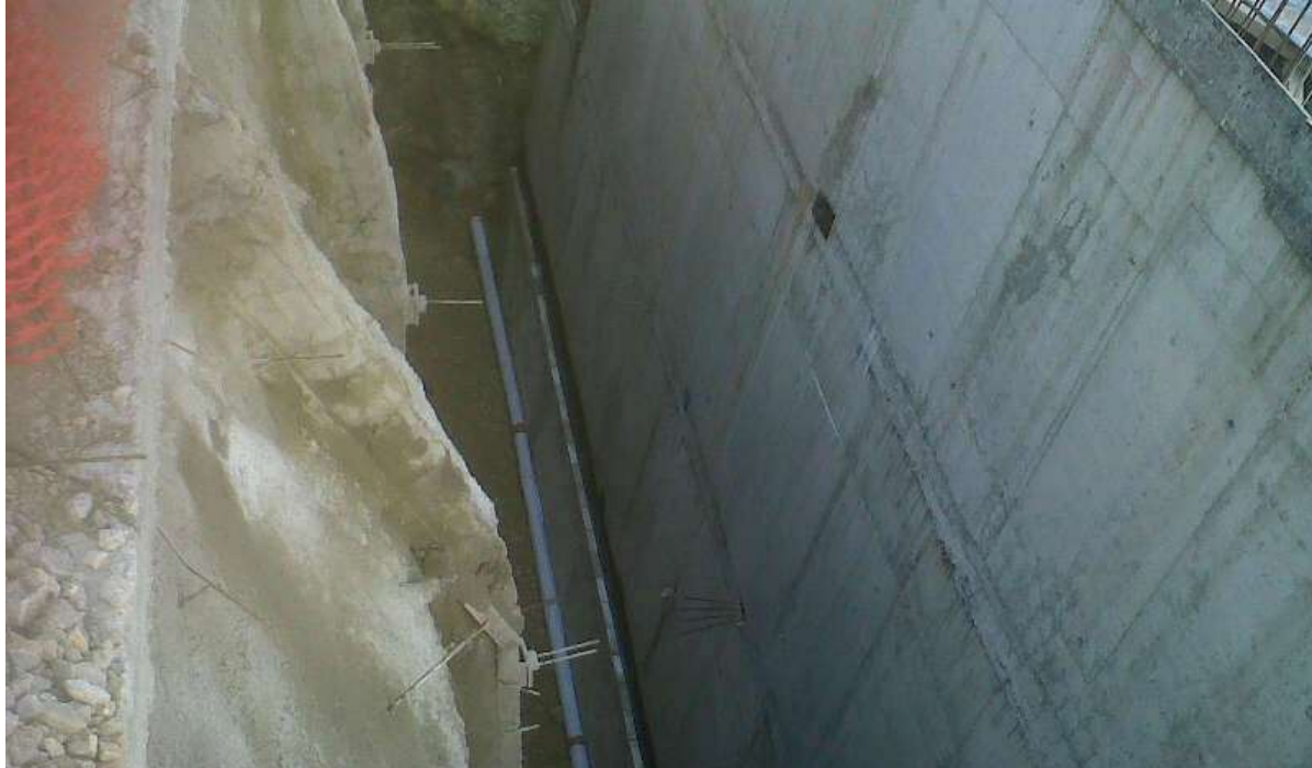
Figure 2-Installation of drainage pipe
