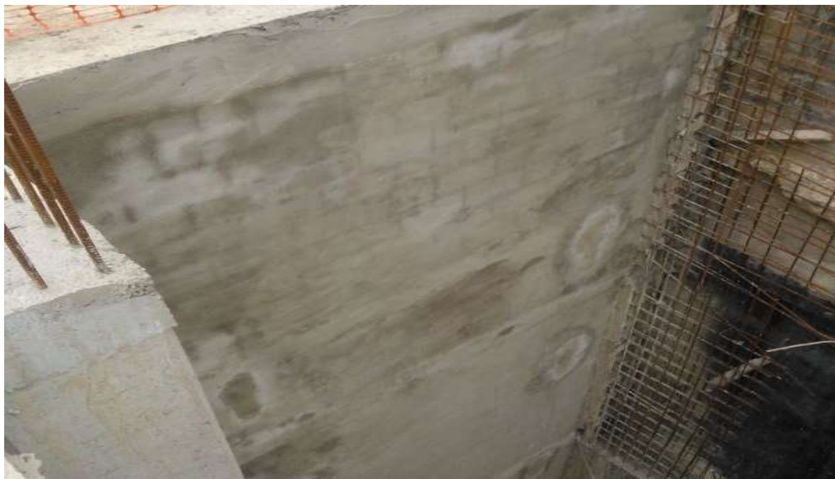
Figure 5- Installation and plastering of hollow block Wall block A
