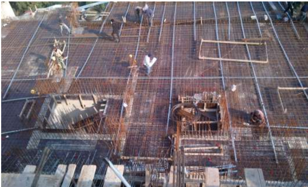
Figure 3-Reinforcement for level 3 slab
