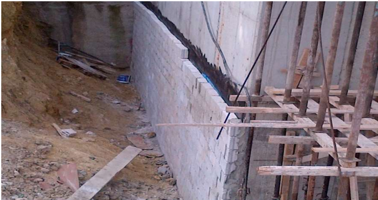
Figure 11-Waterproofing and block installation for basement walls
