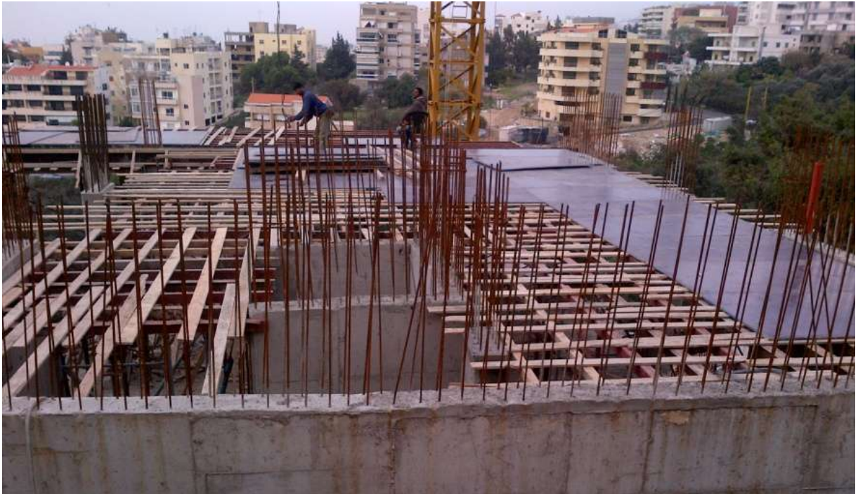
Figure 8-Formwork for slab level 0
