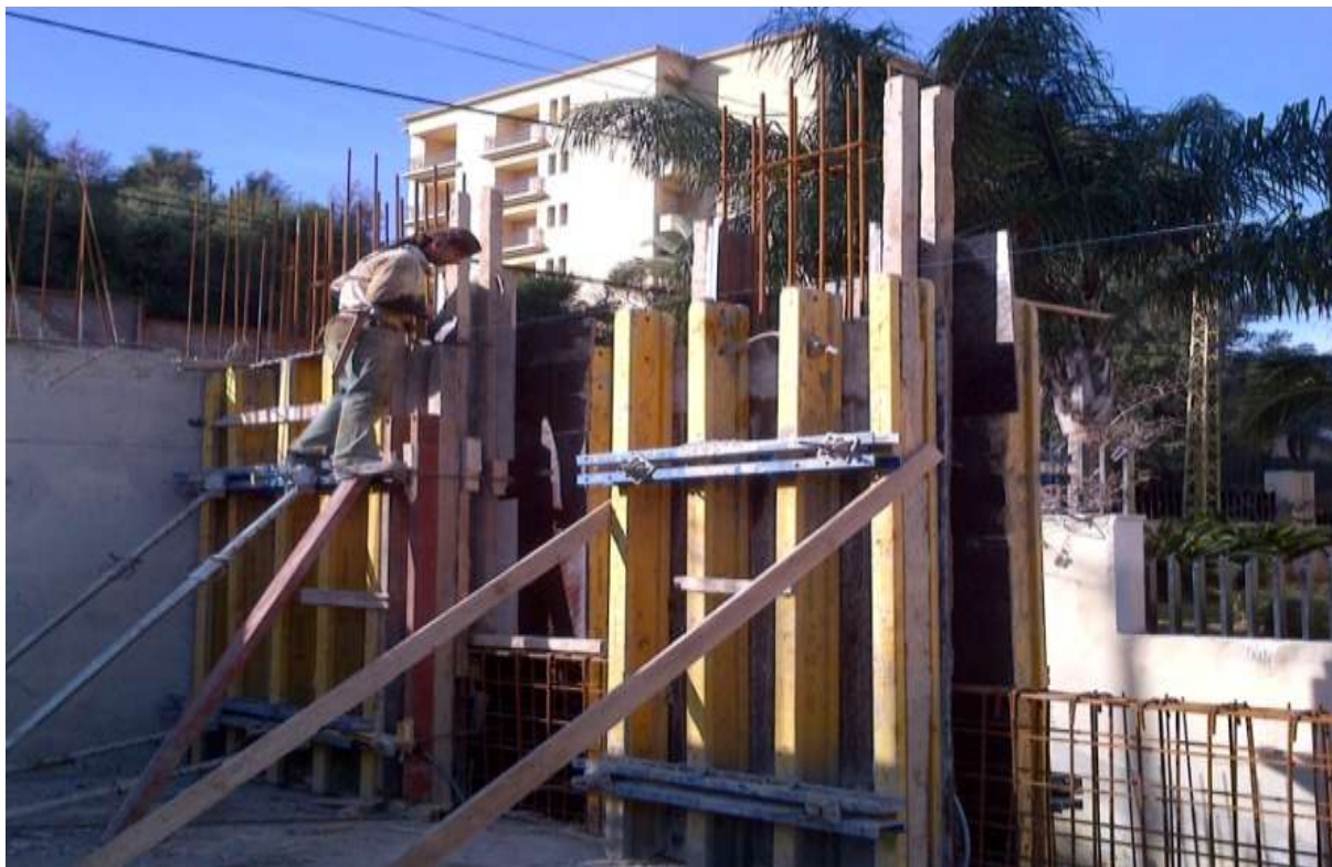
Figure 7-Formwork for columns garden floor
