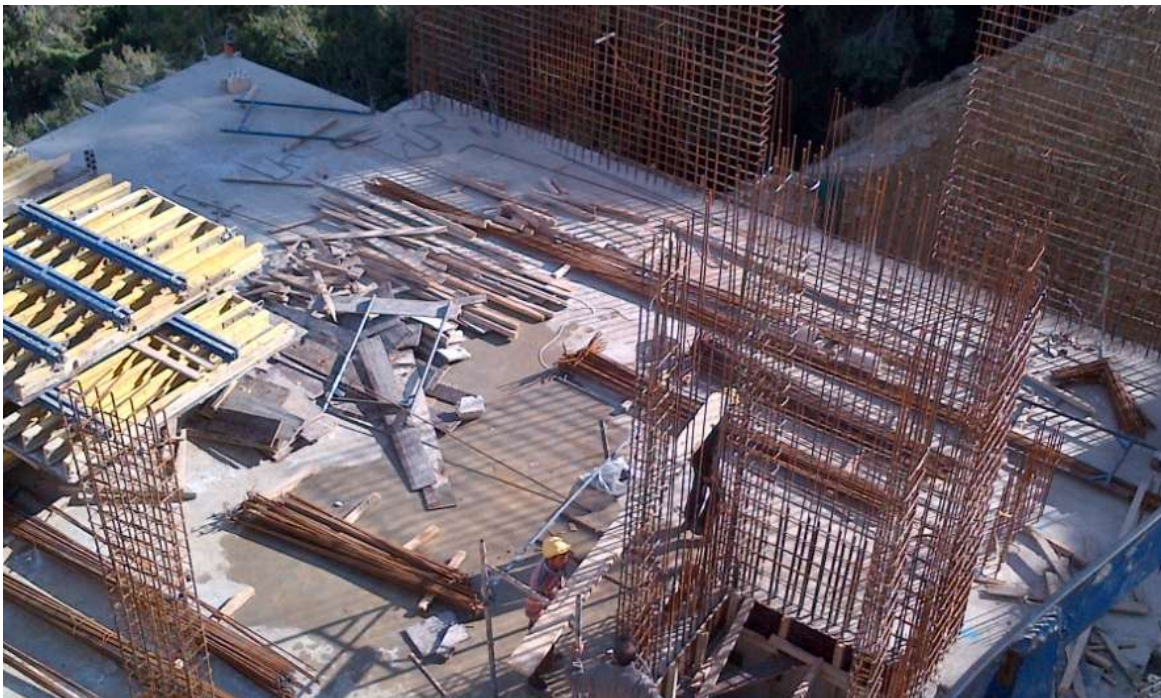
Figure 5-Steel works for core and basement walls level 3
