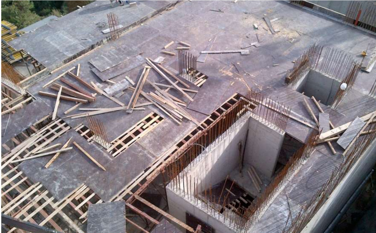
Figure 10-Formwork for slab level 0
