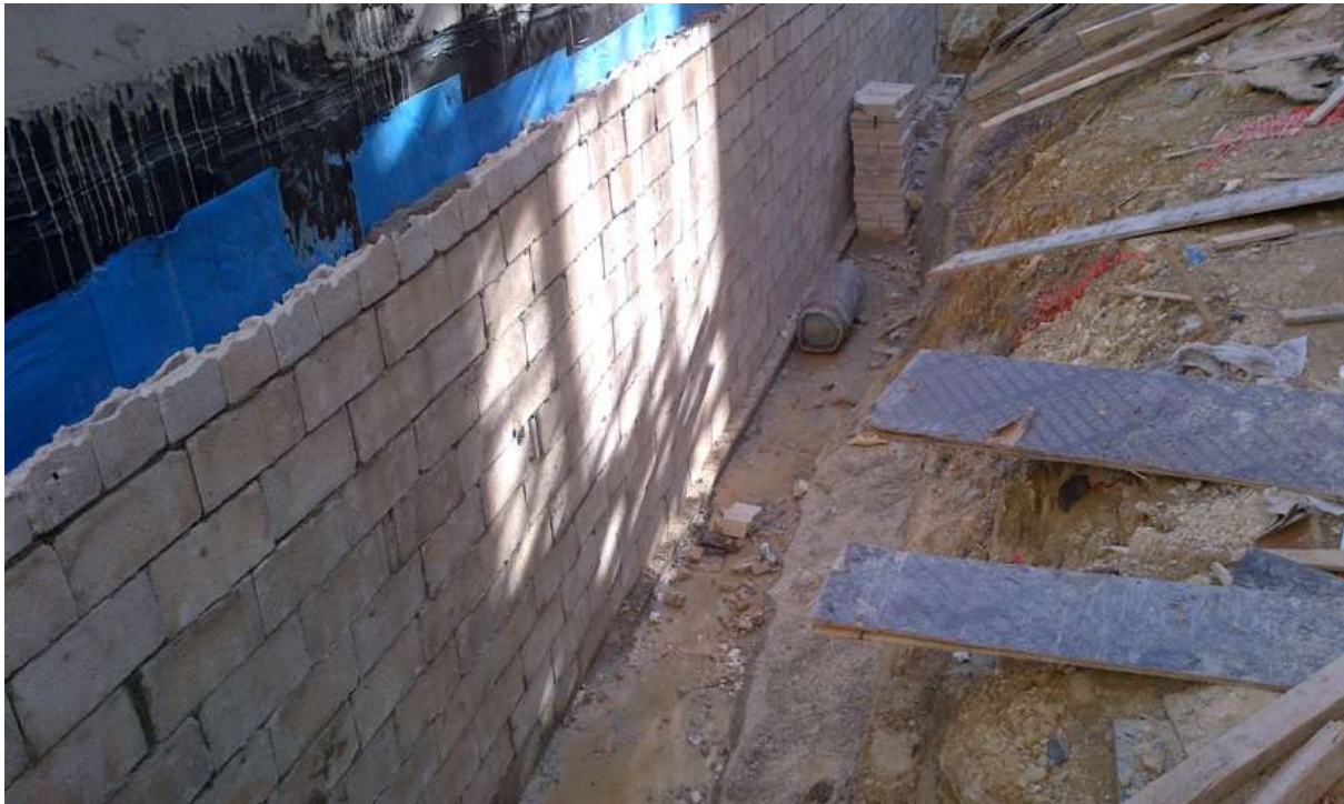
Figure 6-Waterproofing and block installation for basement walls
