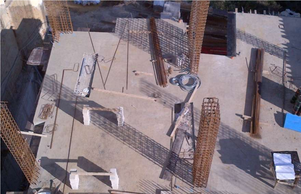
Figure 4-Steel works for columns level 3
