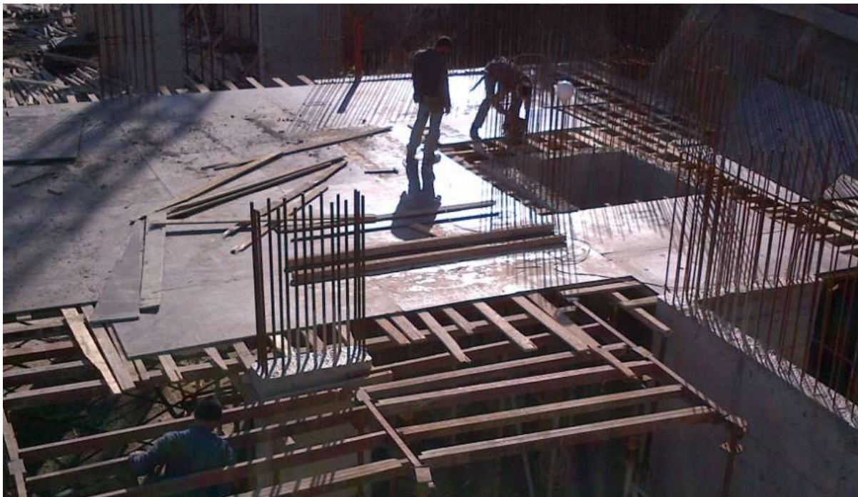
Figure 9-Formwork for slab level 0
