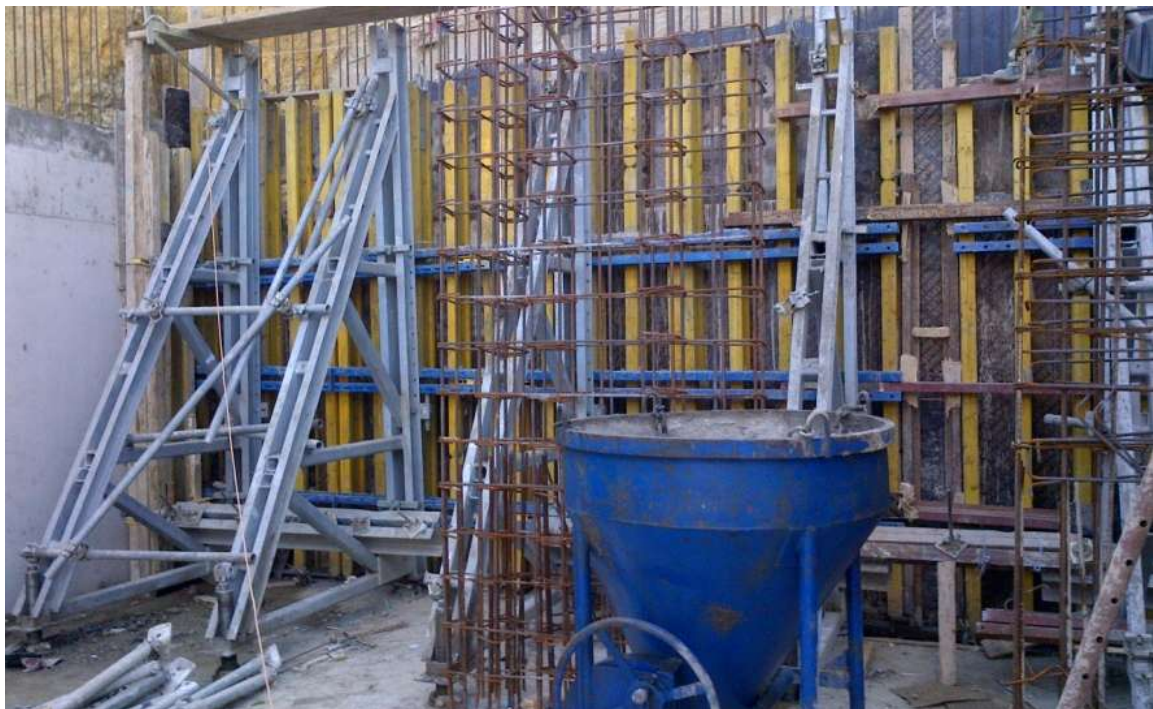
Figure 7-Formwork for wall level 1
