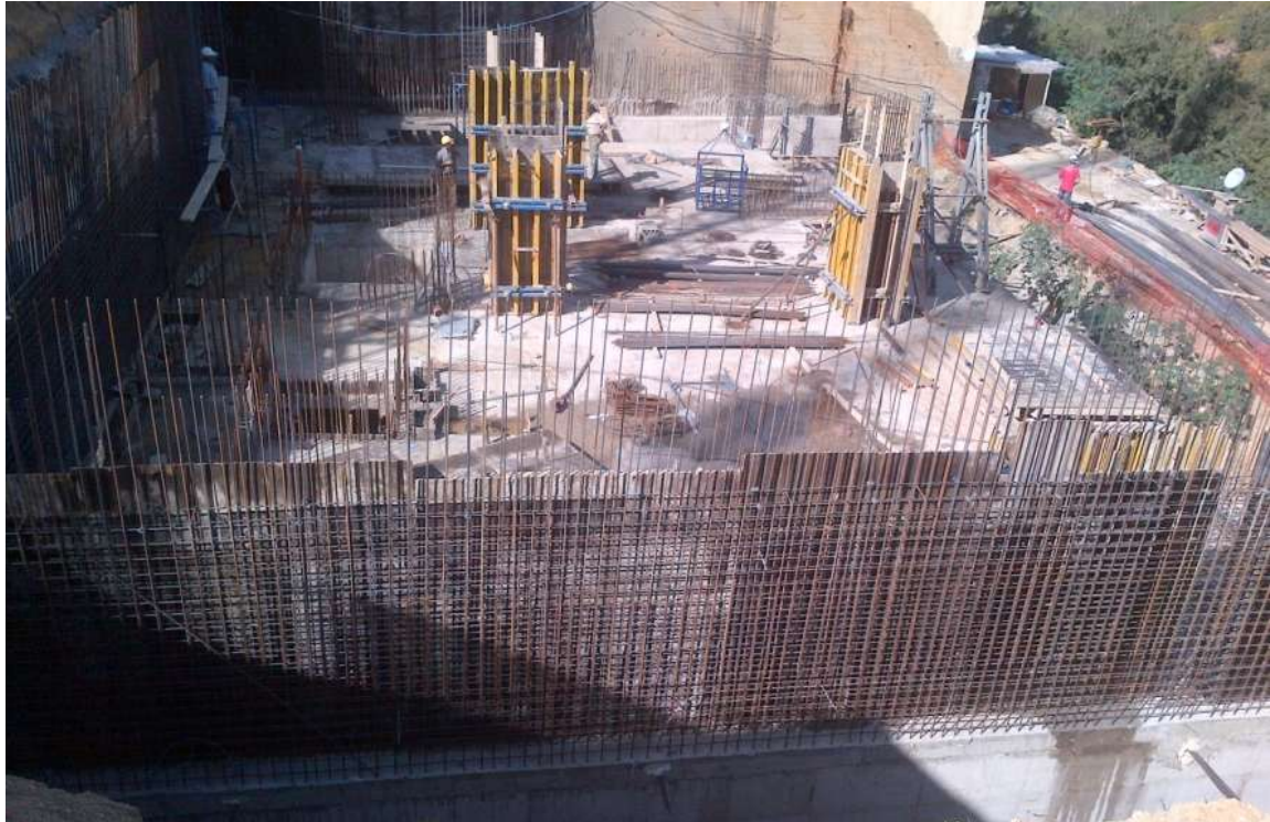
Figure 6-Works on level 1 slab
