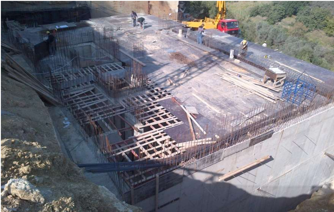
Figure 8-Formwork for level 2 slab
