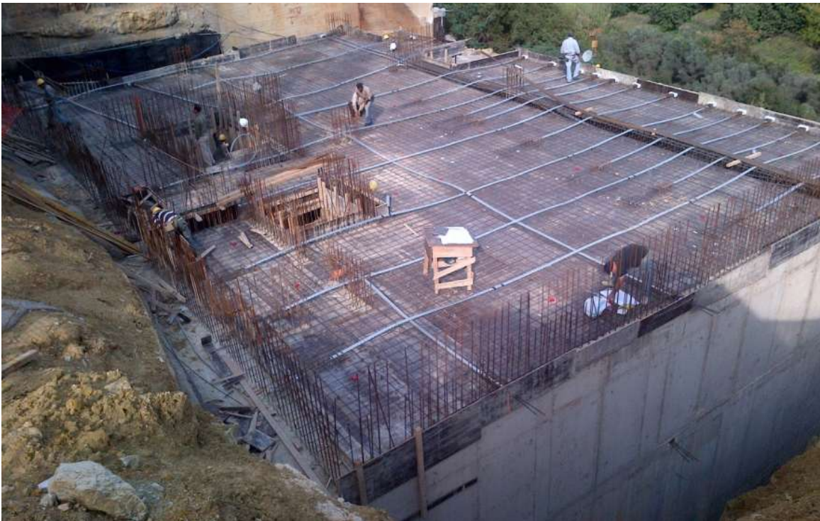
Figure 9-Reinforcement and PT works for level 2 slab
