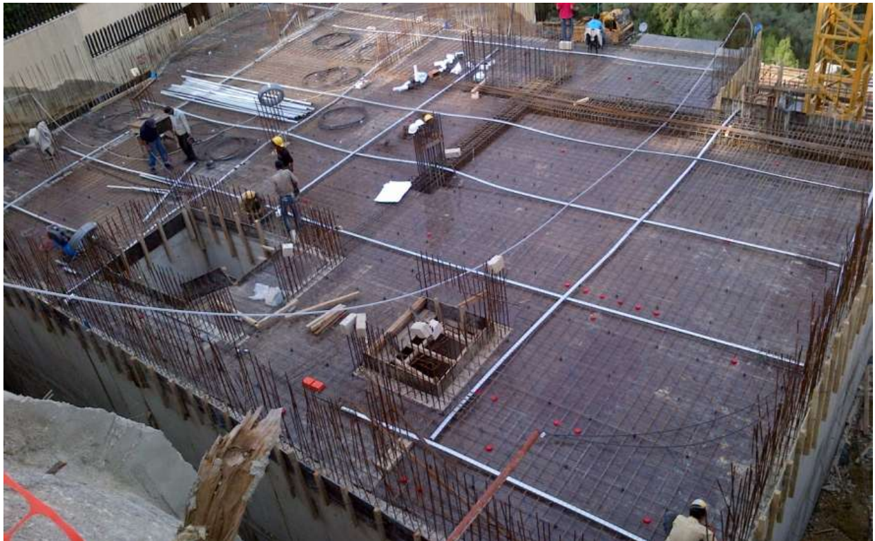
Figure 13-Reinforcement and PT works for garden floor slab
