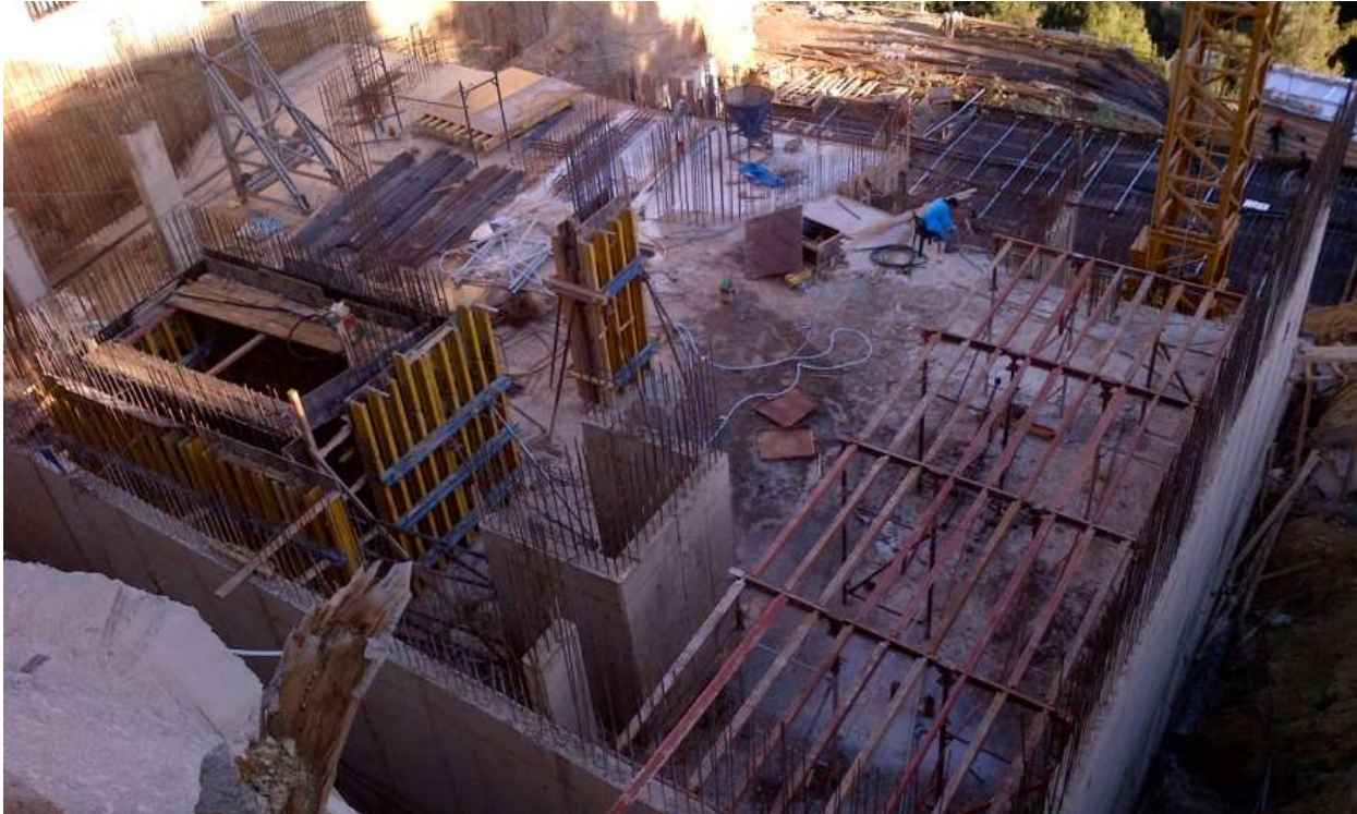
Figure 10-Work on garden floor slab
