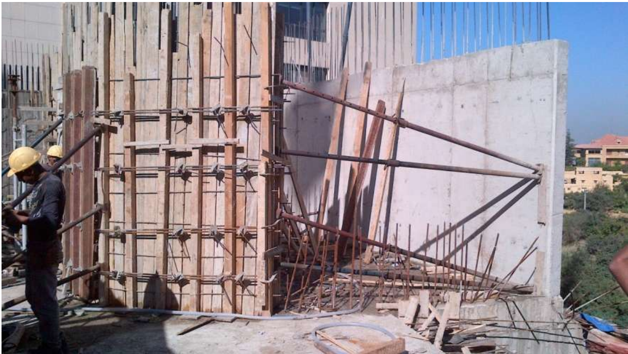
Figure 11-Formwork for ramp wall Garden Floor
