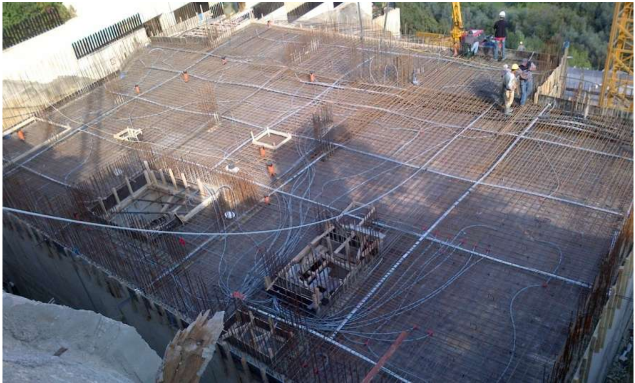
Figure 14-Reinforcement and PT works for garden floor slab
