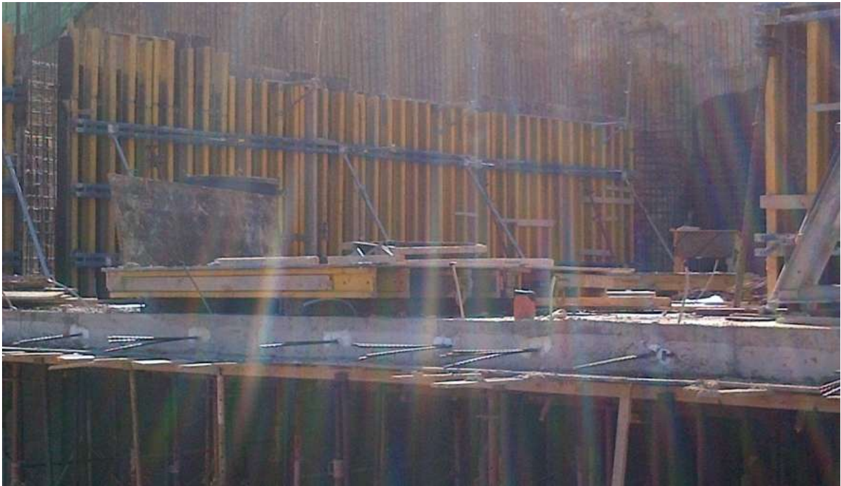
Figure 4-Formwork for wall level 1
