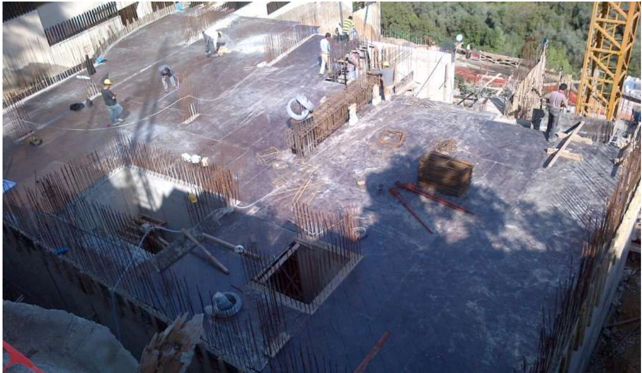
Figure 12-Formwork for garden floor slab
