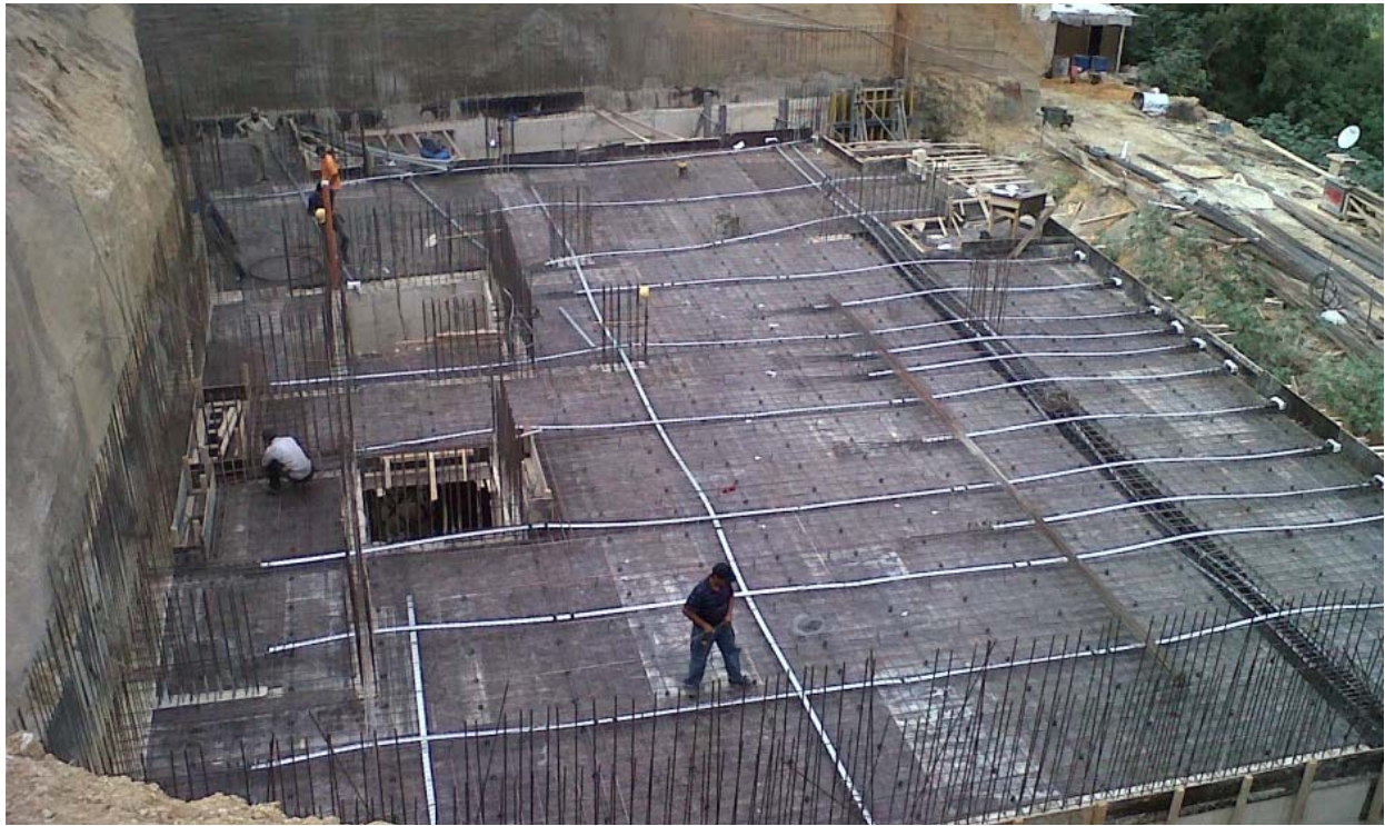
Figure 8-Post-tension for slab 1st floor
