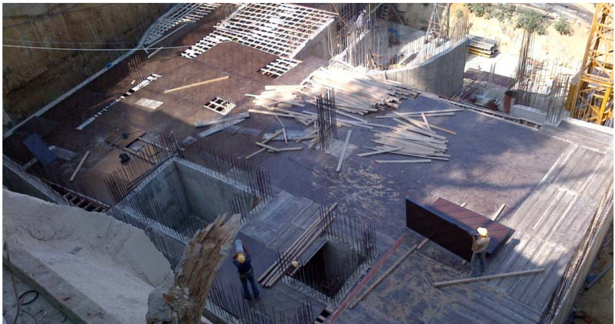
Figure 9-Formwork for slab basement 1
