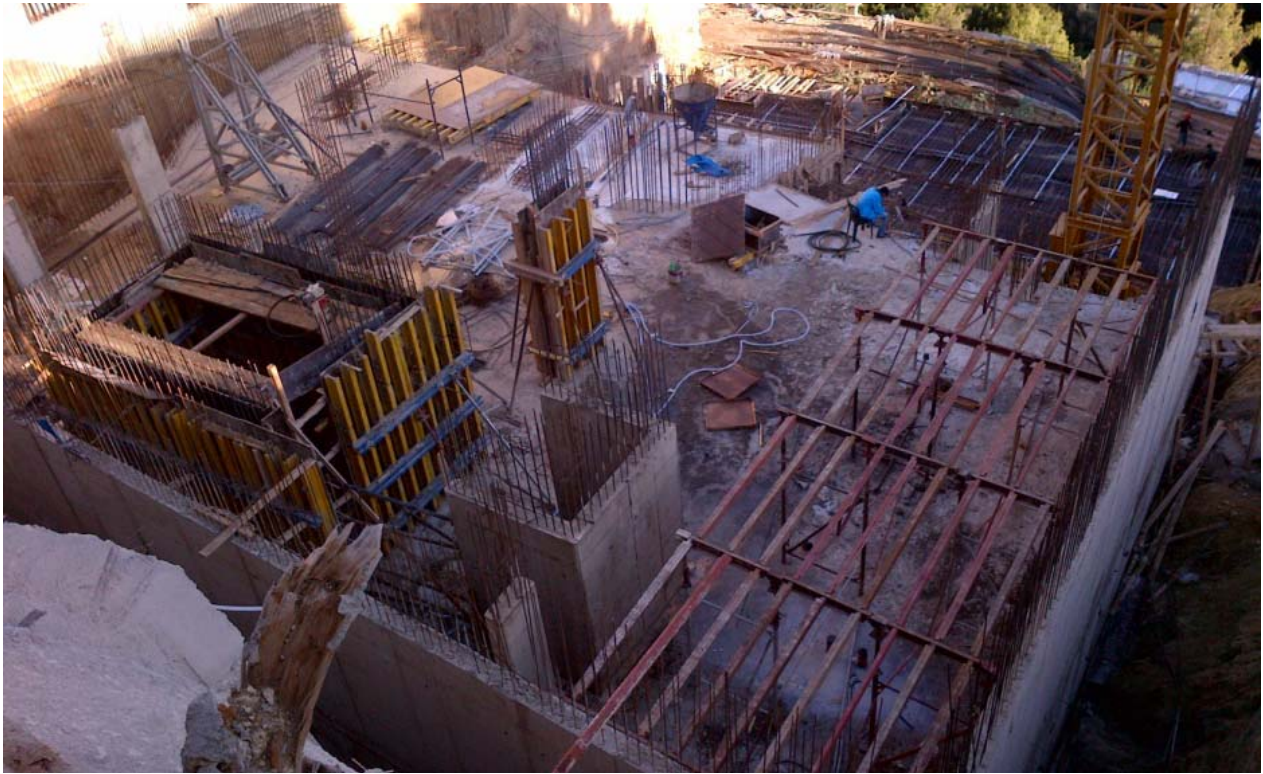
Figure 14-Formwork and steel work for vertical elements basement 1
