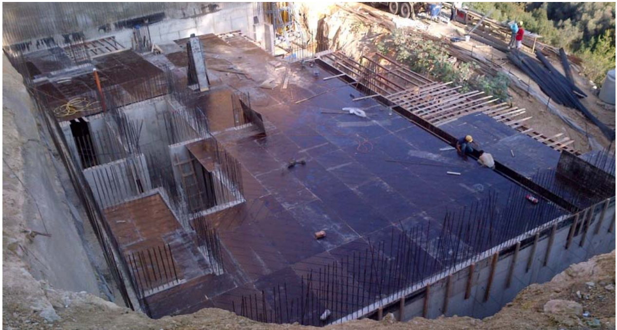
Figure 7-Formwork for slab 1st floor
