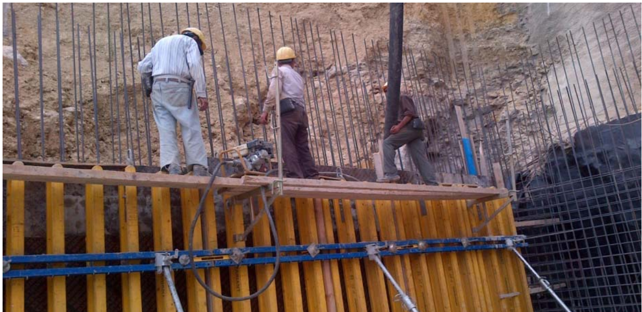
Figure 3-Pouring of wall Ground floor
