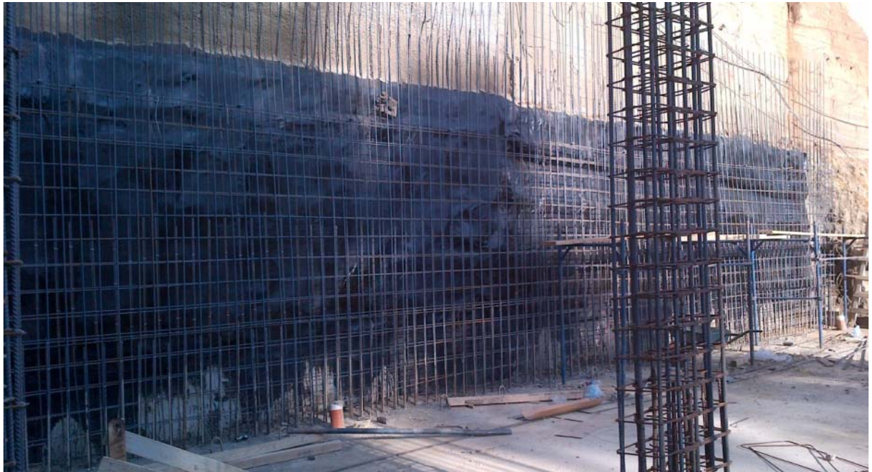
Figure 4-Steel work for wall Ground floor
