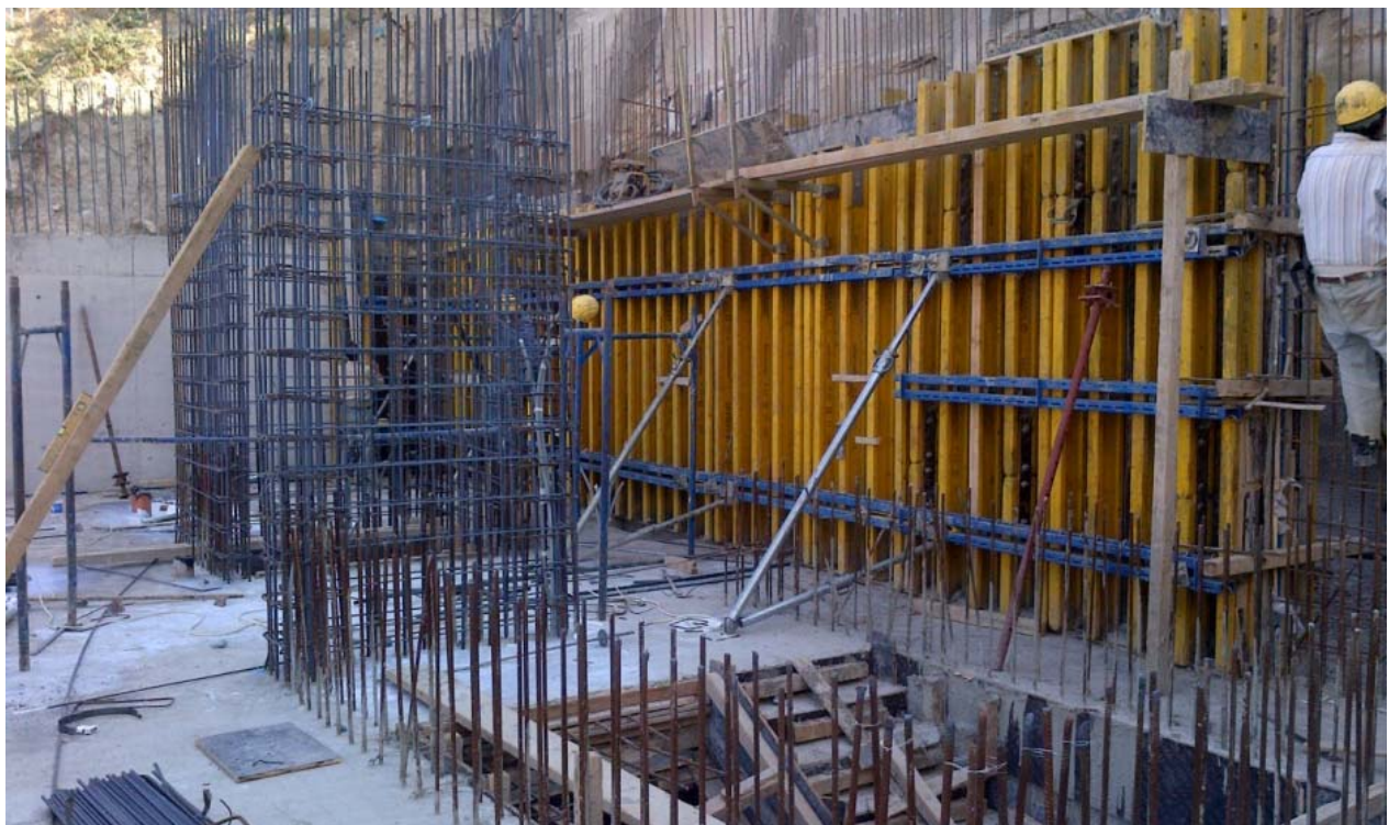
Figure 13-Steel and formwork for vertical elements basement 1
