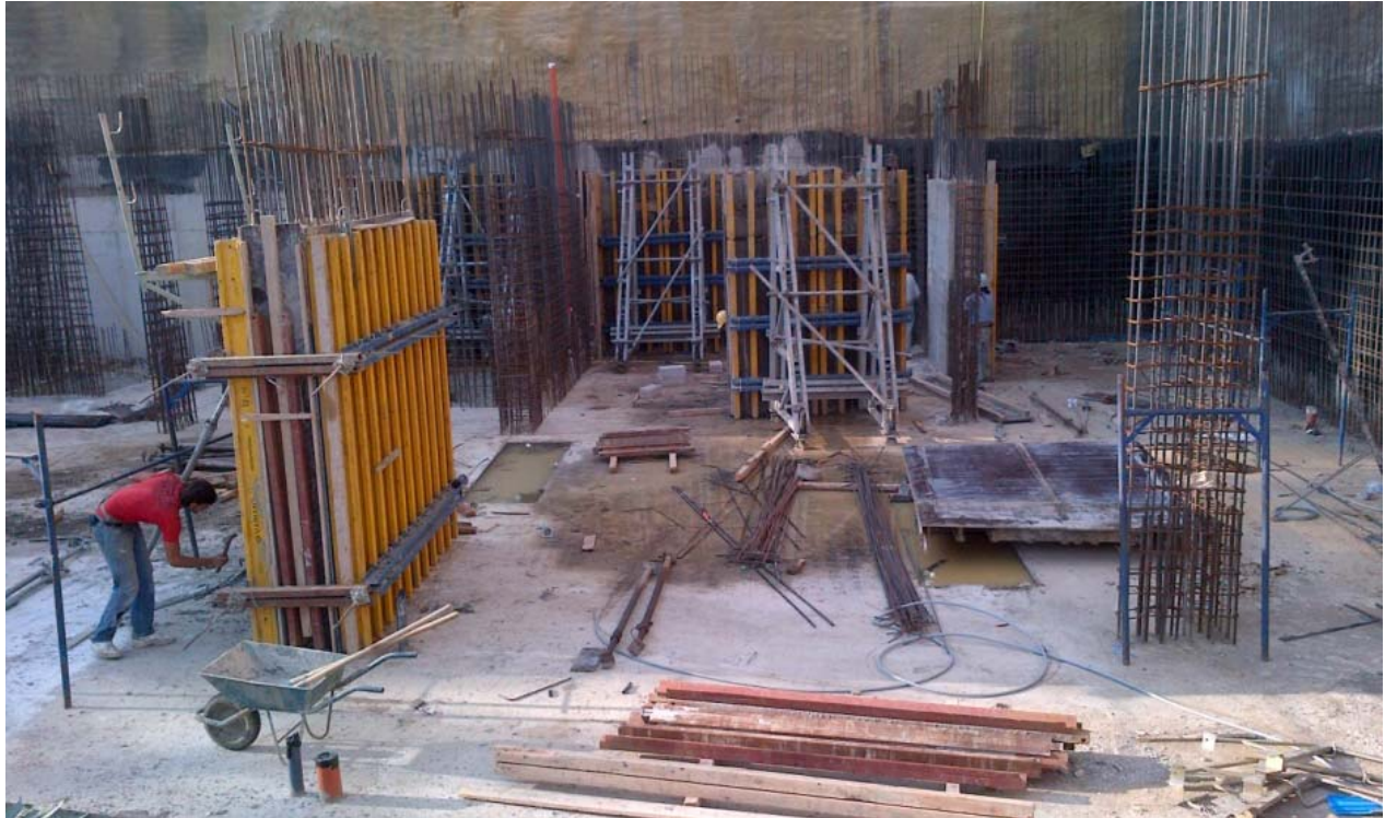
Figure 6-Steel work and formwork for vertical elements Ground floor
