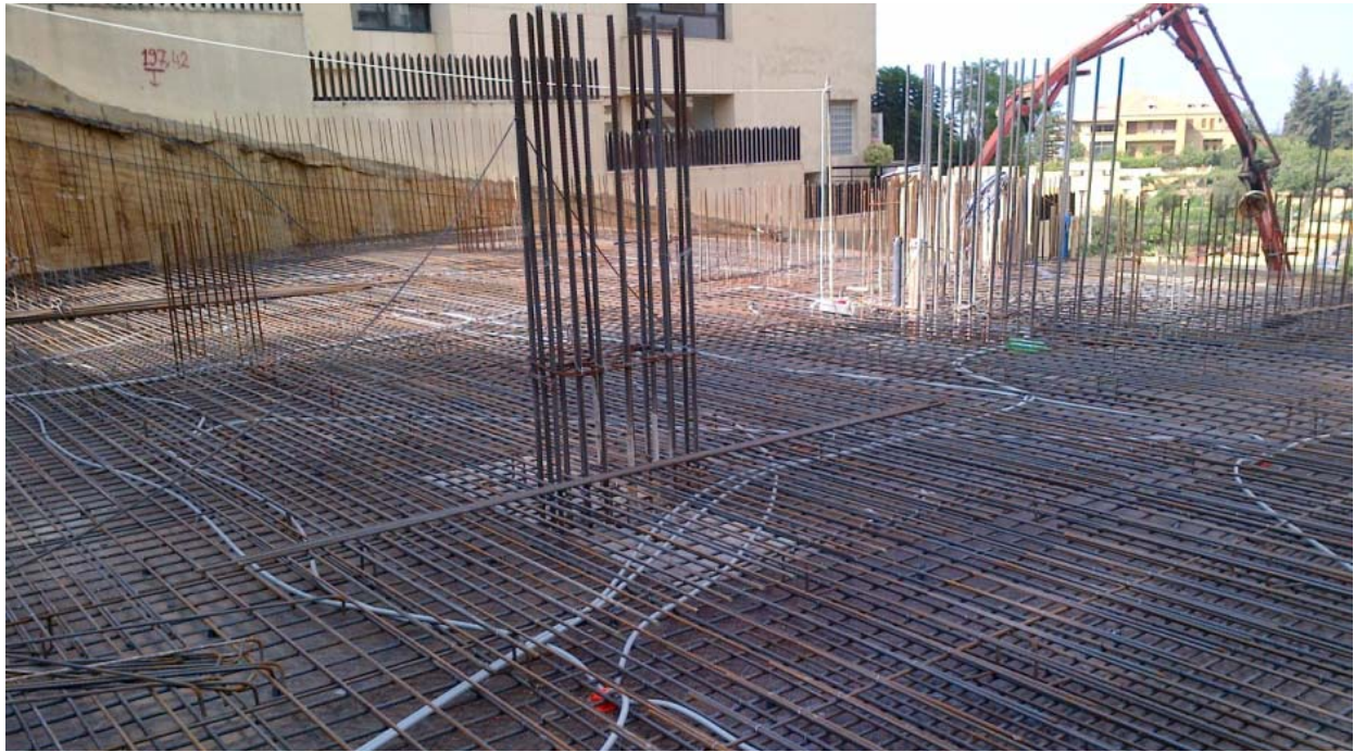
Figure 10-Steel and electrical works on slab basement 1
