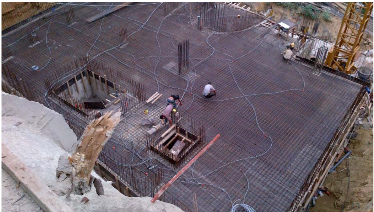
Figure 11-Steel works for slab basement 1
