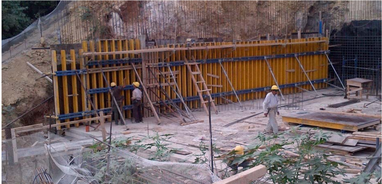
Figure 2-Formwork of Wall Ground floor
