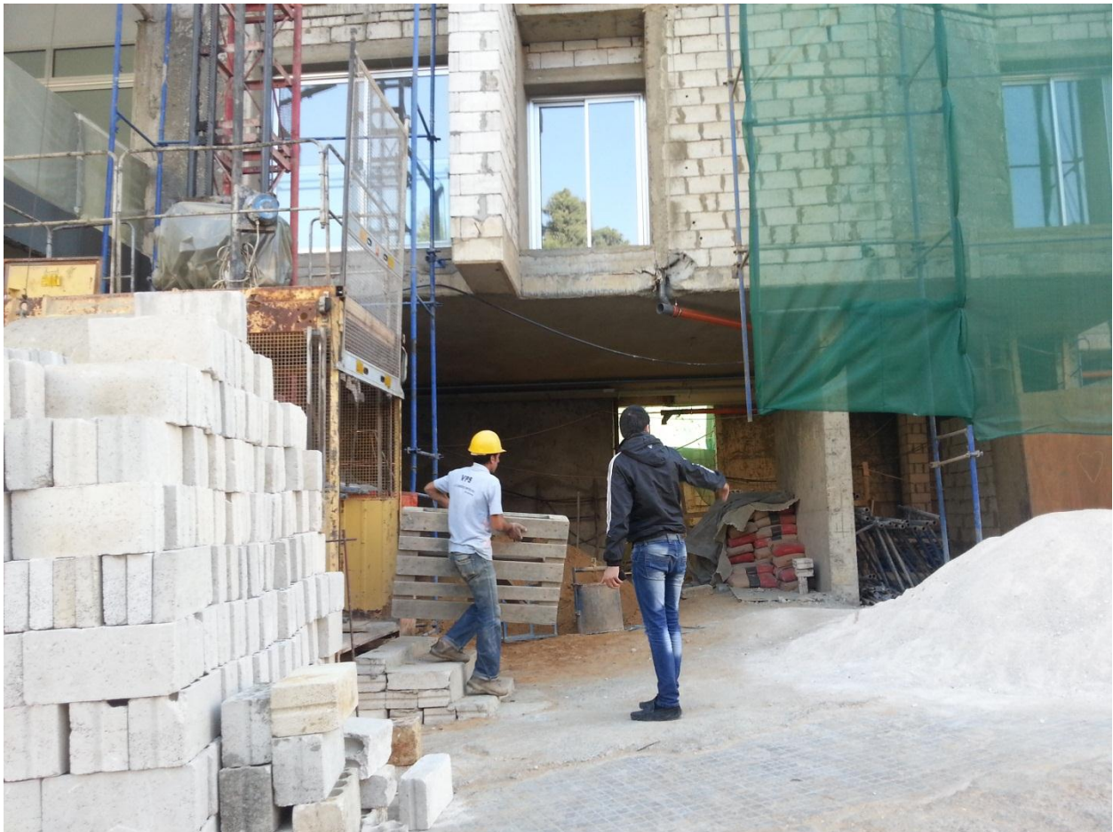
Ground Floor Work Progress
