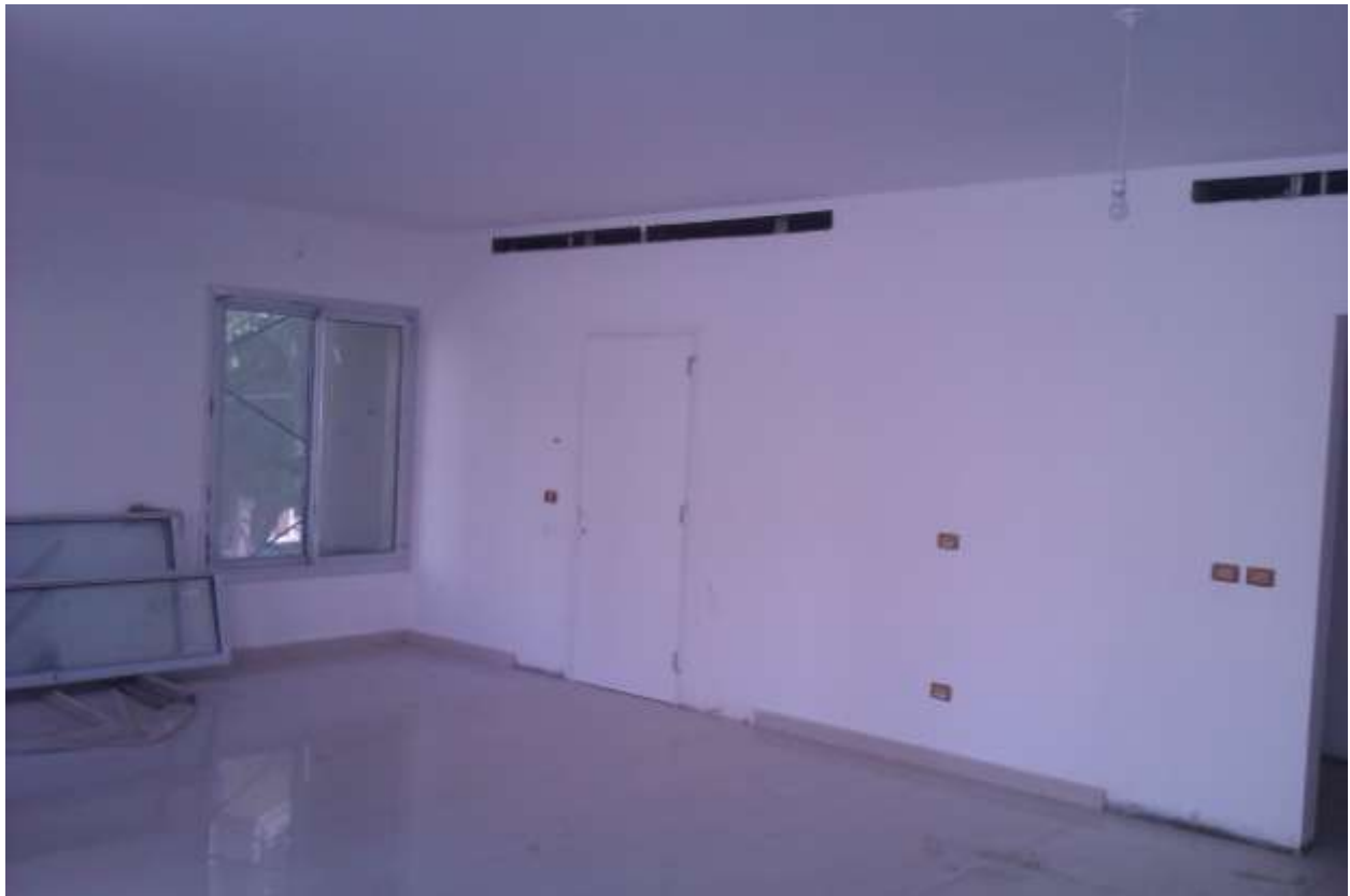
Work progress in the 1 st floor / mockup apartment
