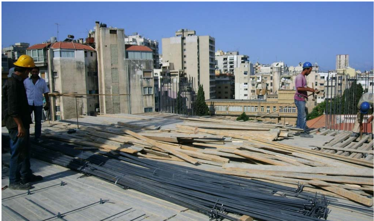
Figure 3: Preparation for pouring 6th floor slab
