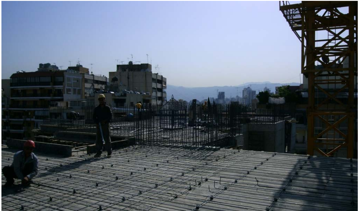
Figure 2: Preparation for pouring 6th floor slab
