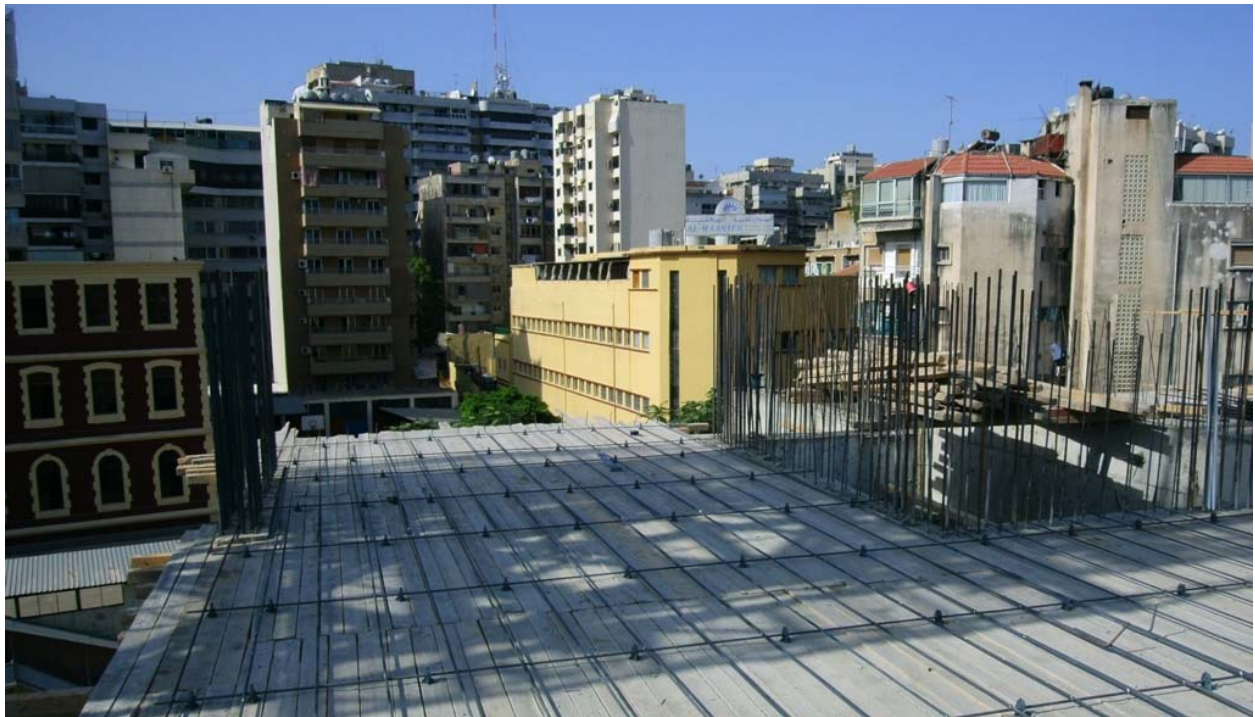
Figure 5: Preparation for pouring 6th floor slab
