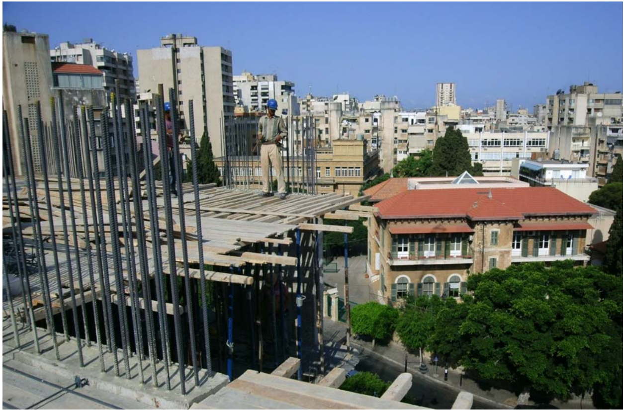
Figure 4: Preparation for pouring 6th floor slab
