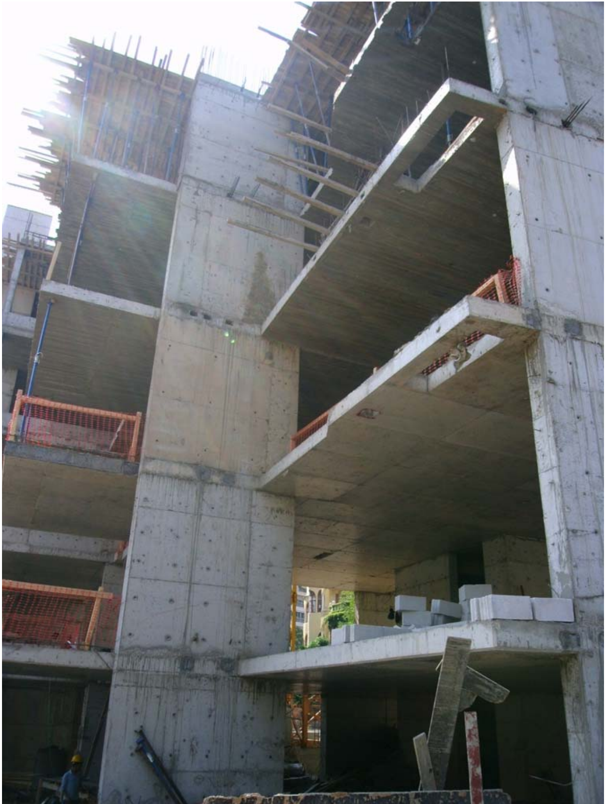
Figure 7: Preparation for blockwork @ 1st floor
