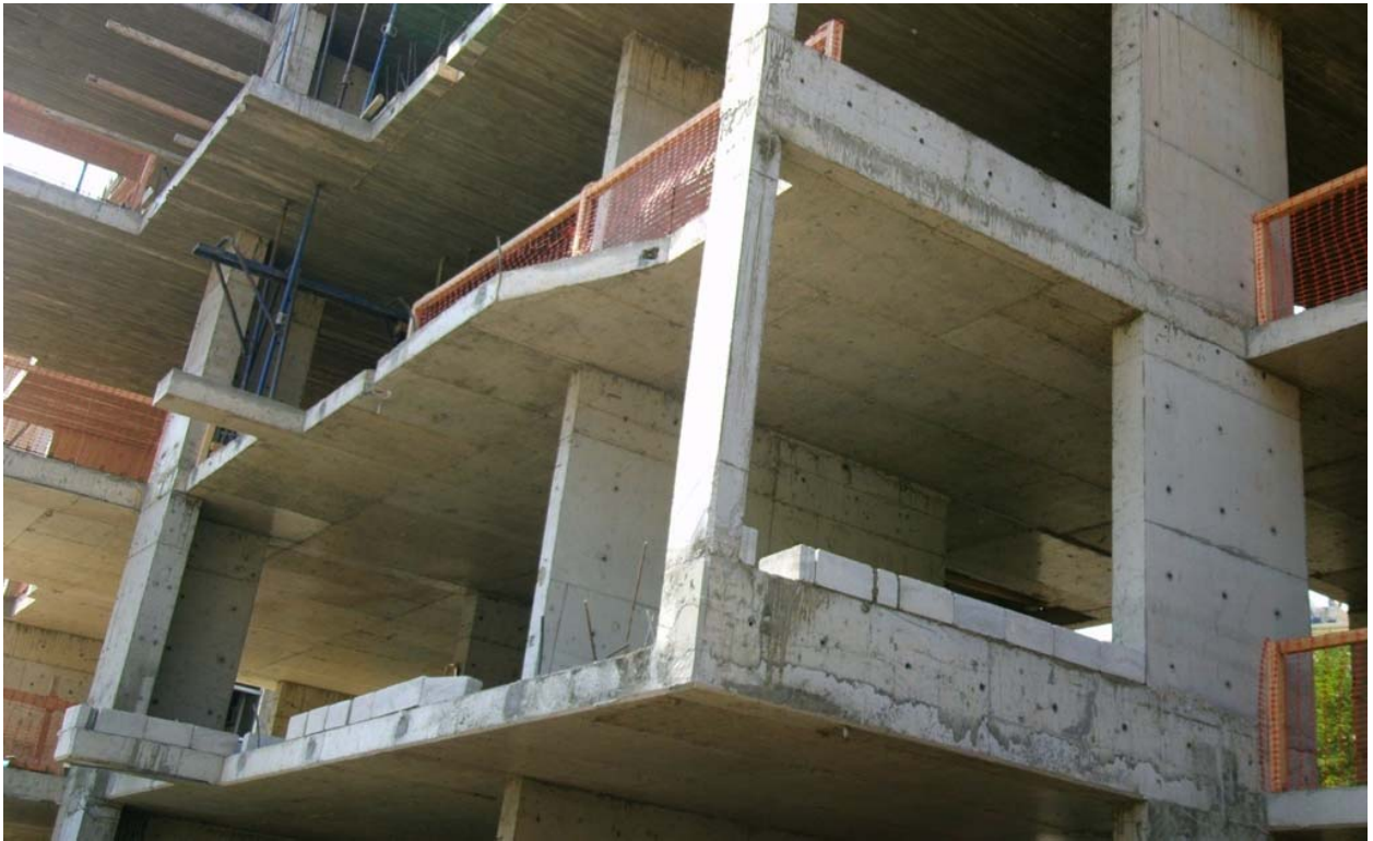
Figure 10: Preparation for blockwork @ 1st floor
