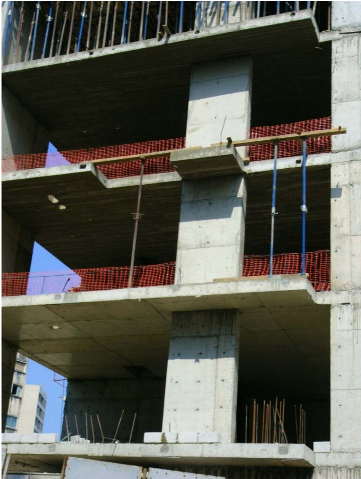
Figure 6: Safety measures being taken on site
