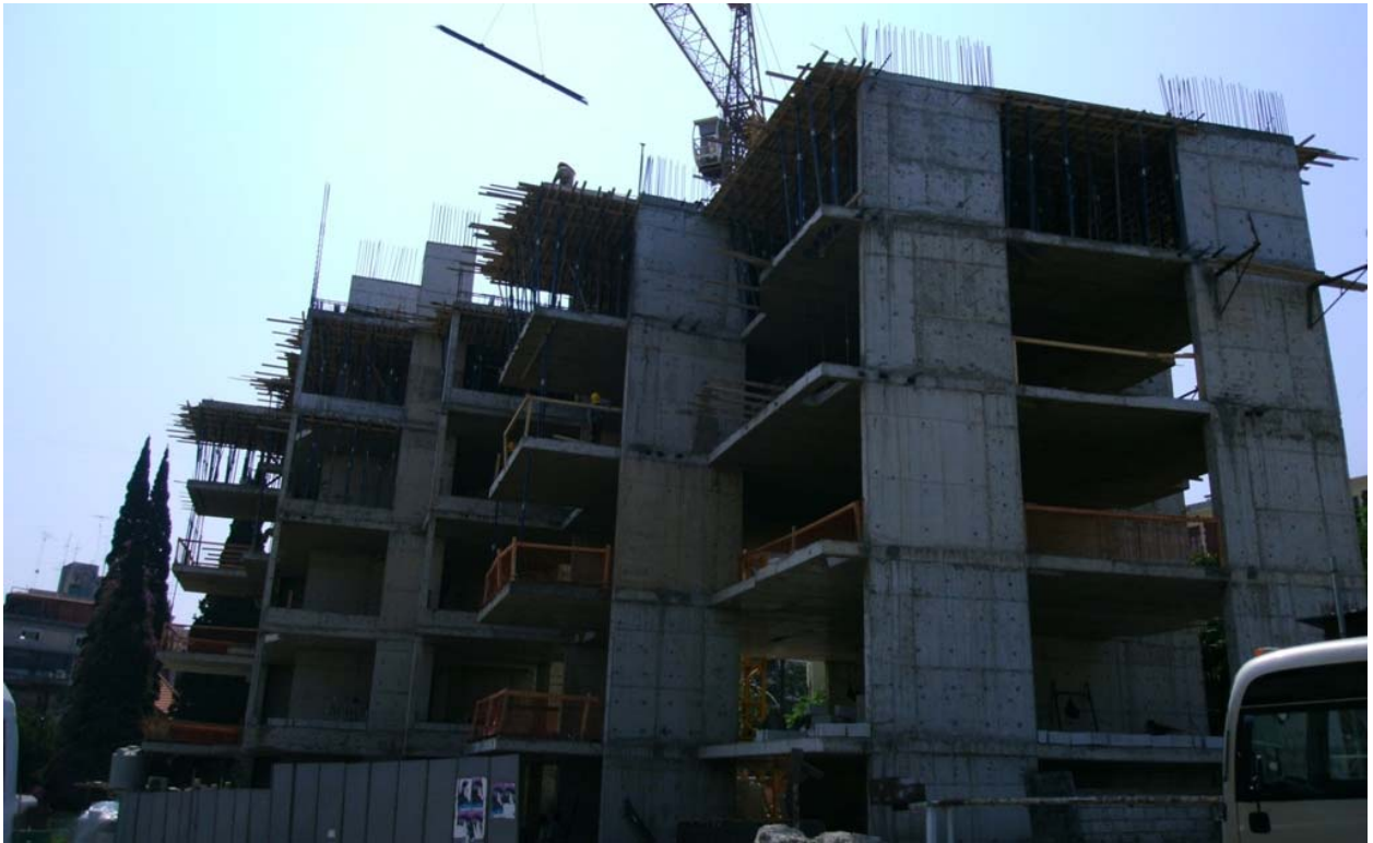
Figure 2: Concrete works / blocks A and B
