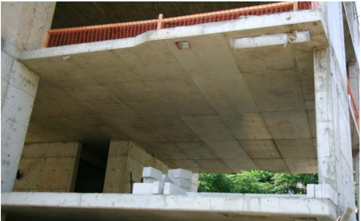
Figure 11: Preparation for blockwork @ 1st floor
