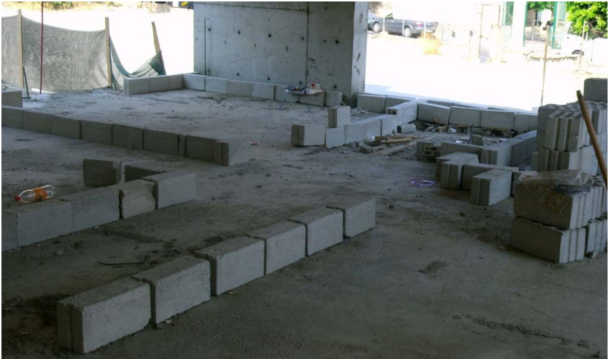
Figure 12: Blockwork start @ 1st floor
