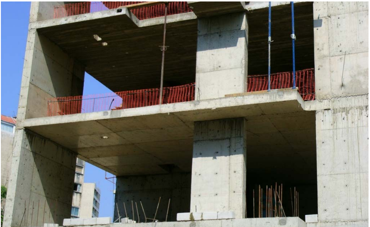
Figure 5: Safety measures being taken on site
