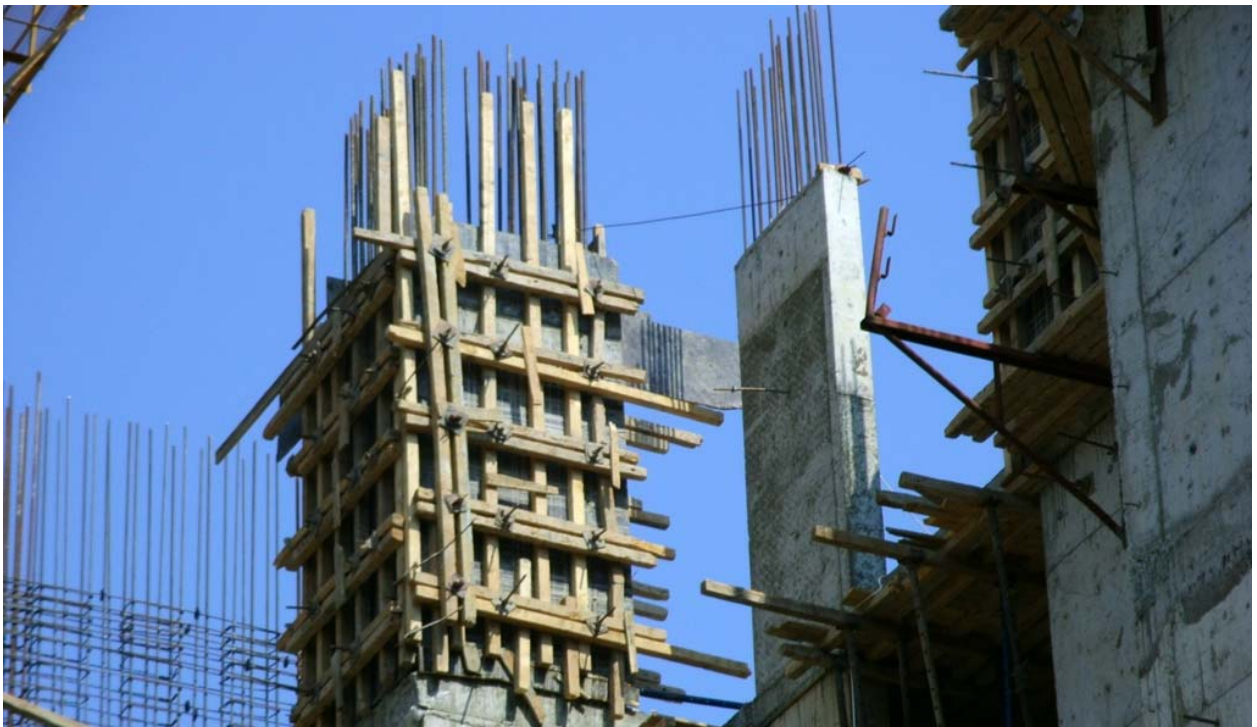
Figure 3: Concrete column casting
