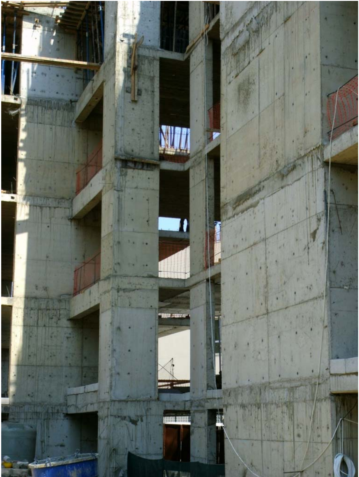
Figure 8: Preparation for blockwork @ 1 st floor
