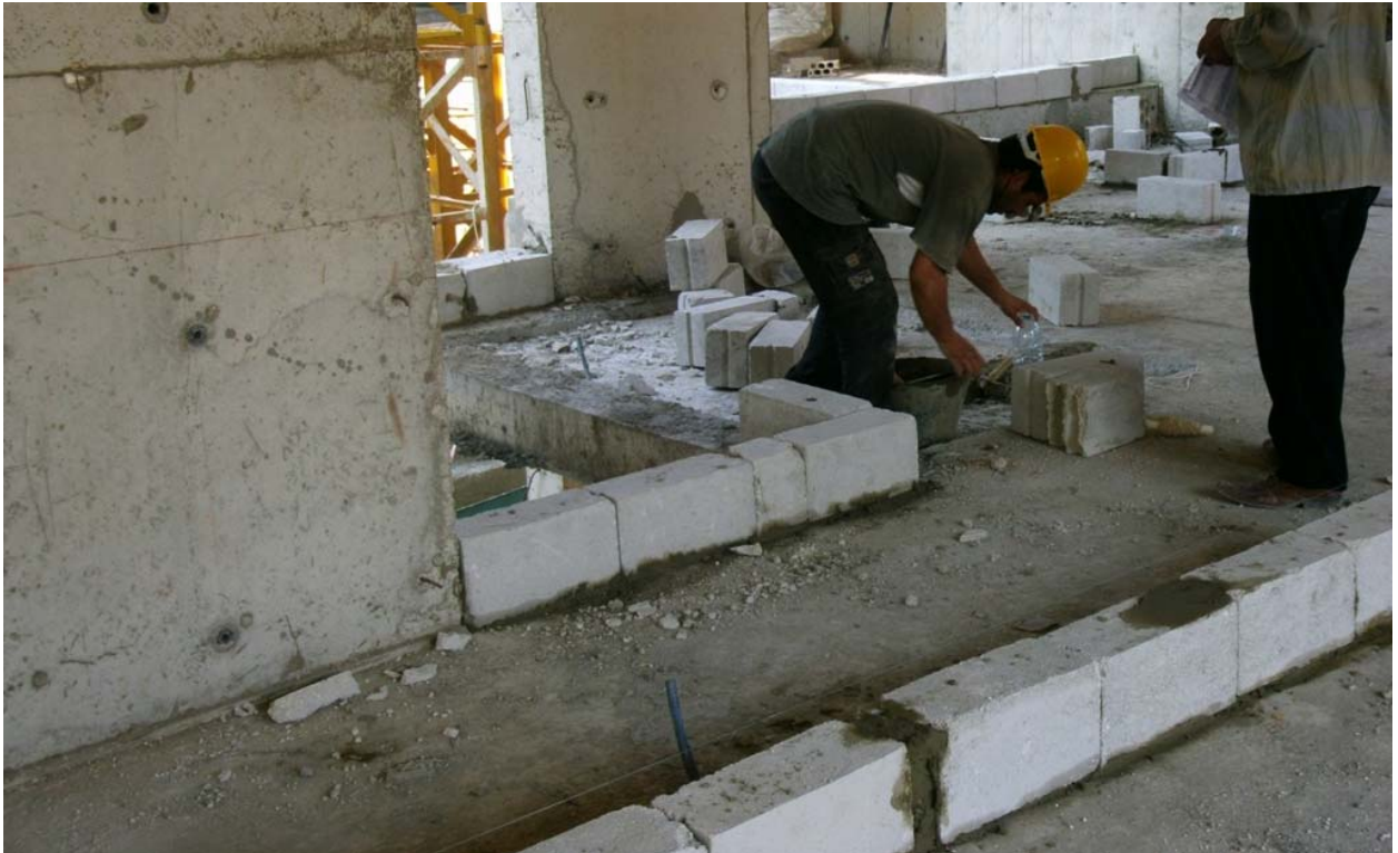
Figure 13: Blockwork start @ 1st floor
