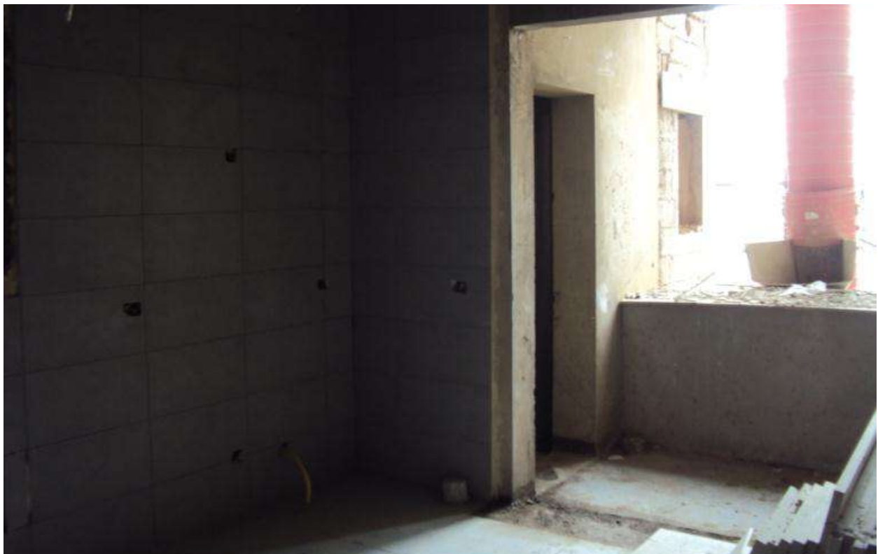
Progress of works in 7 th floor - East & West
