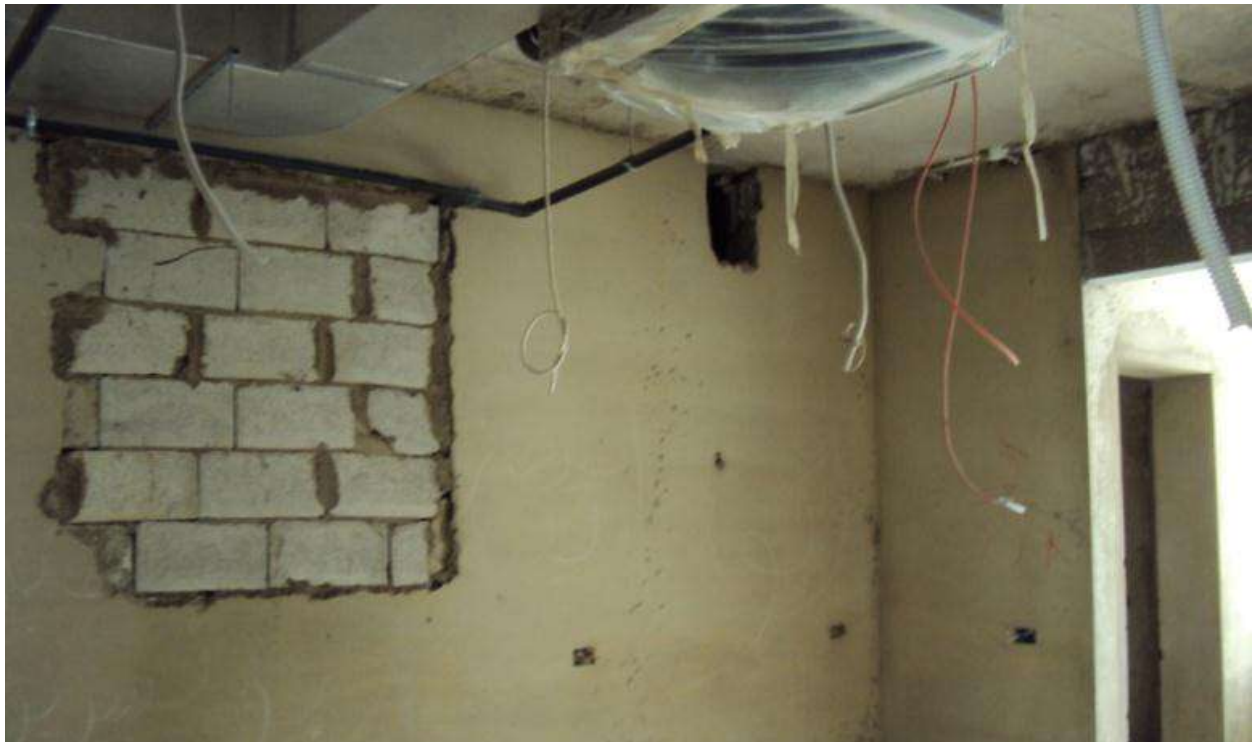
Progress of works in 4 th floor - East & West
