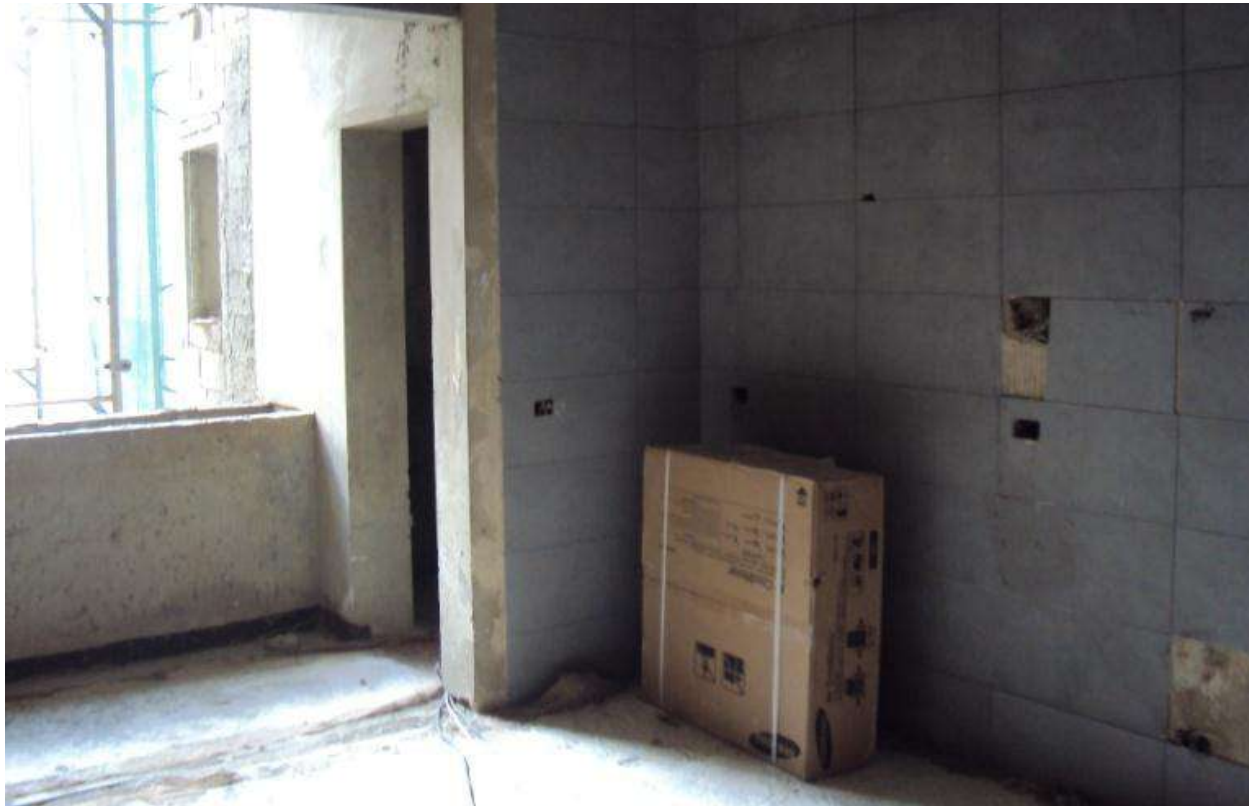
Progress of works in 1 st floor - East & West
