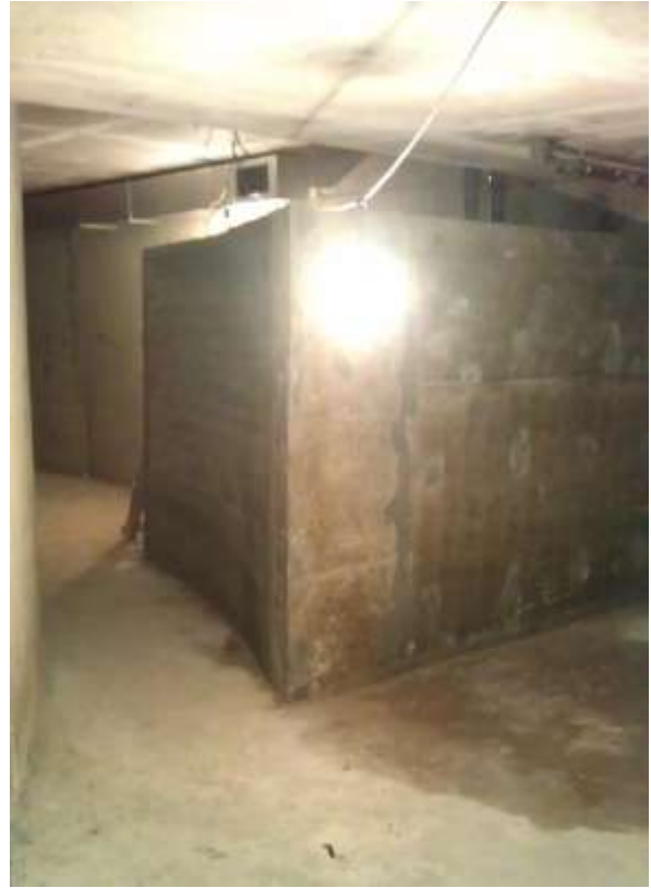
Progress of works in B2
