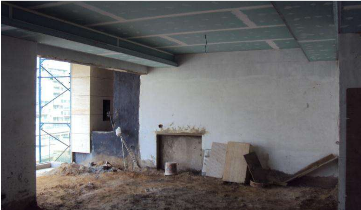
Progress of works in 6 th floor - East & West
