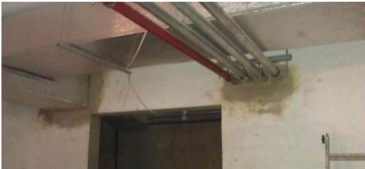
Progress of works in B4
