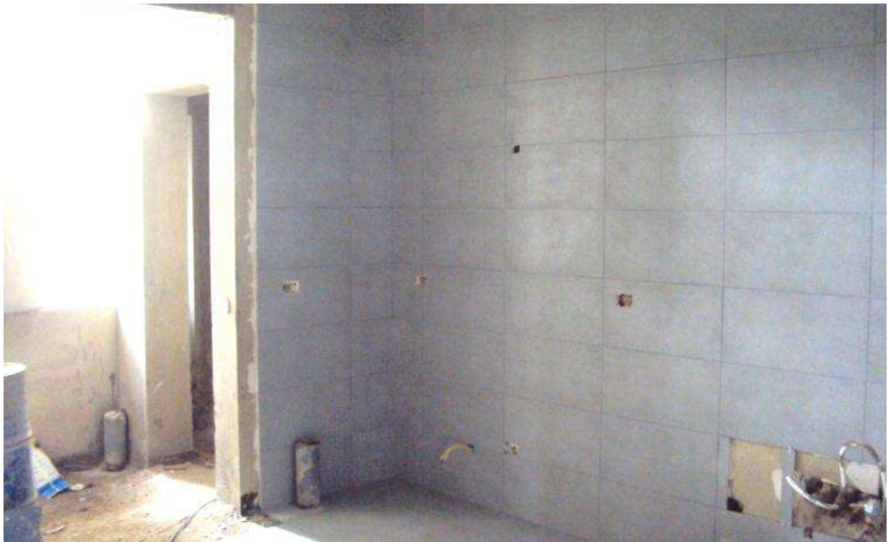
Progress of works in 11 th floor - East & West
