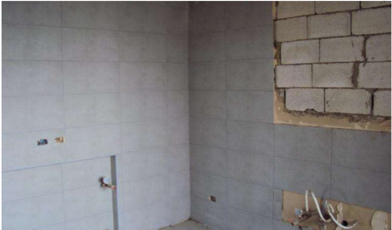
Progress of works in 9 th floor - East & West
