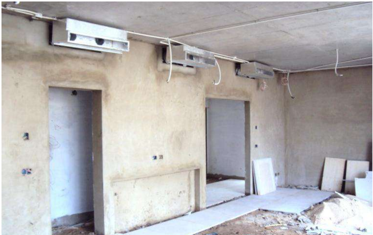
Progress of works in 10 th floor - East & West
