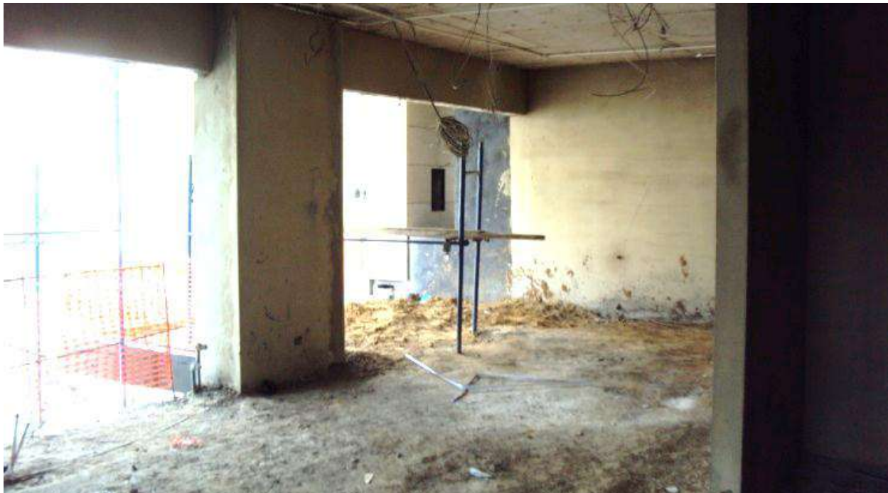
Progress of works in 2 nd floor - East & West
