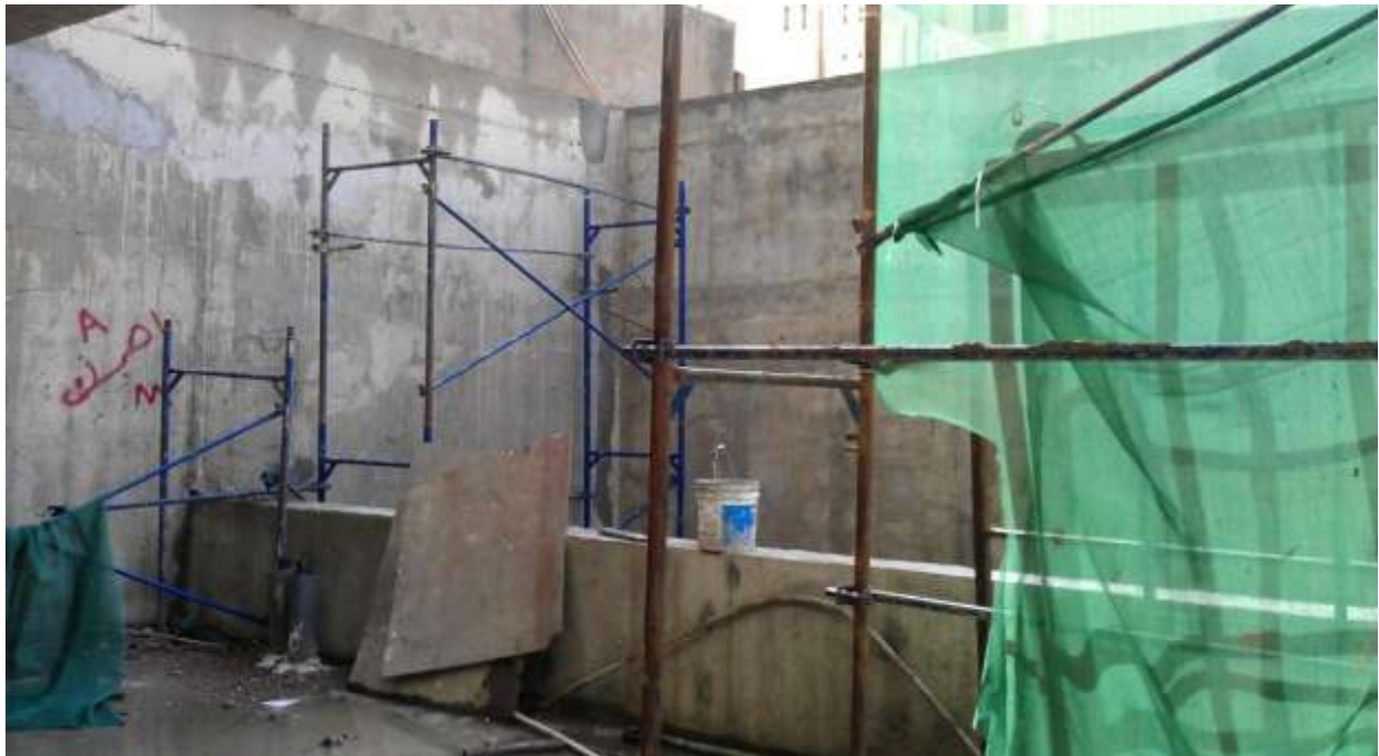
Progress of works in B1
