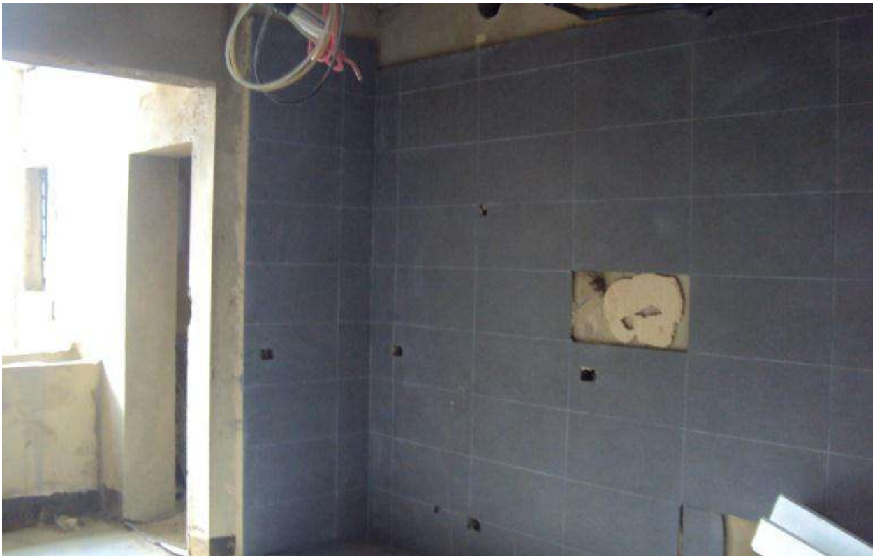
Progress of works in 5 th floor - East & West
