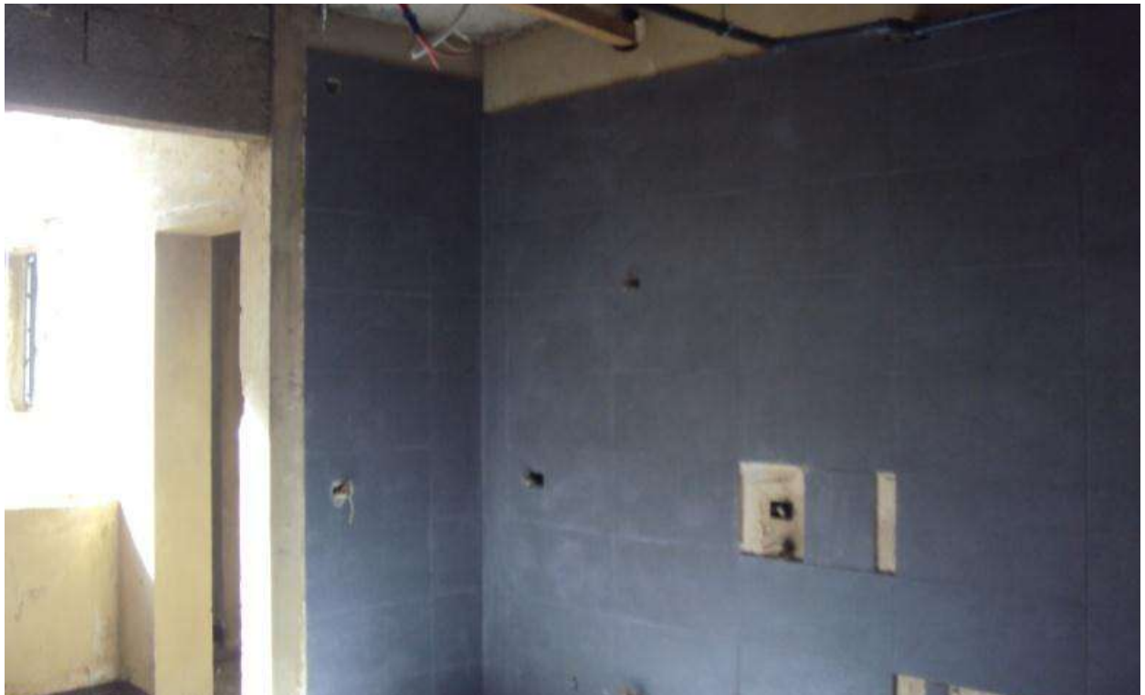
Progress of works in 3 rd floor - East & West
