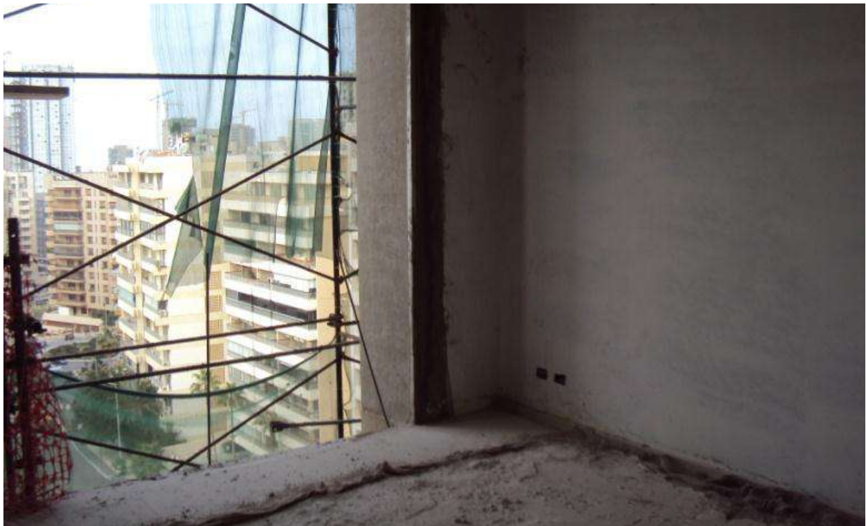
Progress of works in 8 th floor - East & West
