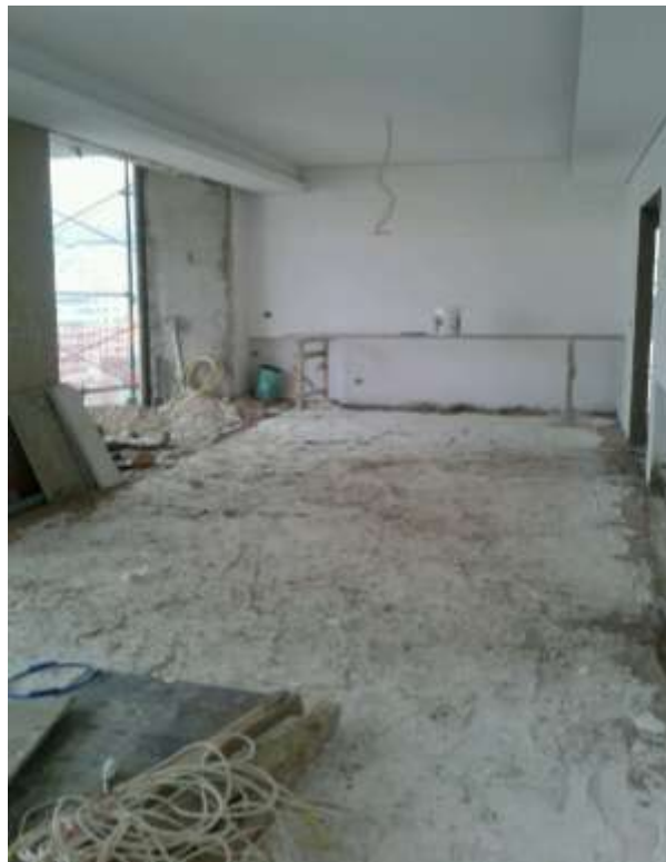
Progress of works in 11 th floor
