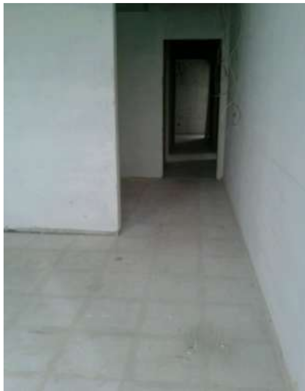
Progress of works in 9 th floor
