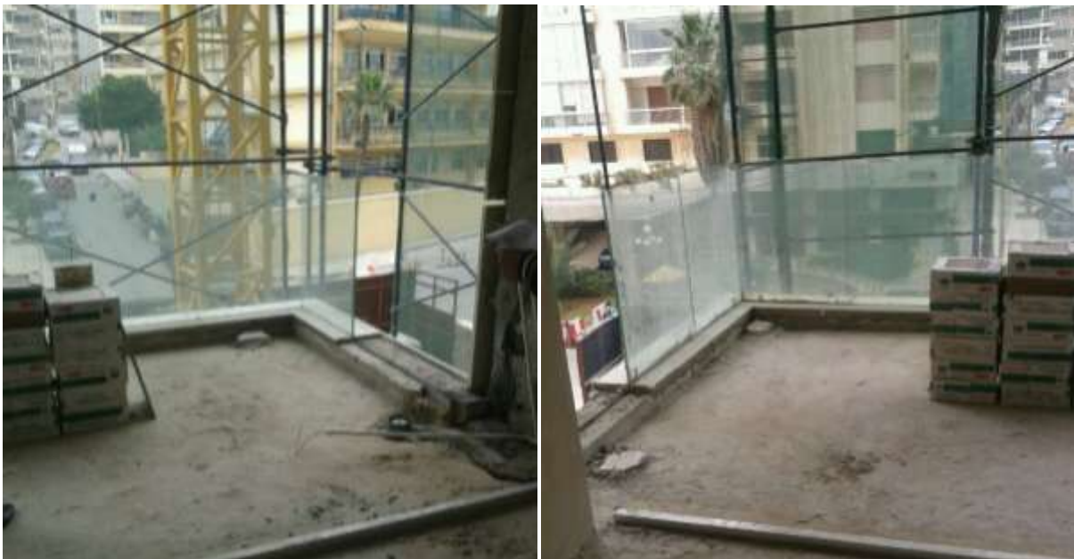
Progress of works in 1 st floor
