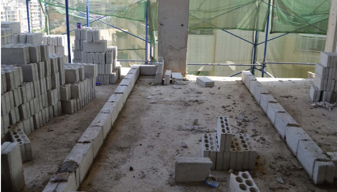
Figure 19: Blockwork start on 12th floor
