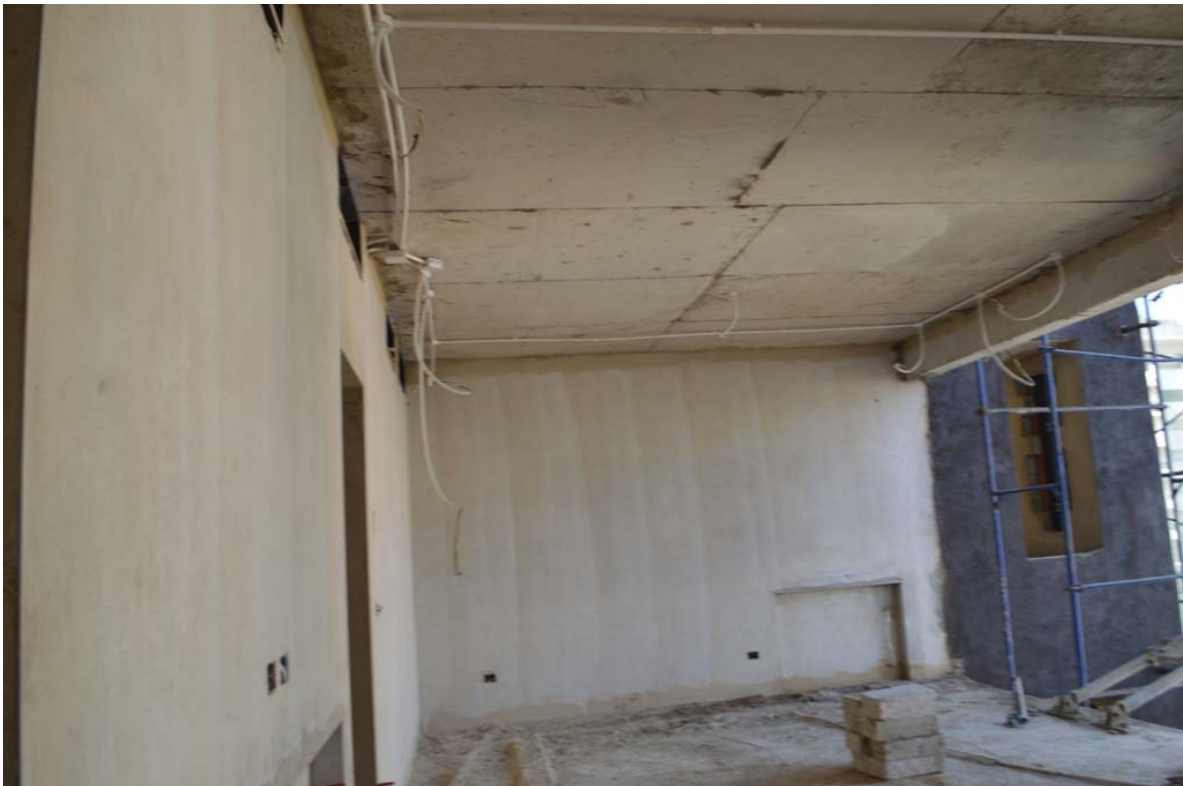
Figure 26: 1st paint coats being applied
