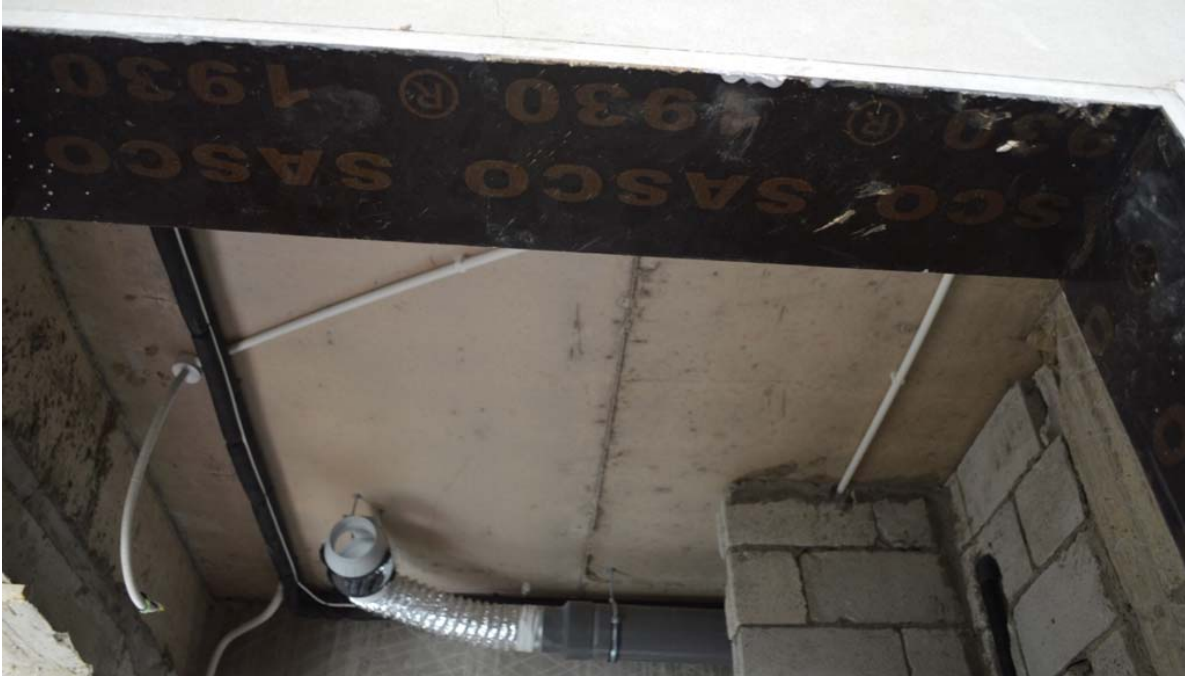
Figure 25: Wood subframes on 8th floor
