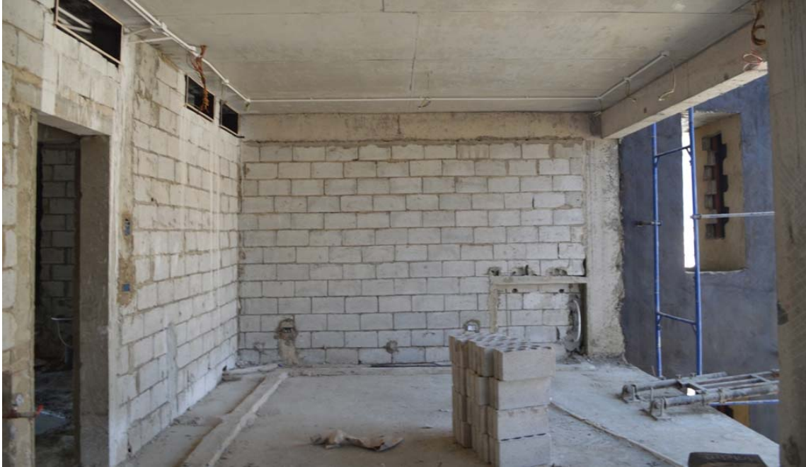
Figure 23: Blockwork on 10th floor
