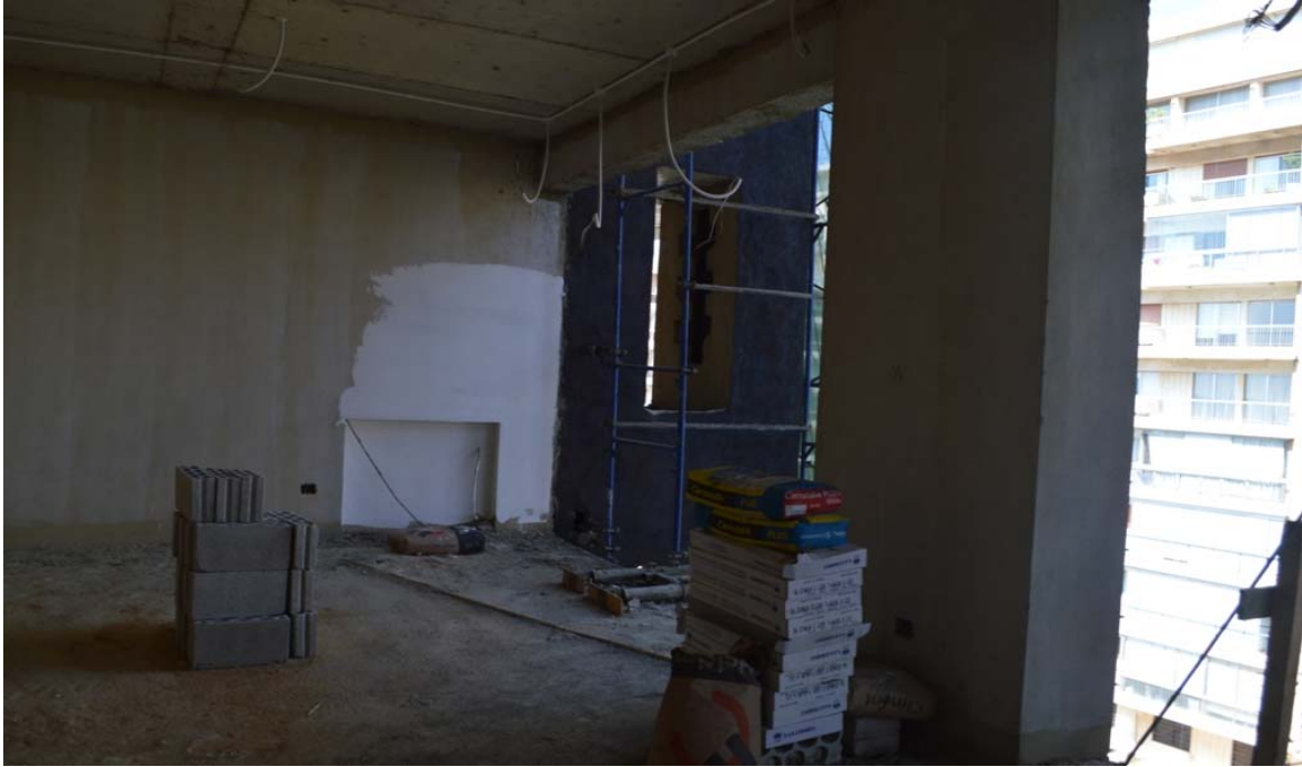
Figure 27: Tiling works ready to start @ upper floors
