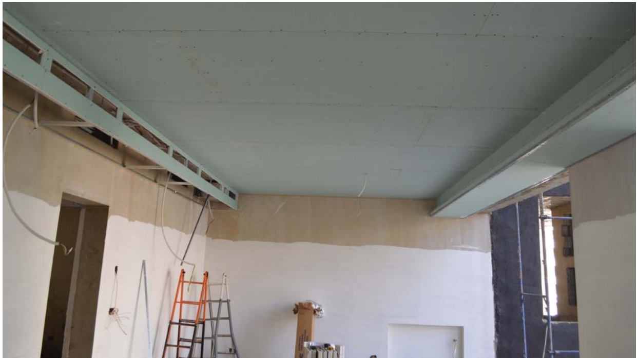
Figure 28: False ceiling works being finalized on 1st floor
