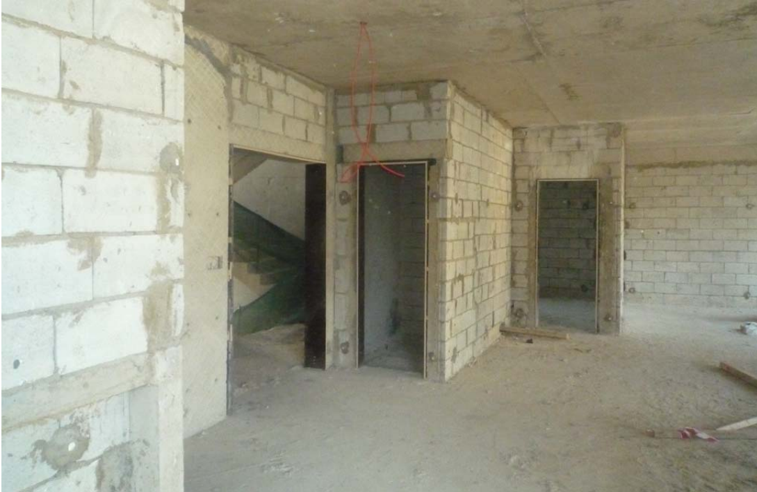
Figure 43: Blockwork @ 4th floor (east)
