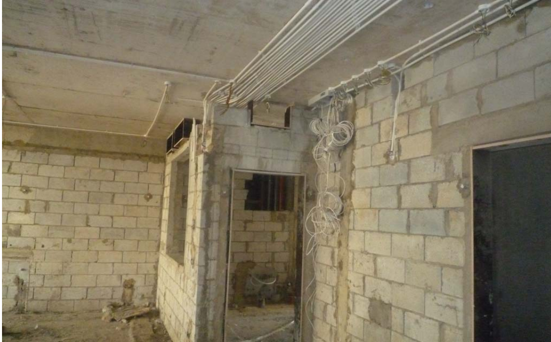
Figure 47: Blockwork @ 1st floor (west)
