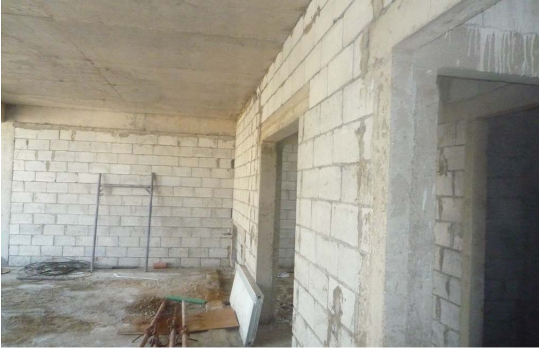
Figure 23: Blockwork @ 11th floor
