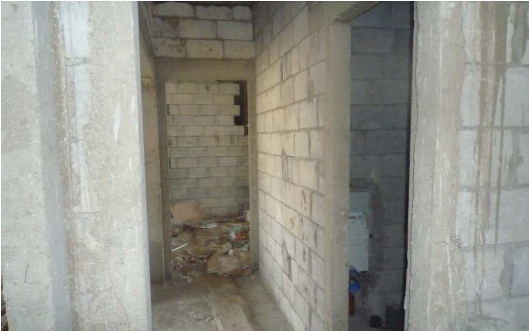
Figure 24: Blockwork @ 10th floor
