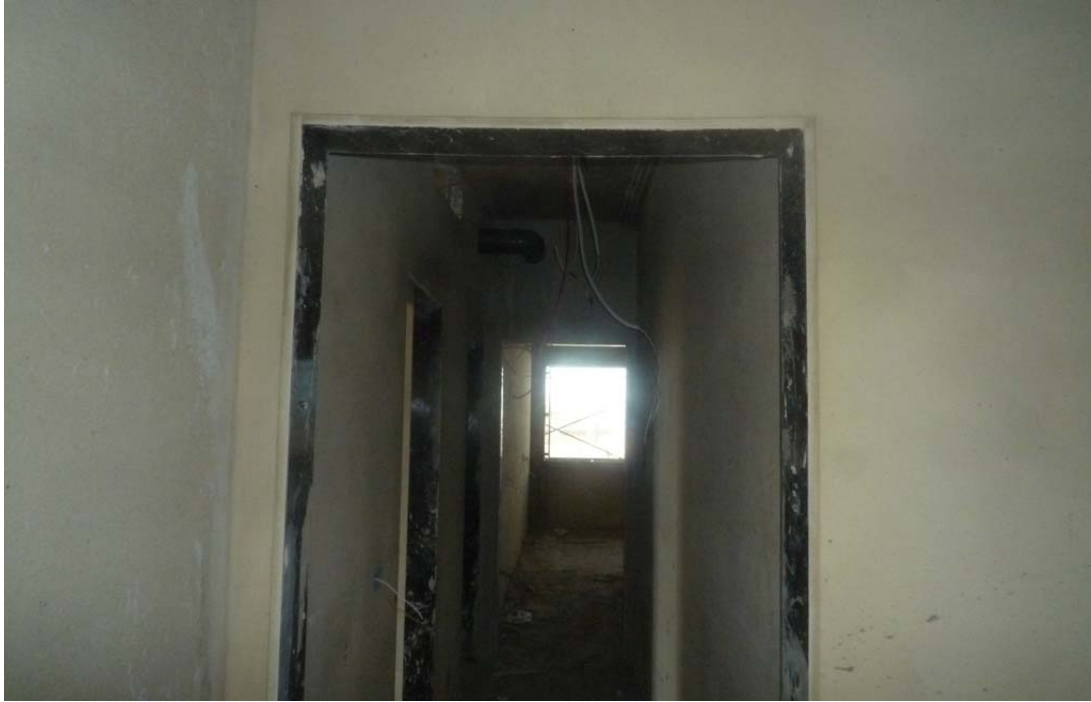
Figure 39: Wood subframes installation @ 7th floor
