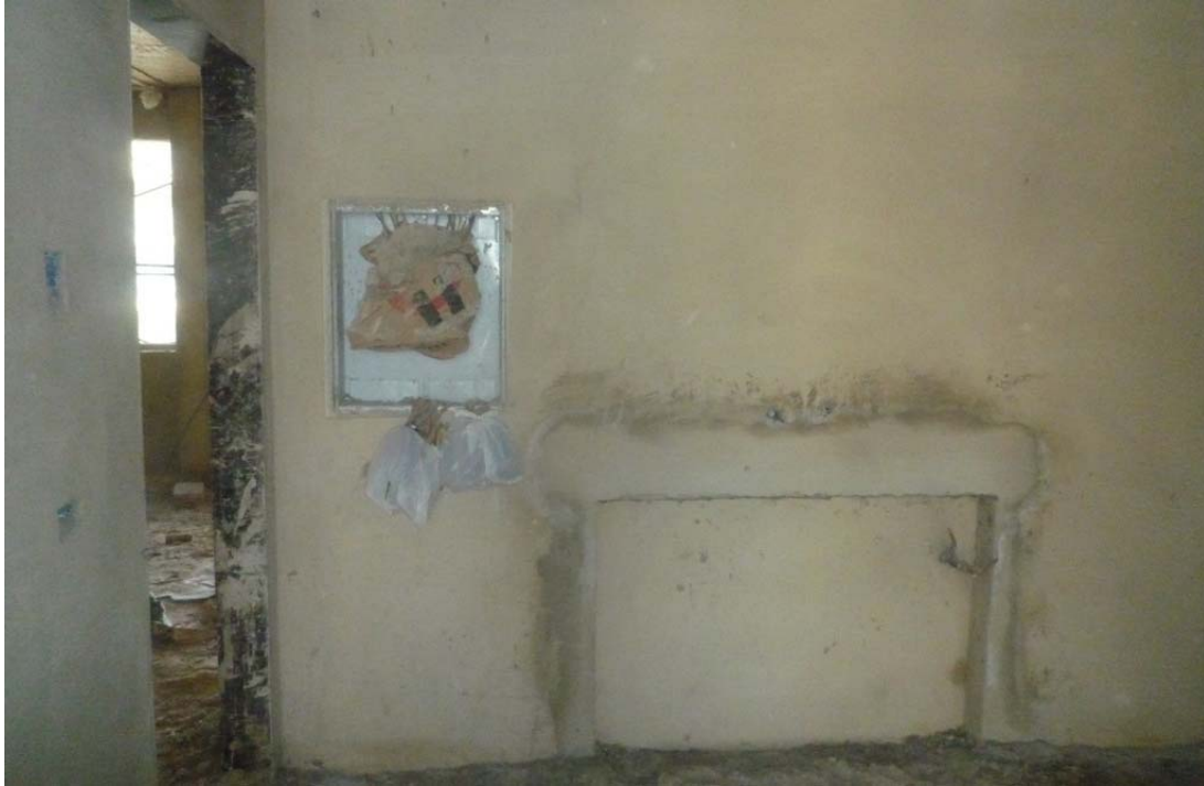
Figure 37: Panel board installation @ 7th floor
