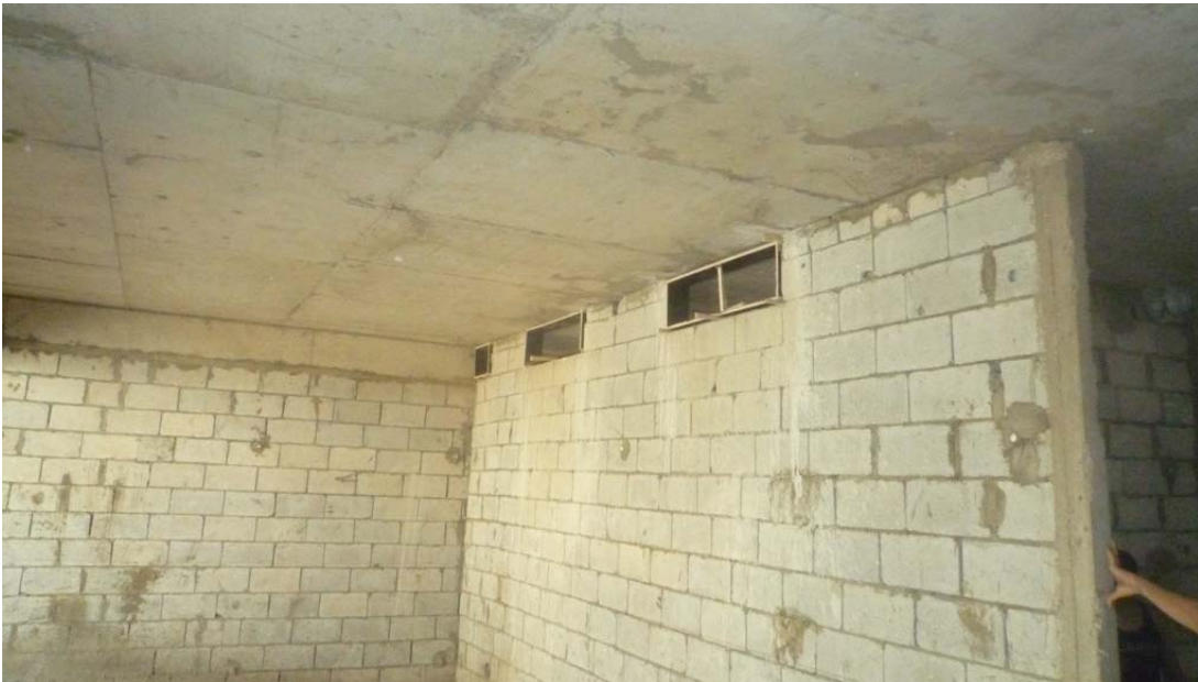
Figure 46: Blockwork @ 2nd floor (west)
