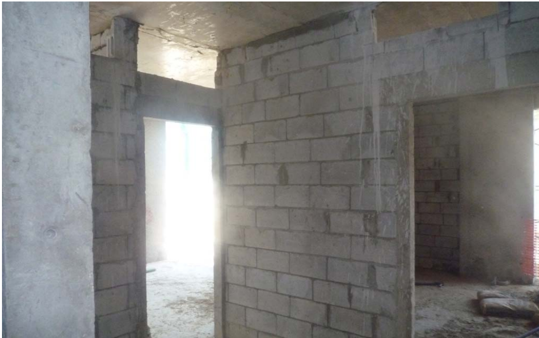
Figure 22: Blockwork @ 11th floor
