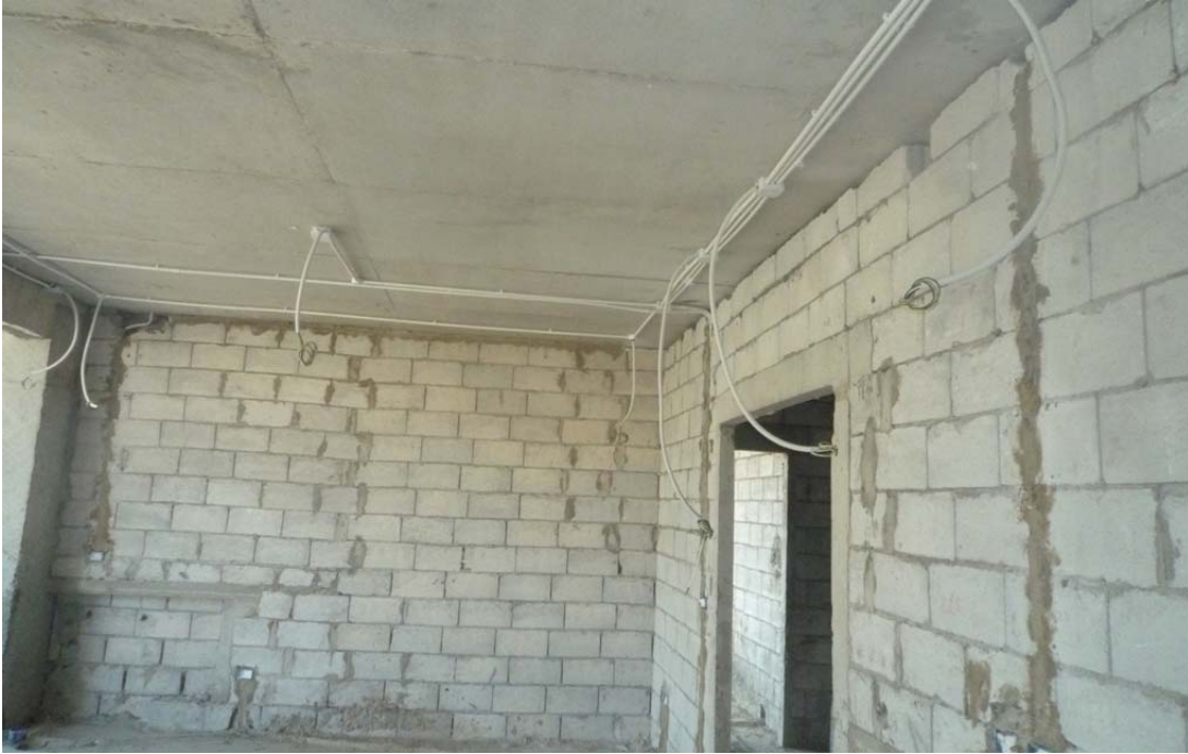
Figure 25: Blockwork @ 10th floor
