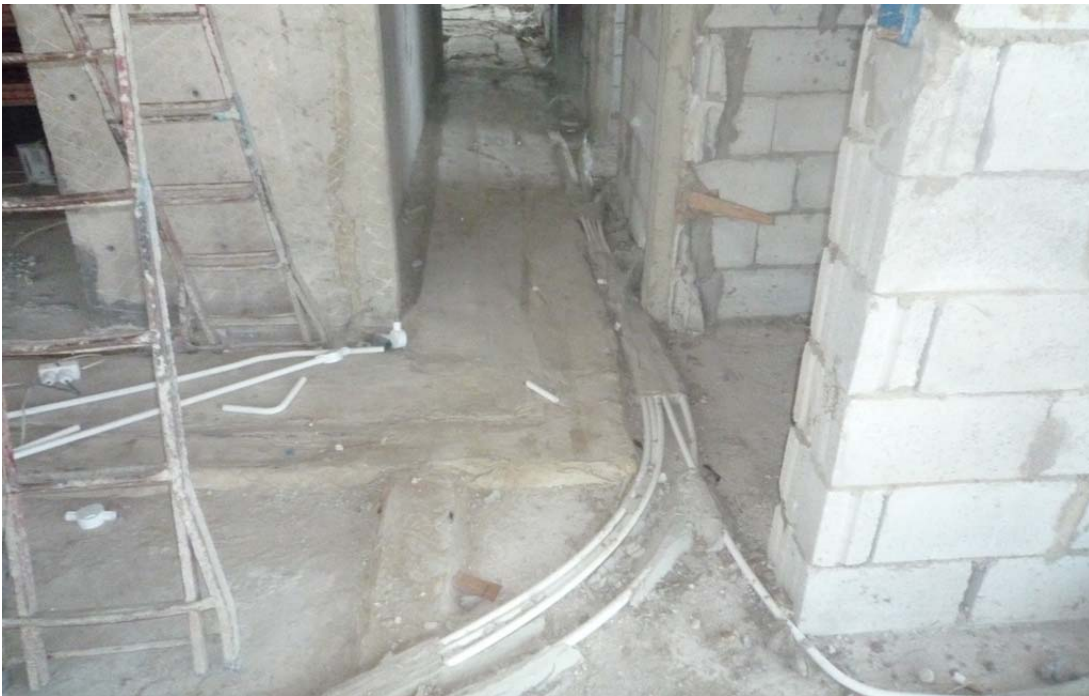
Figure 30: Blockwork @ 9th floor
