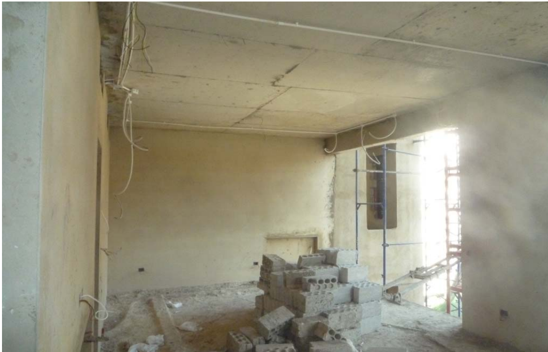
Figure 38: Plaster works @ 7th floor
