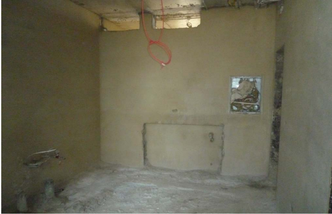
Figure 33: Plastering works @ 8th floor
