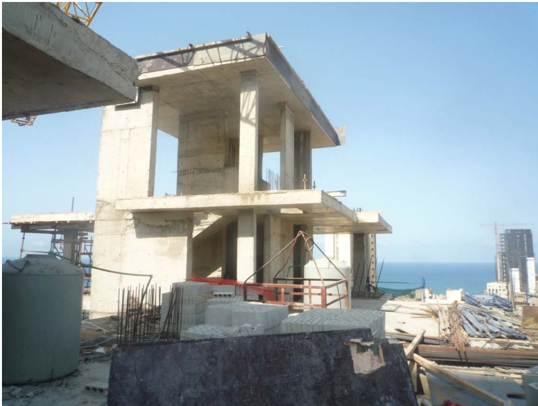
Figure 16: Concrete works complete - View from the 13th floor
