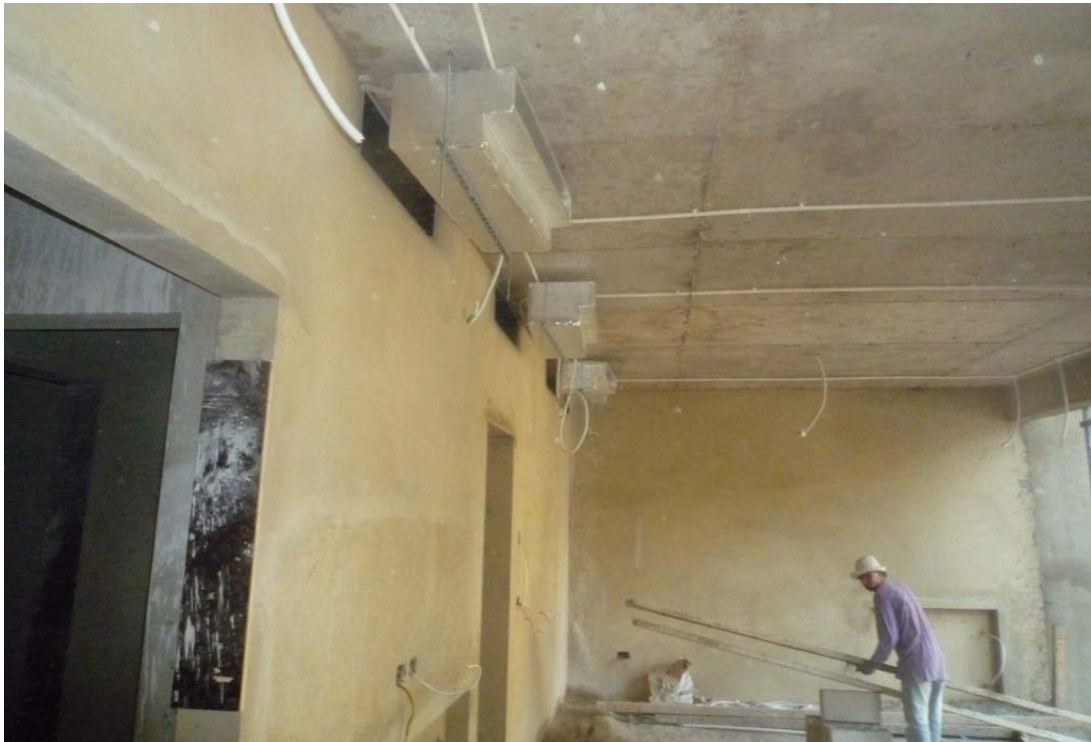
Figure 48: Plaster works and VAC installations @ 1st floor (east)
