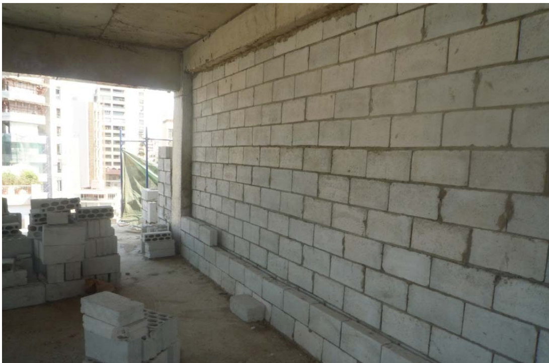
Figure 20: Blockwork @ 11th floor
