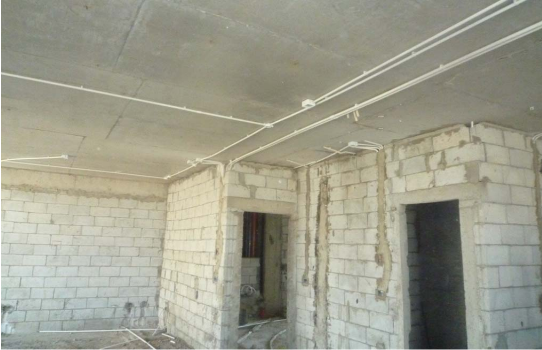
Figure 29: Blockwork @ 9th floor
