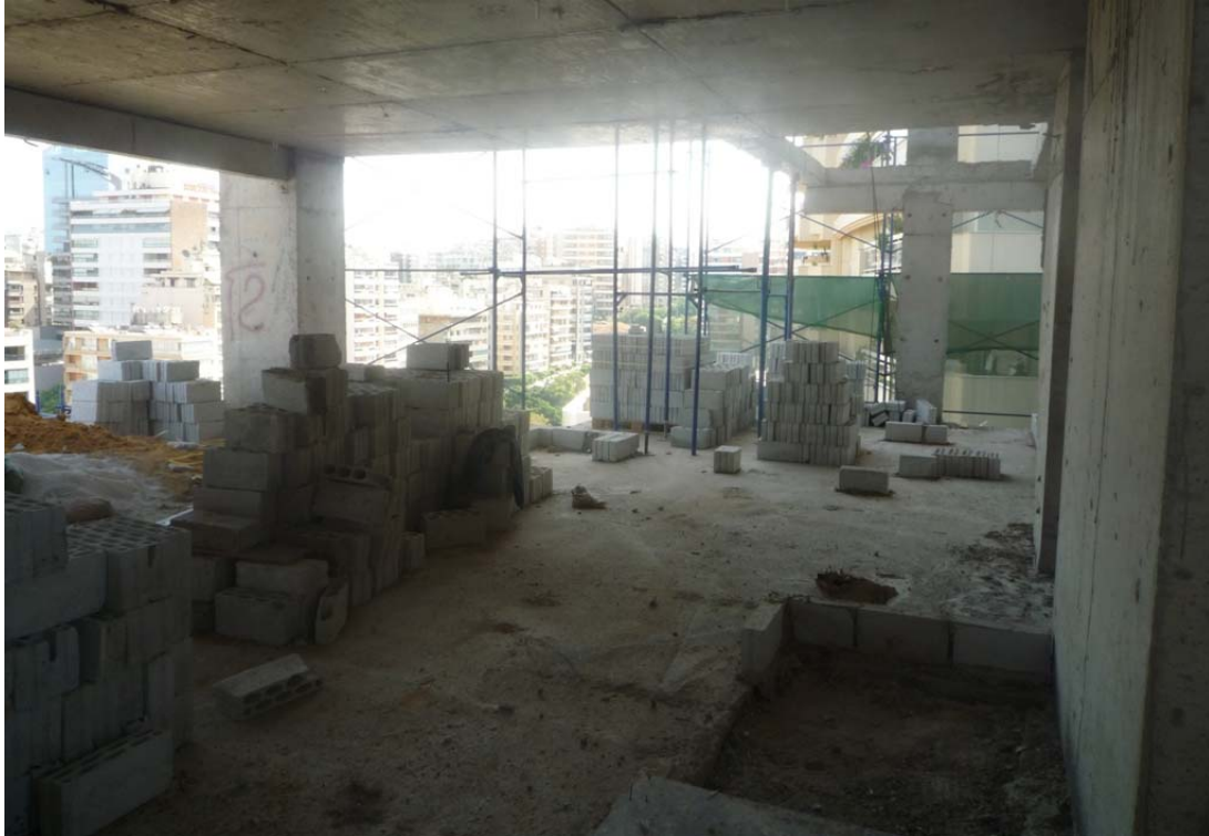
Figure 19: Blockwork initiation @ 12th floor
