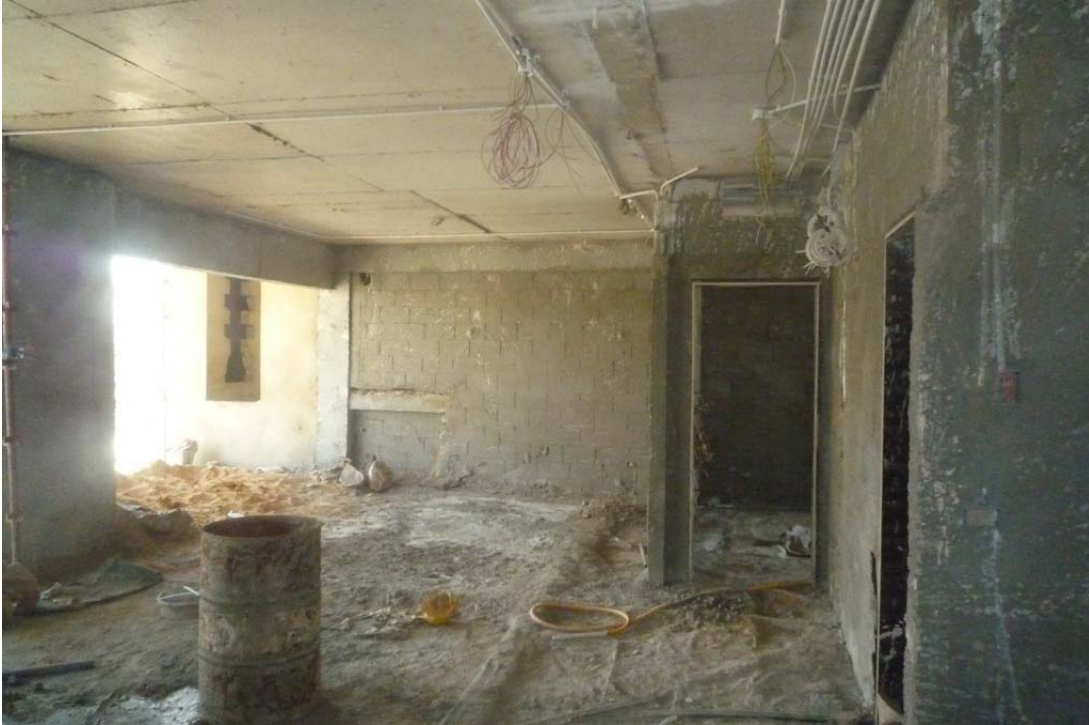
Figure 35: Blockwork @ 8th floor (recent modifications)
