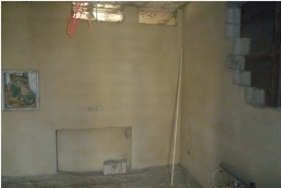
Figure 40: Plaster works @ 6th floor
