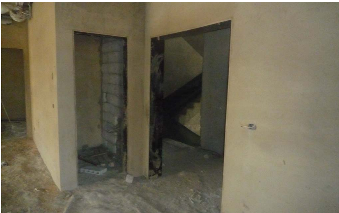
Figure 42: Plaster works @ 6th floor
