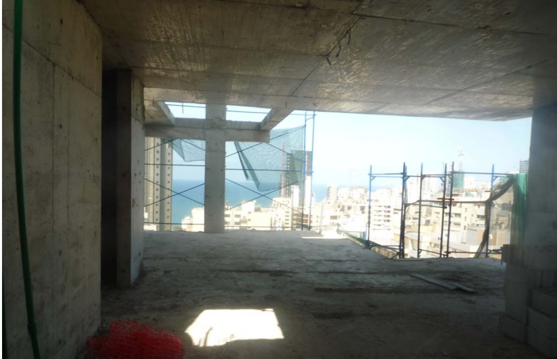
Figure 21: Concrete works @ 12th floor
