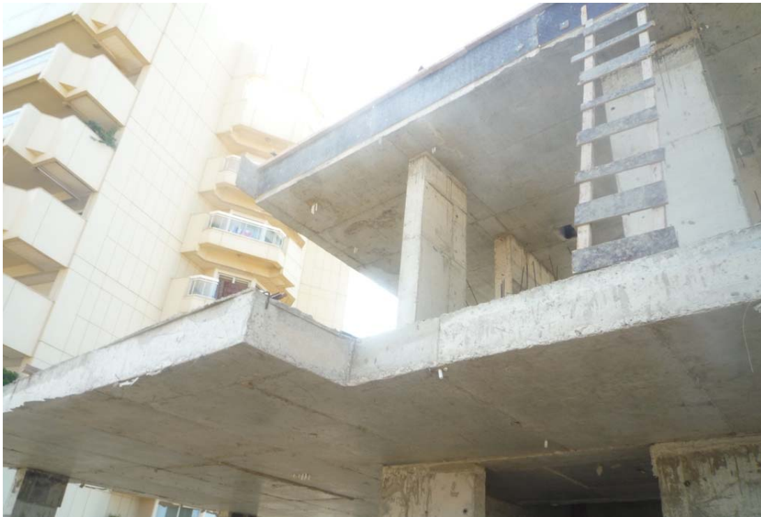
Figure 18: Concrete works complete @ 12th floor
