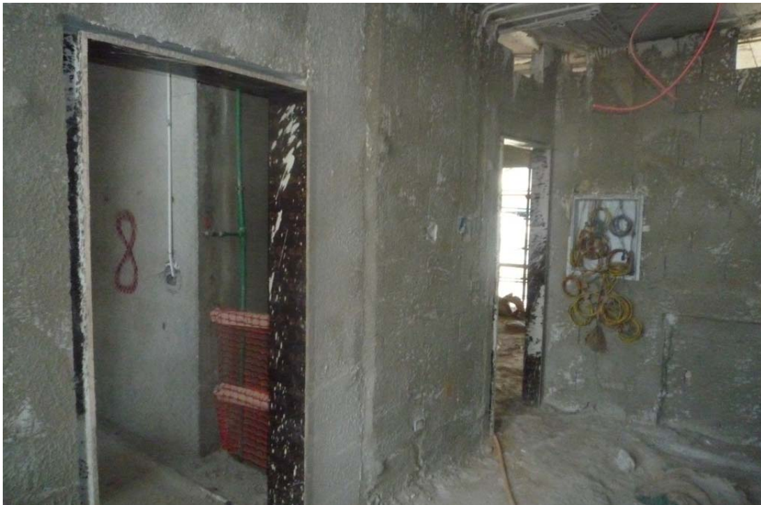
Figure 34: Wood subframes installation @ 8th floor
