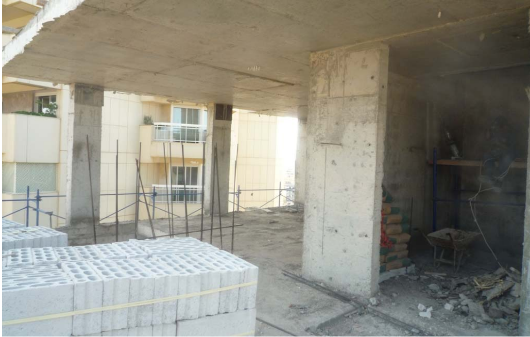
Figure 17: Blockwork initiation @ 12th floor
