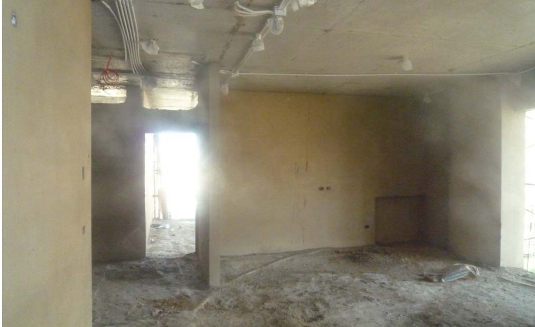
Figure 41: Plastering works @ 6th floor
