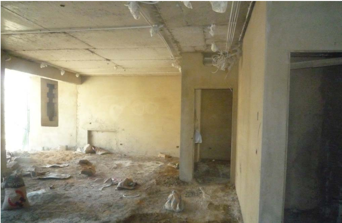
Figure 36: Blockwork @ 7th floor
