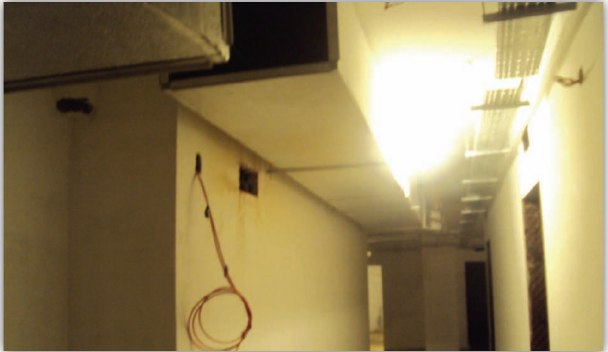
Figure 17: Ducting works in basements - June 2012
