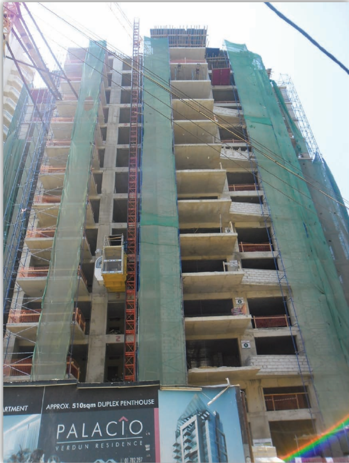
Figure 16: Main elevation - June 2012
