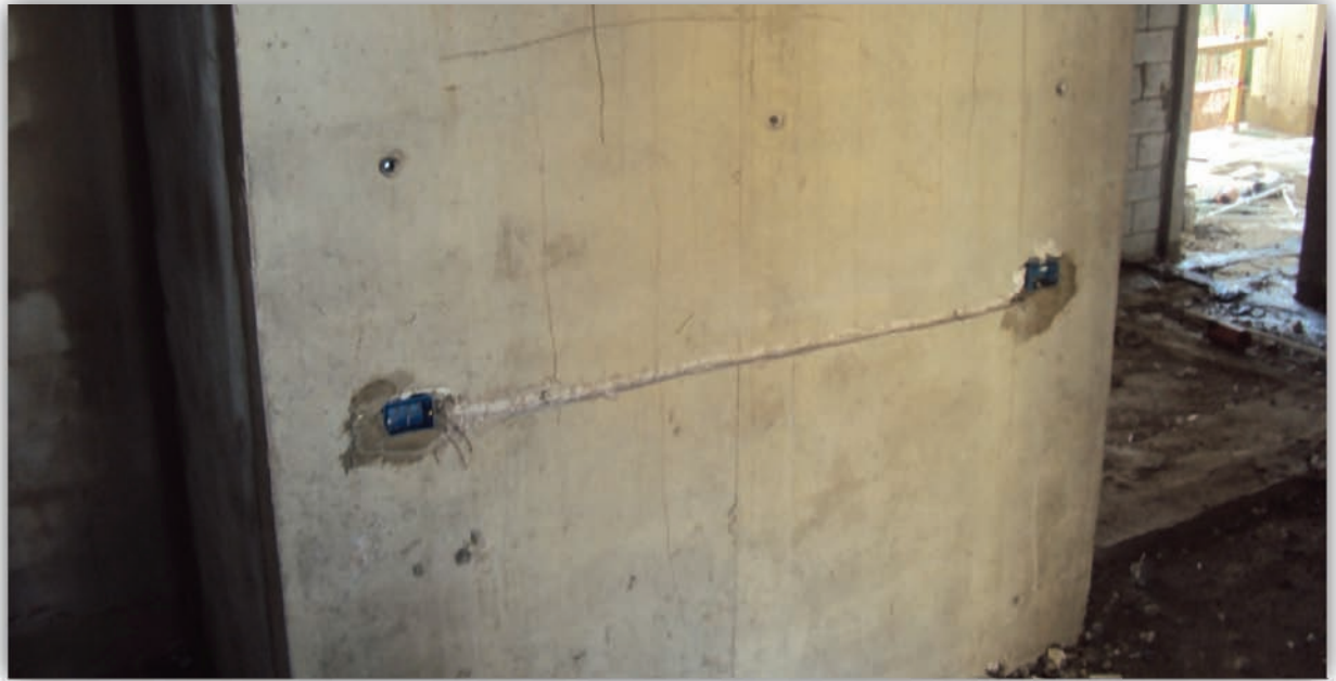
Figure 29: Electrical works in 7th floor - June 2012
