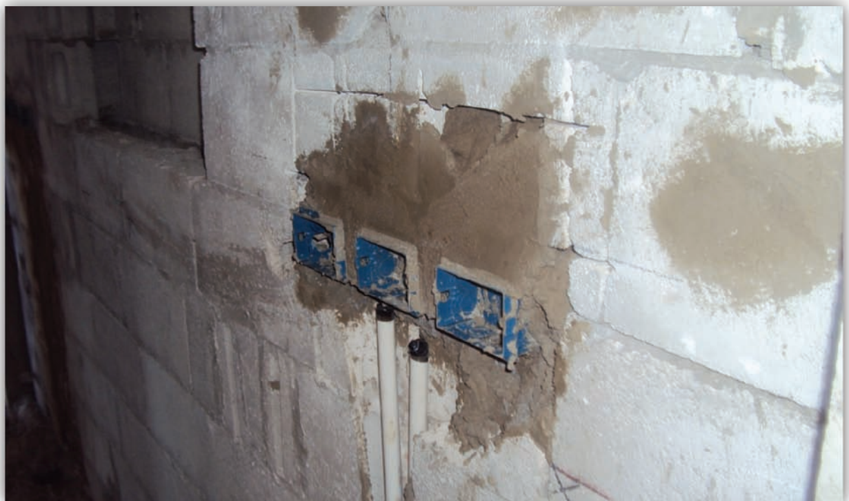
Figure 30: Electrical works in 7th floor - June 2012
