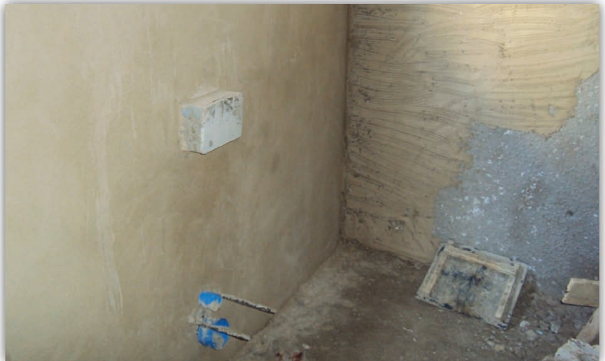
Figure 34: Plastering works complete in 3rd floor - June 2012
