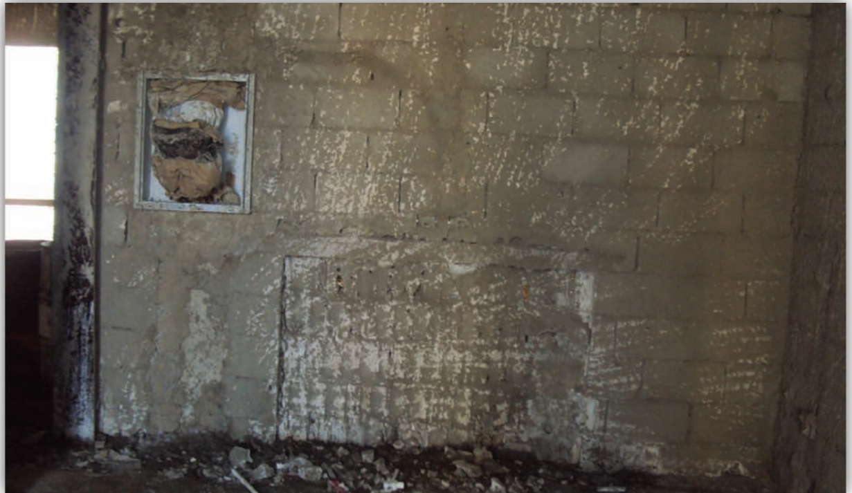
Figure 31: Preparation for plastering in 6th floor - June 2012
