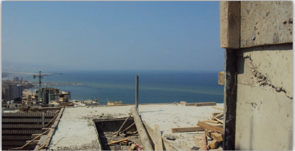
Figure 23: Concrete works on 12th floor - June 2012
