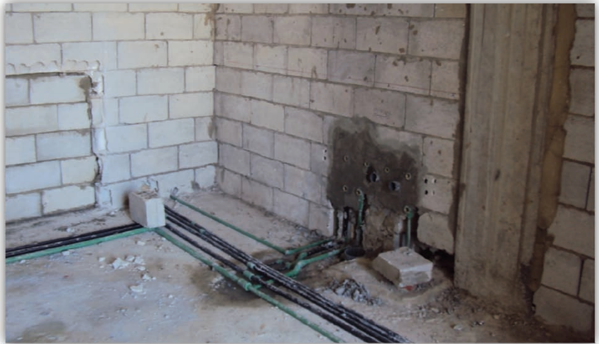
Figure 27: Plumbing installations in 9th floor - June 2012
