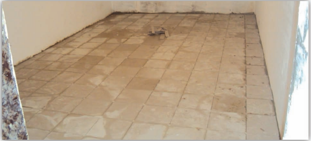
Figure 19: Tiling and paint works in basements - June 2012
