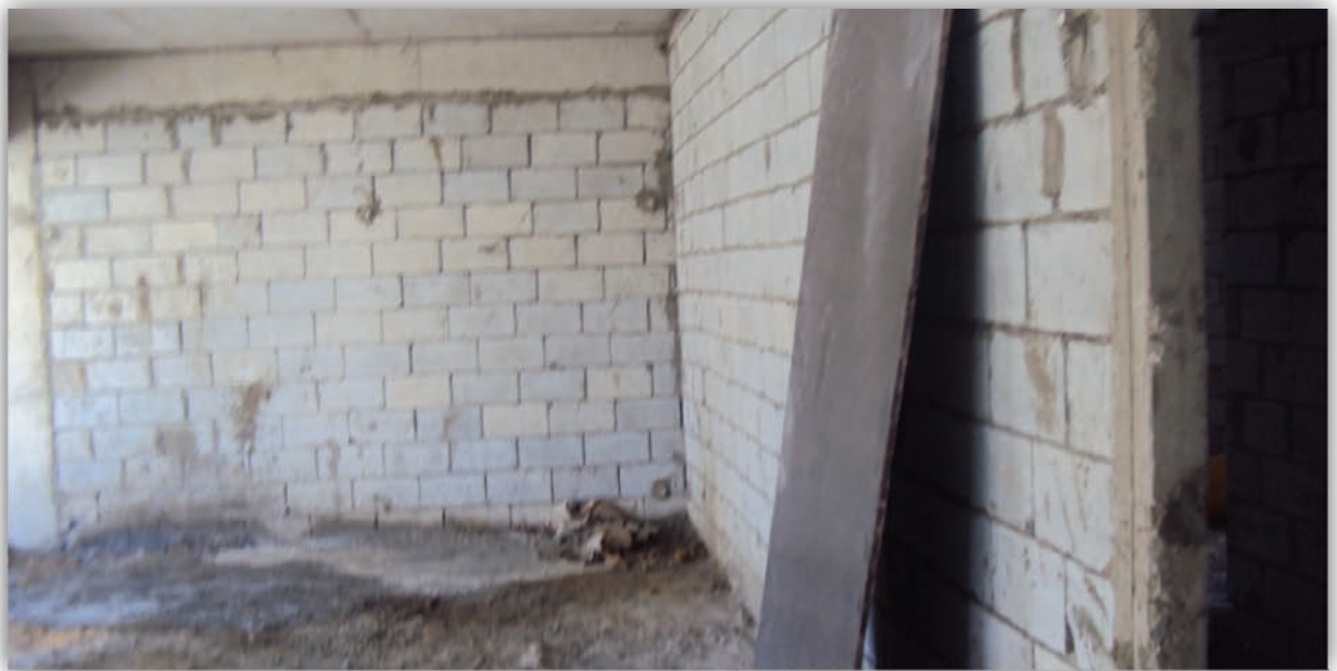
Figure 26: Blockwork on 10th floor - June 2012
