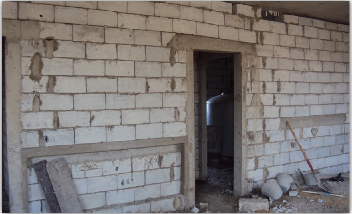
Figure 25: Blockwork on 11th floor - June 2012
