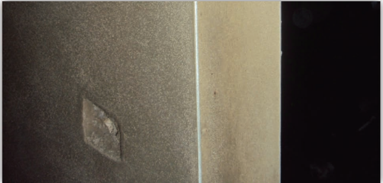
Figure 33: Plastering works complete in 3rd floor - June 2012
