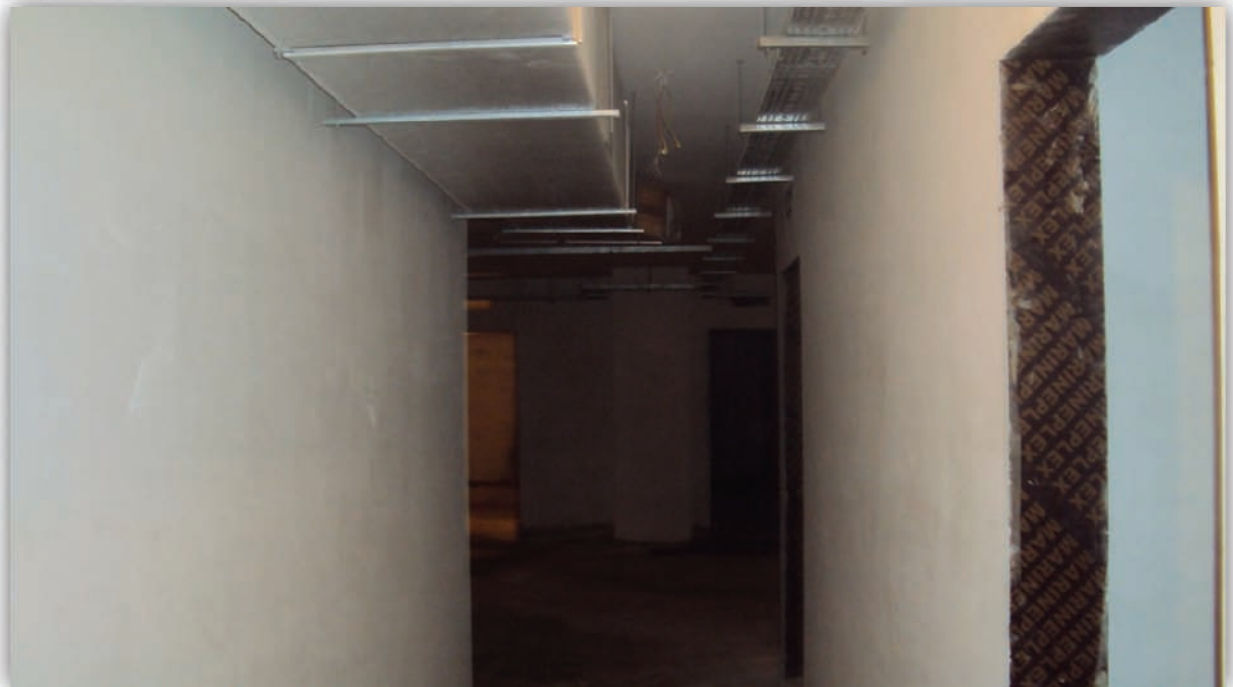
Figure 18: Ducting works in basements - June 2012
