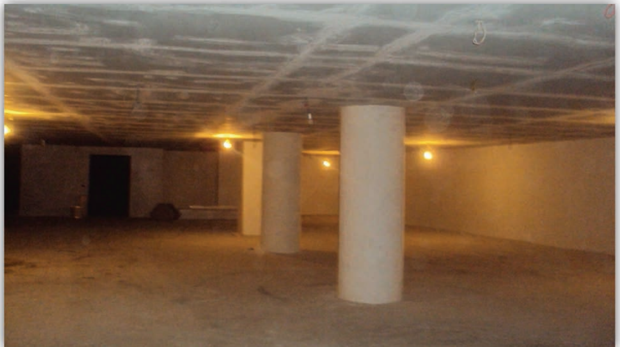
Figure 20: Ceilings and walls repair in basements - June 2012
