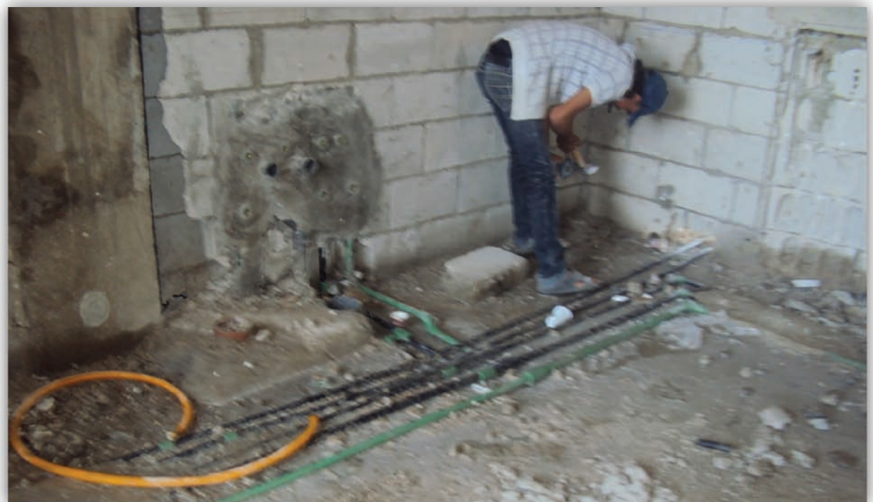
Figure 28: Plumbing installations in 8th floor - June 2012
