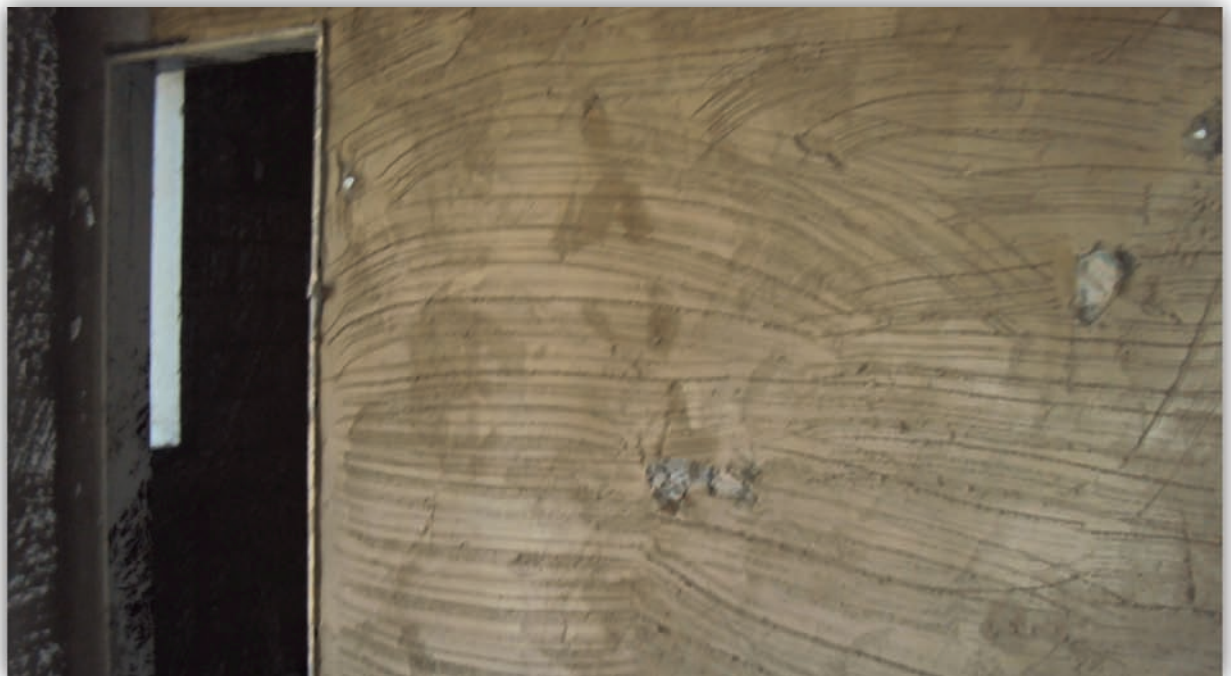
Figure 32: Wood subframes installed, walls prepared for plastering in 5th floor - June 2012
