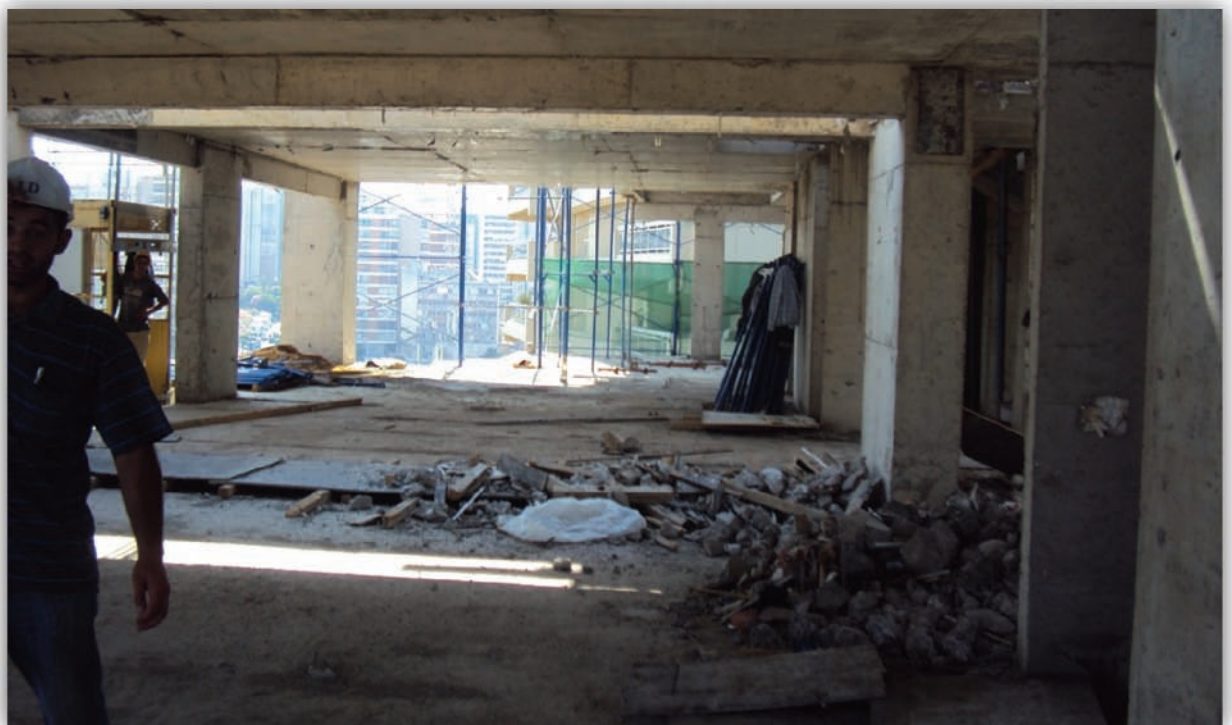
Figure 24: Concrete works on 12th floor - June 2012
