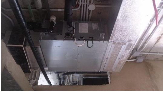
- Fan coil unit fixation at 6 th floor .
