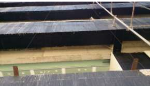
- Verticals level line for aluminum cladding.
