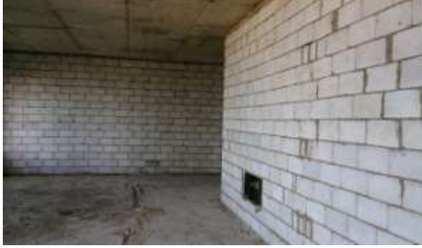
- Blockwork at 13 th floor.
