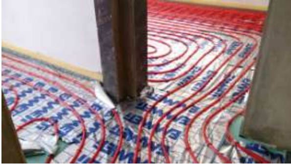
- Floor heating in 2 nd floor.
