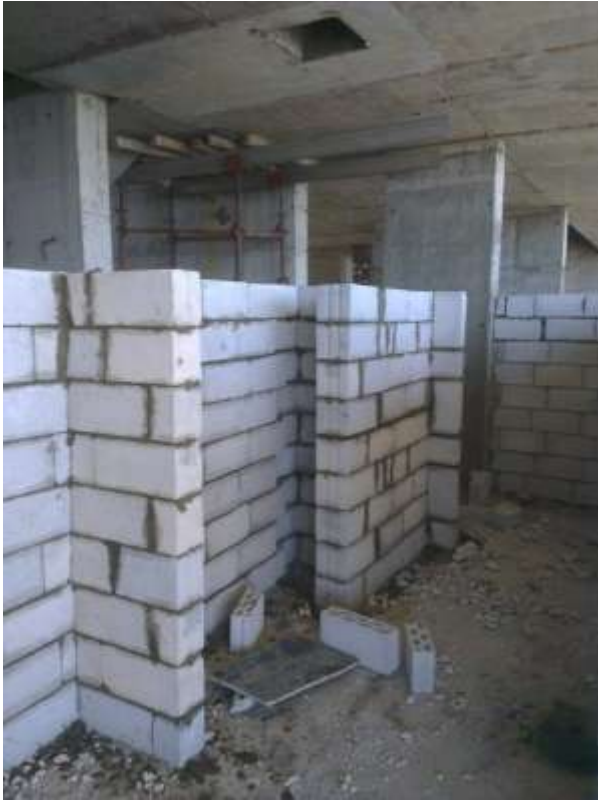
- Blockwork in 16 th and attic floors.
