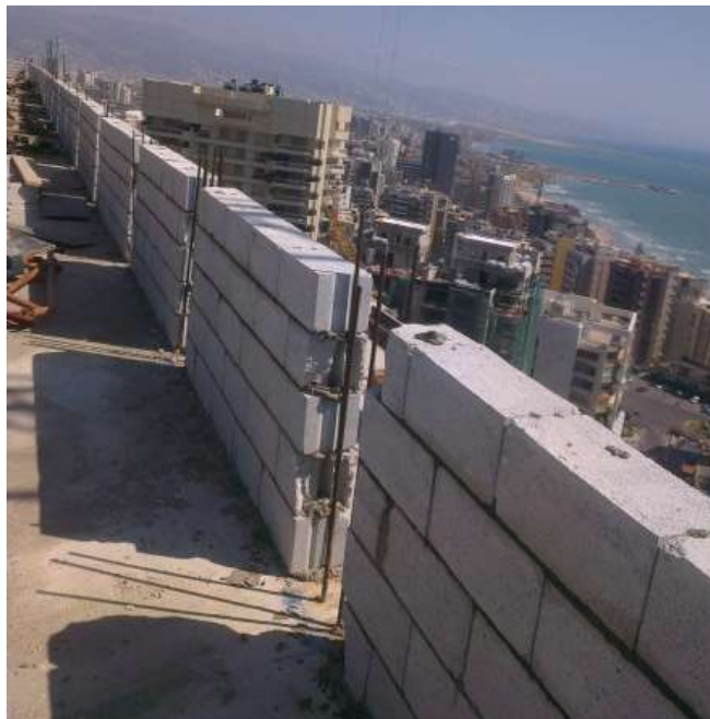
- Blockwork at roof level.
