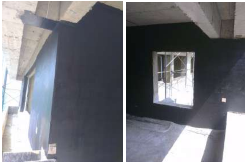
- External water proofing for cladding .
