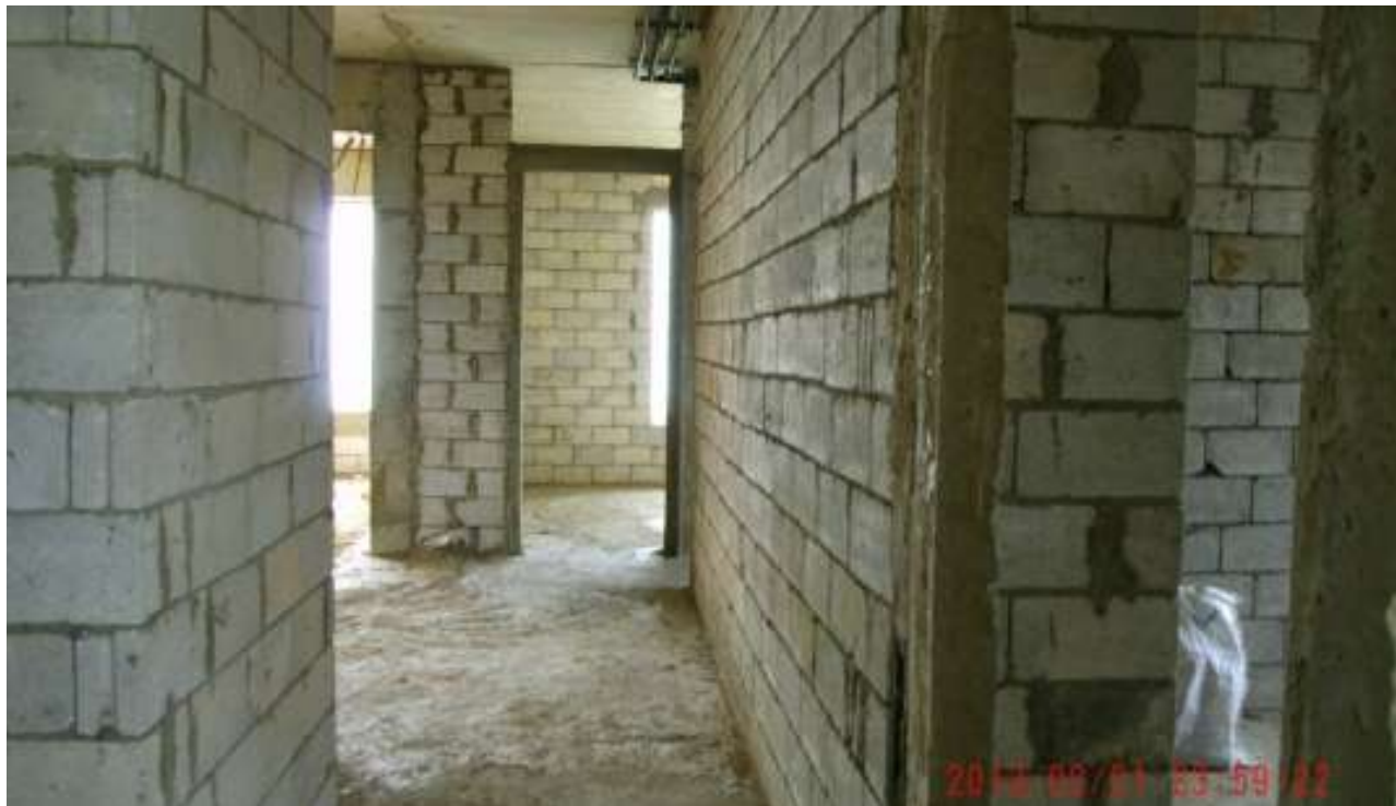
Block work done up to 12 th floor.
