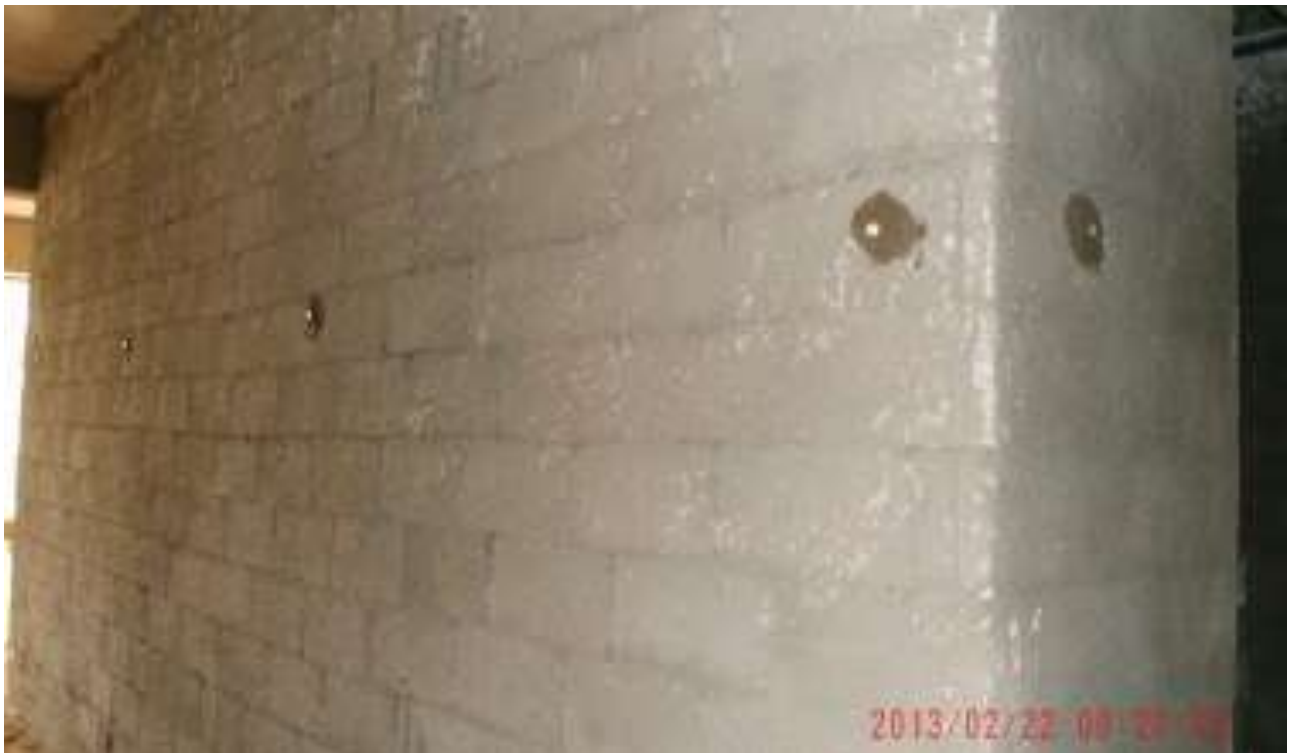
- Rush coat and plastering.
