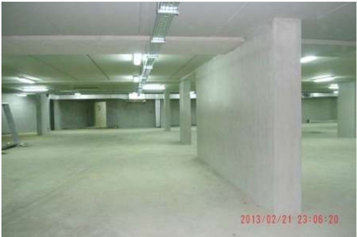
Cleaning and lighting for 3 basements floors
