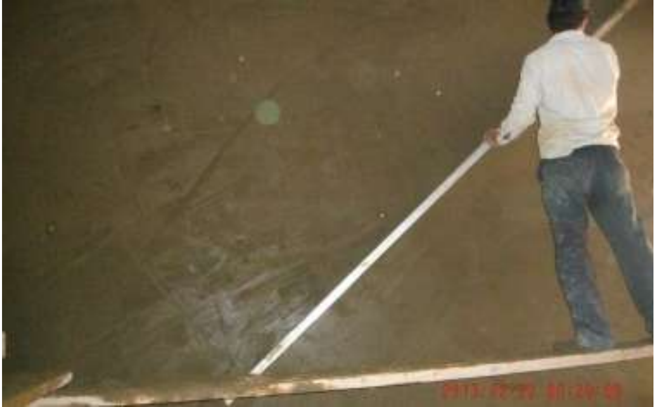
- Rush coat and plastering.
