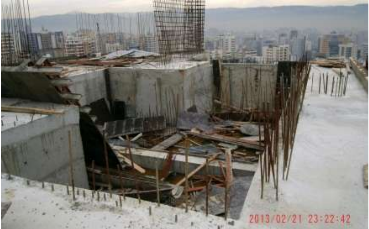
- Concrete casting – Swimming pool and verticals 17 th floor.
