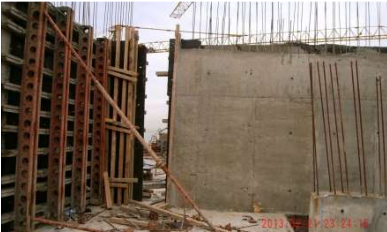
- Concrete casting – Swimming pool and verticales 17 th floor.
