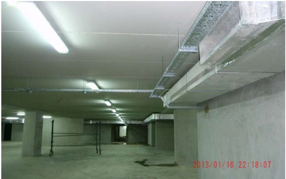
Ceiling paint done in 3 basements , walls ready for final epoxy paint.
