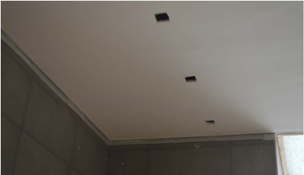
Figure 15: Ceiling and tiling works finalized @ 1st floor kitchen
