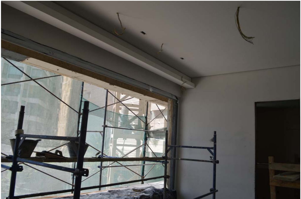
Figure 19: Aluminum subframes installations @ 1st floor
