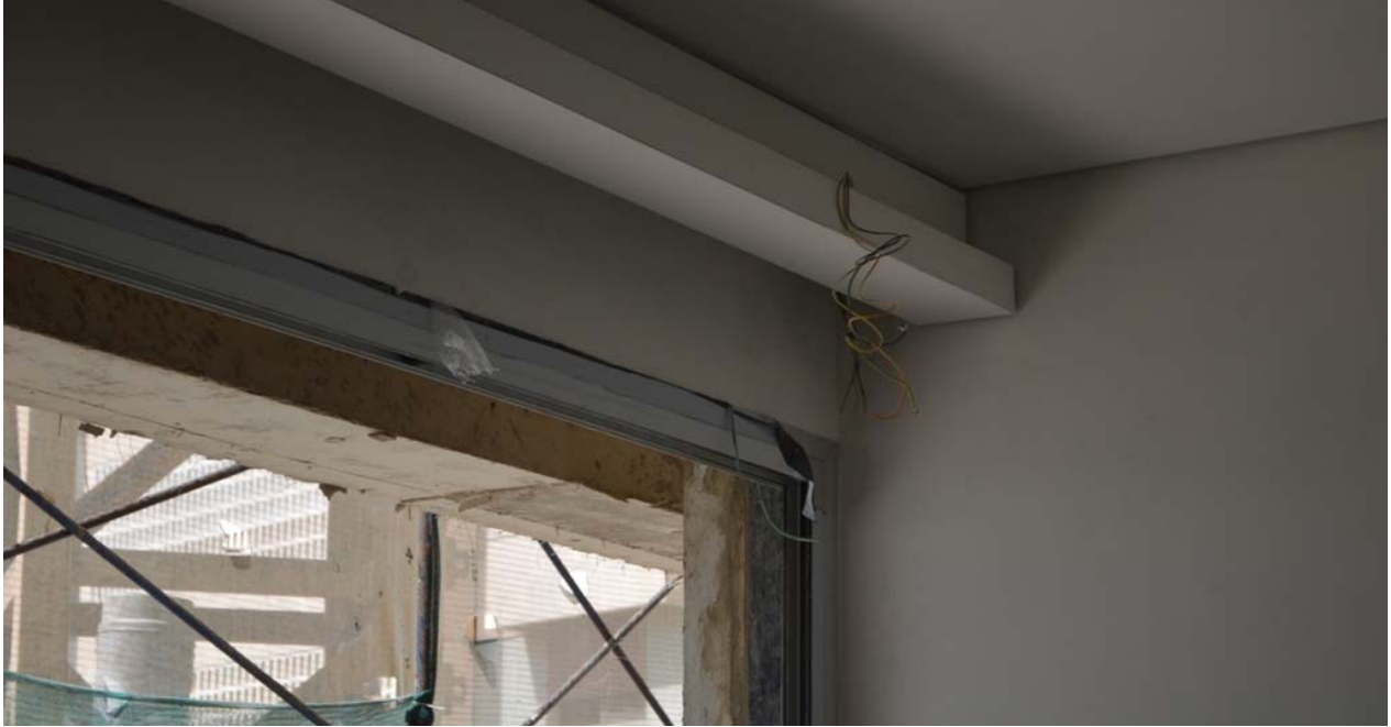
Figure 14: Aluminum subframes installed @ 1st floor
