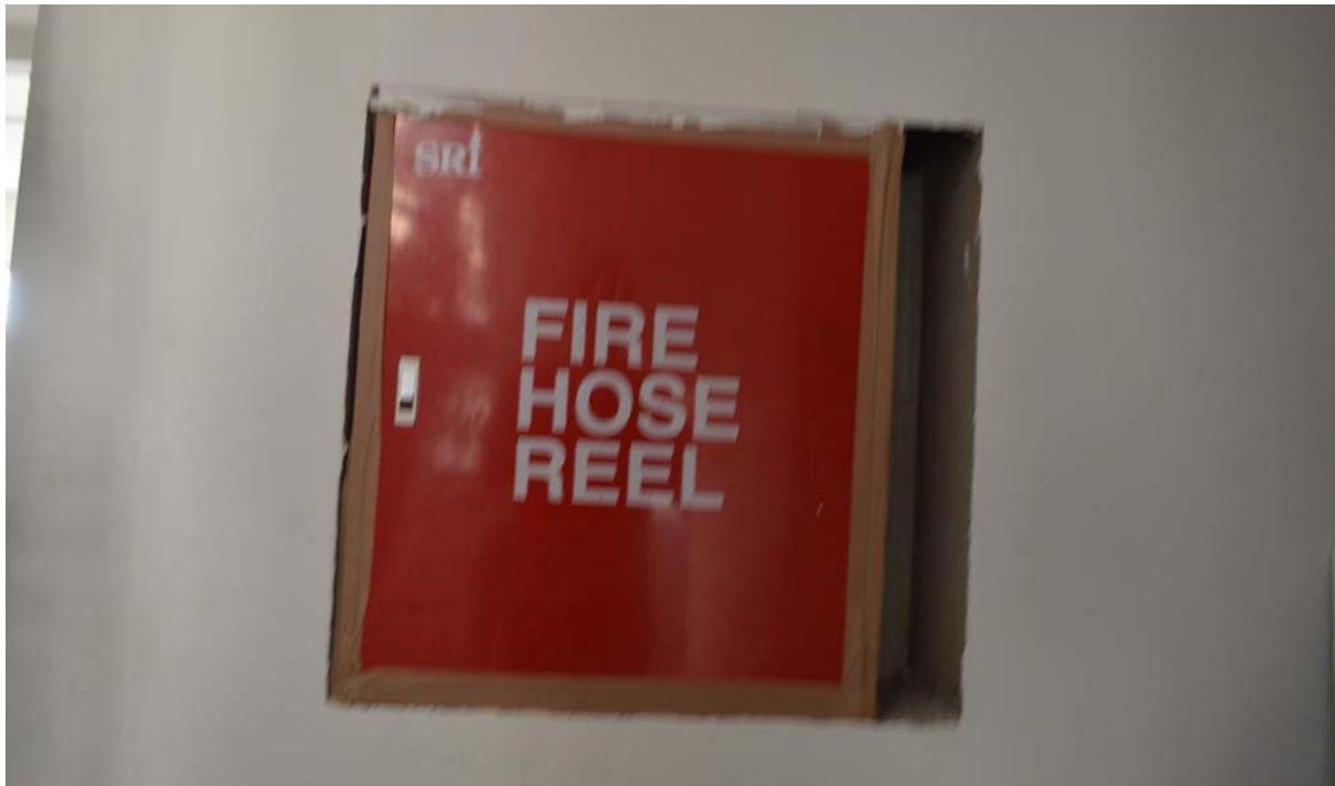
Figure 17, 18, 19: Mechanical installations finalized @ 1st floor (Outdoor units, fire hose reel)
