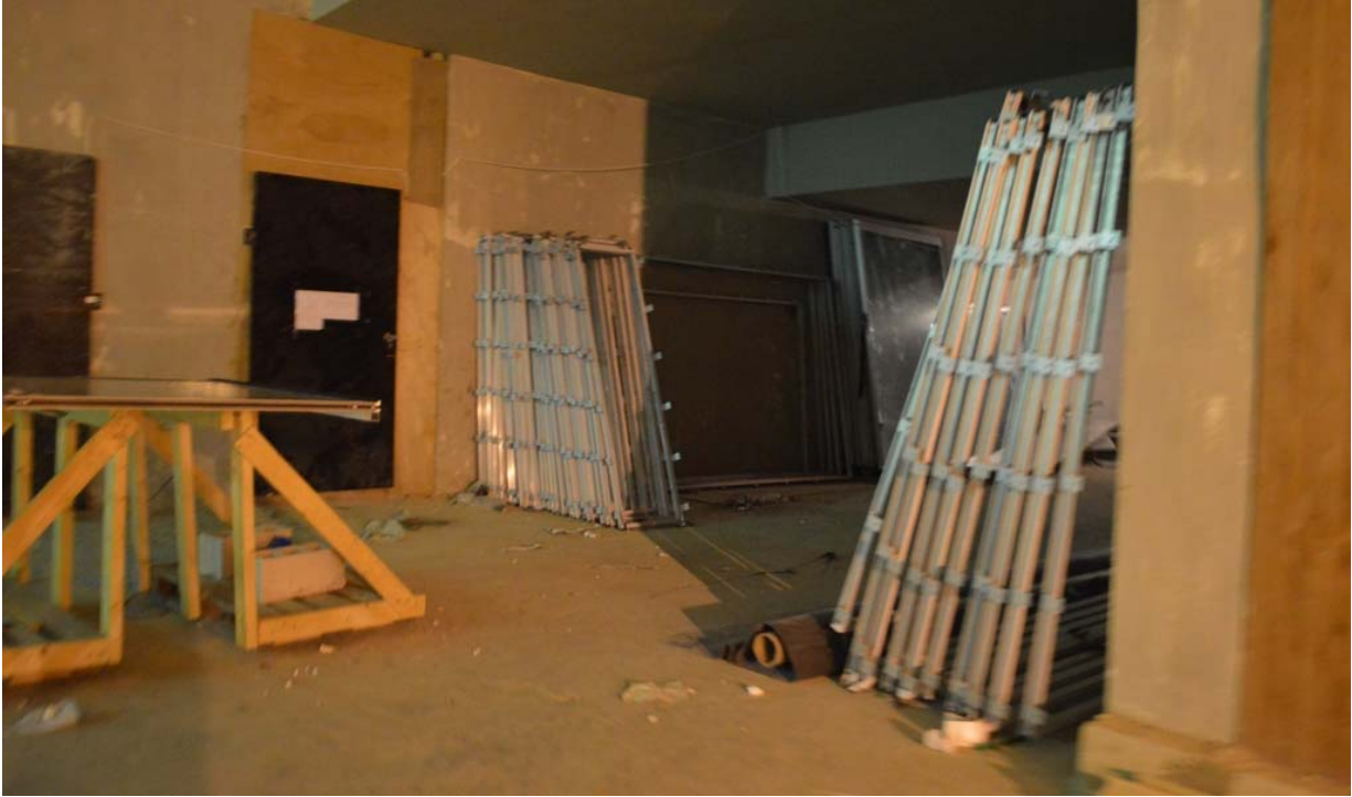
Figure 18: Remaining aluminum subframes ready for installation
