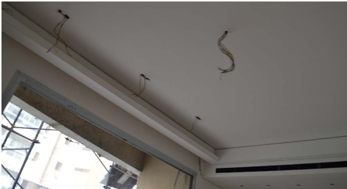
Figure 13: Gypsum and paint works @ 1st floor
