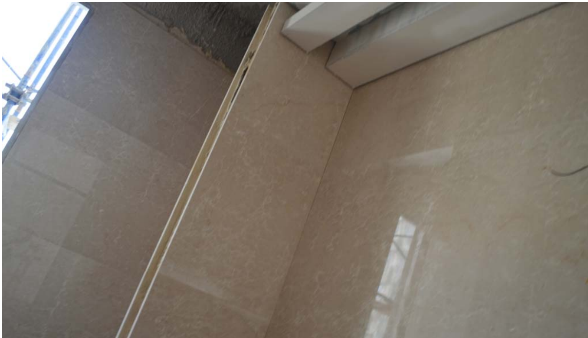
Figure 16: Marble tiling being finalized @ 1st floor bathrooms
