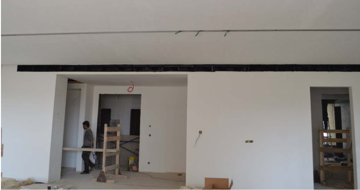
Figure 12: Gypsum and paint works @ 1st floor
