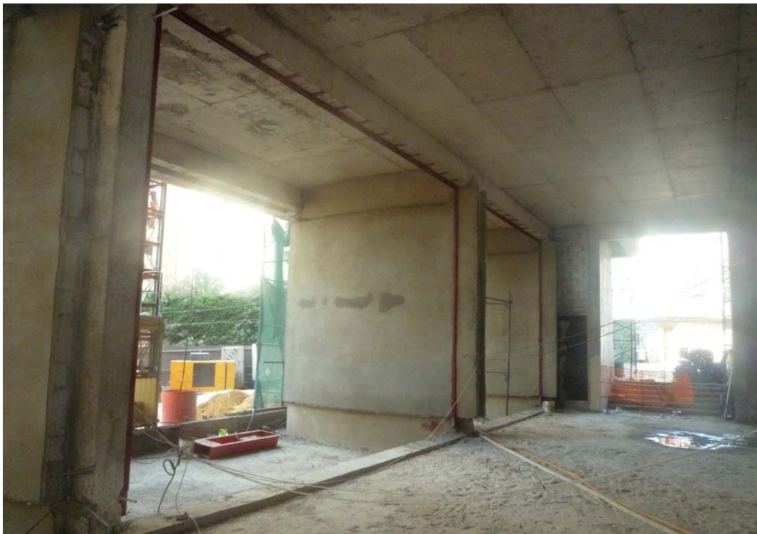
Figure 13: Metal works @ GF
