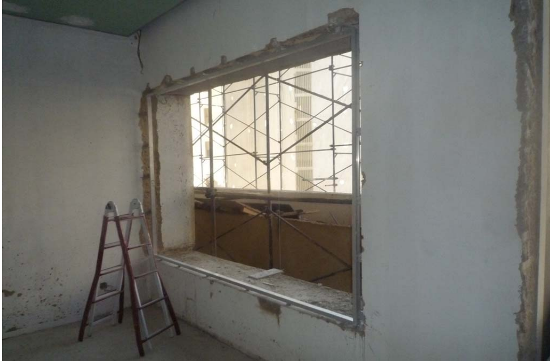
Figure 20: Aluminum subframes installed @ 1st floor
