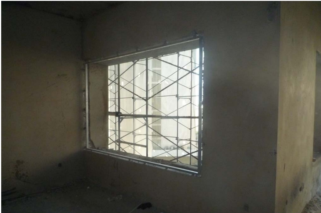
Figure 27: Aluminum subframes @ 2nd floor
