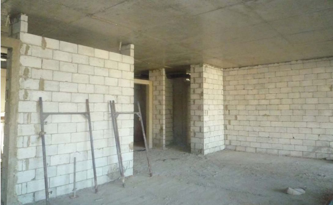
Figure 36: Blockwork @ 9th floor
