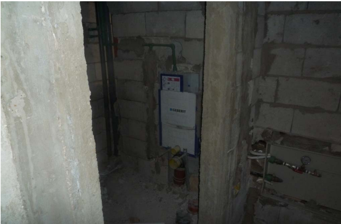
Figure 35: Plumbing works @ 9th floor
