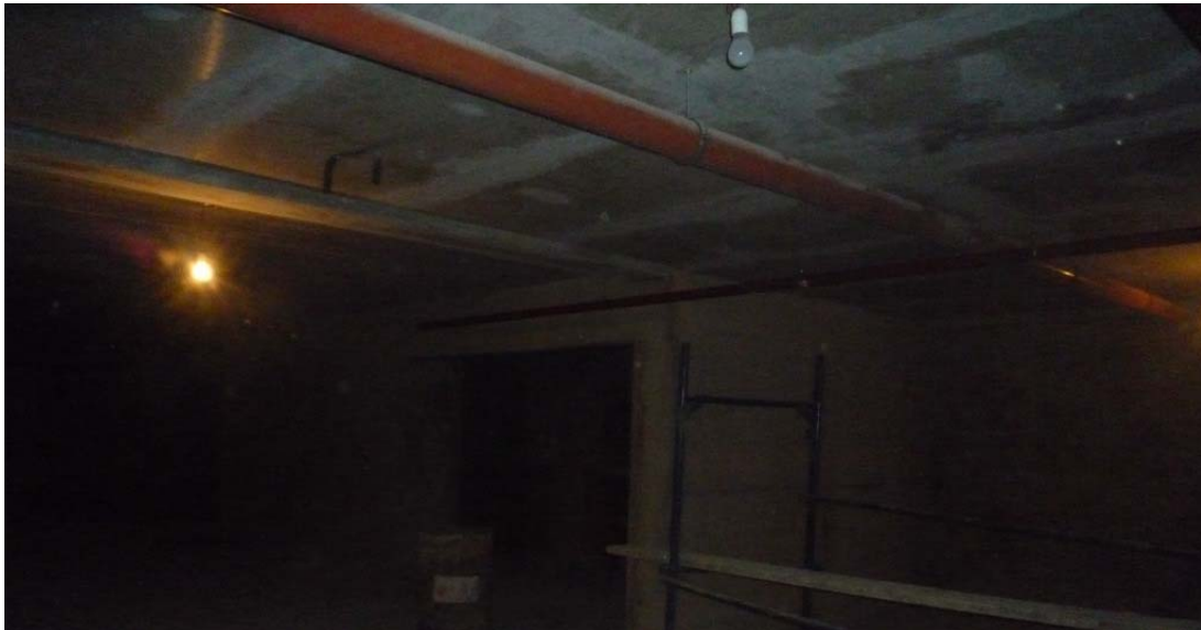
Figure 10: Mechanical works @ B3
