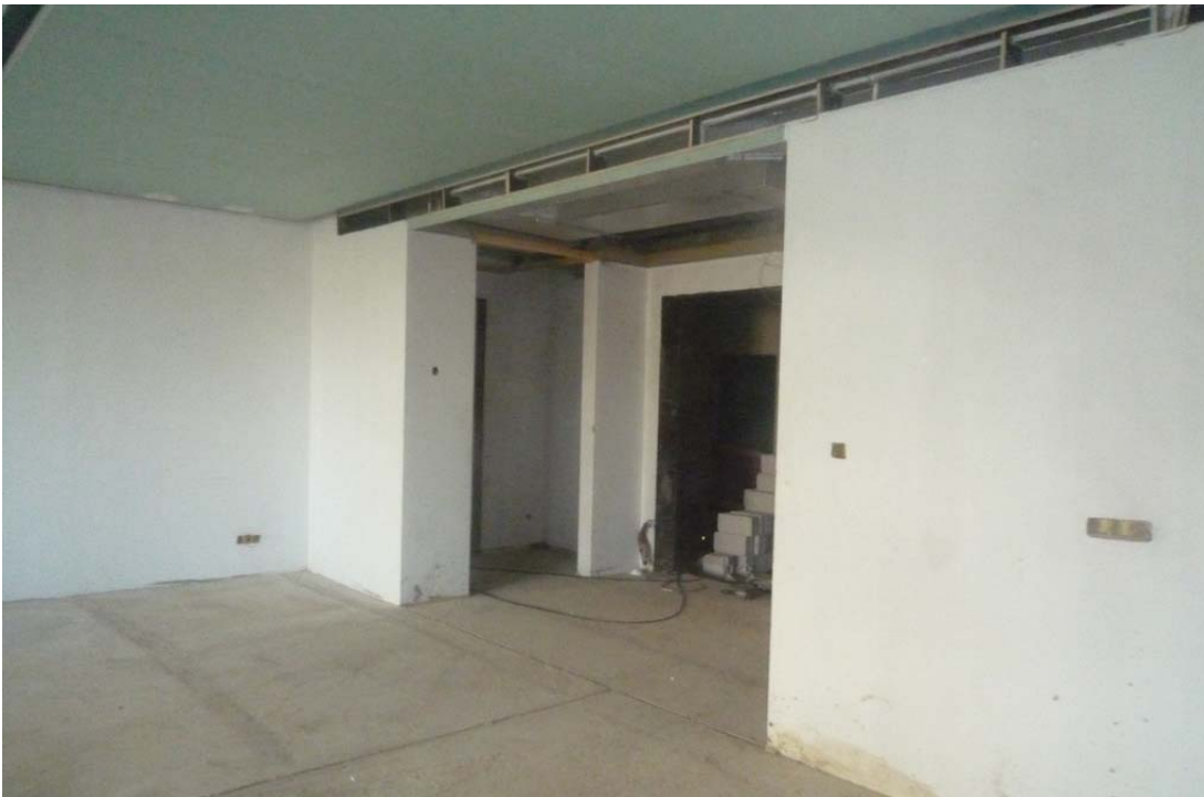
Figure 23: Screed poured @ 1st floor - ready for floor tiling
