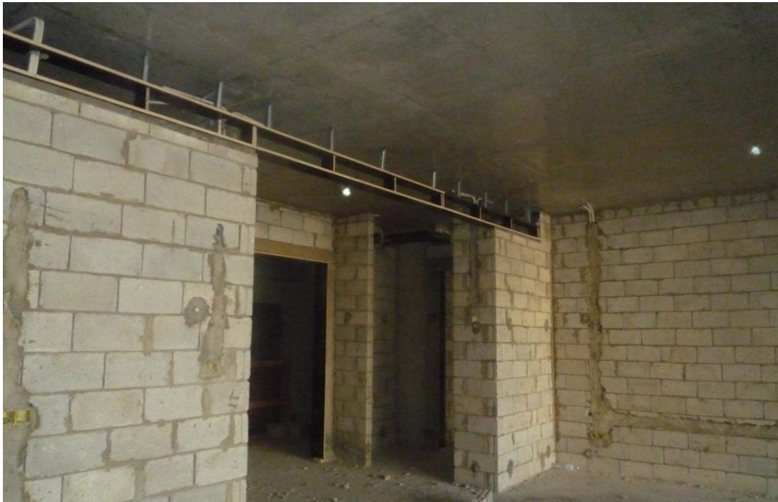
Figure 31: Blockwork @ 7th floor
