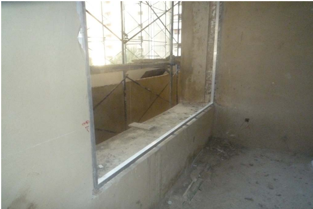
Figure 19: Aluminum subframes installed @ 1st floor
