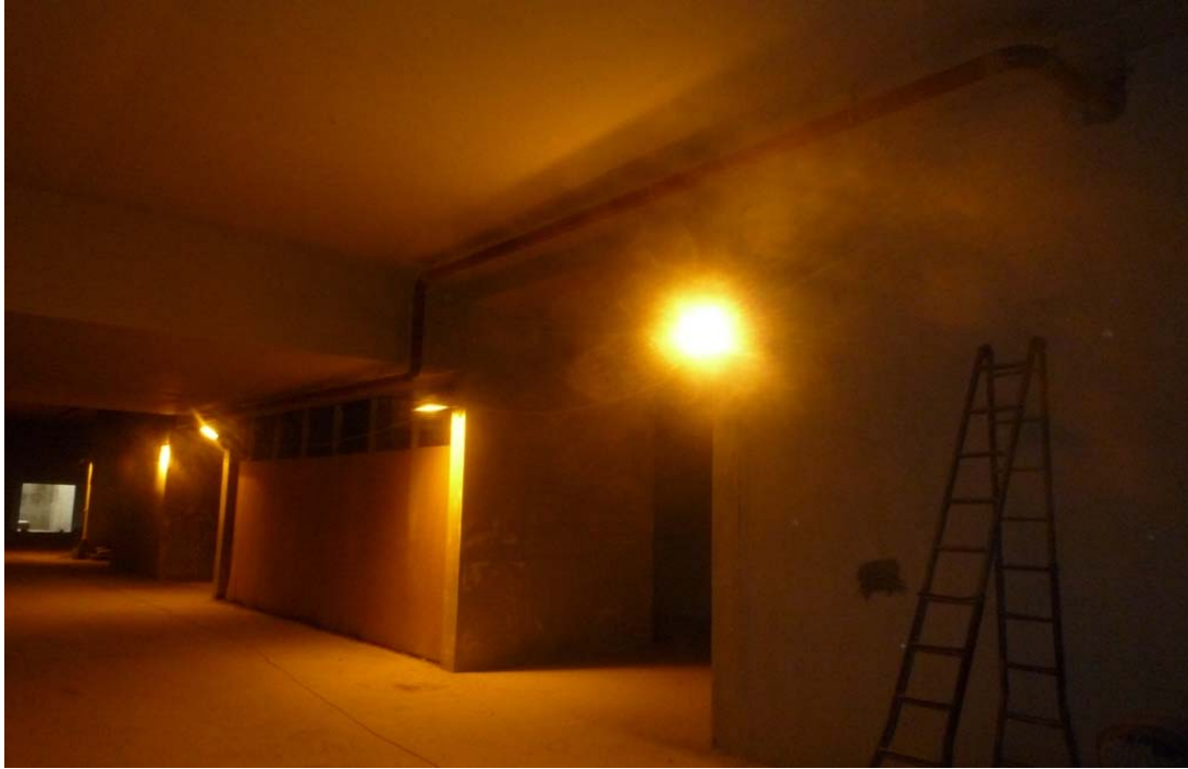
Figure 12: Mechanical works @ B1
