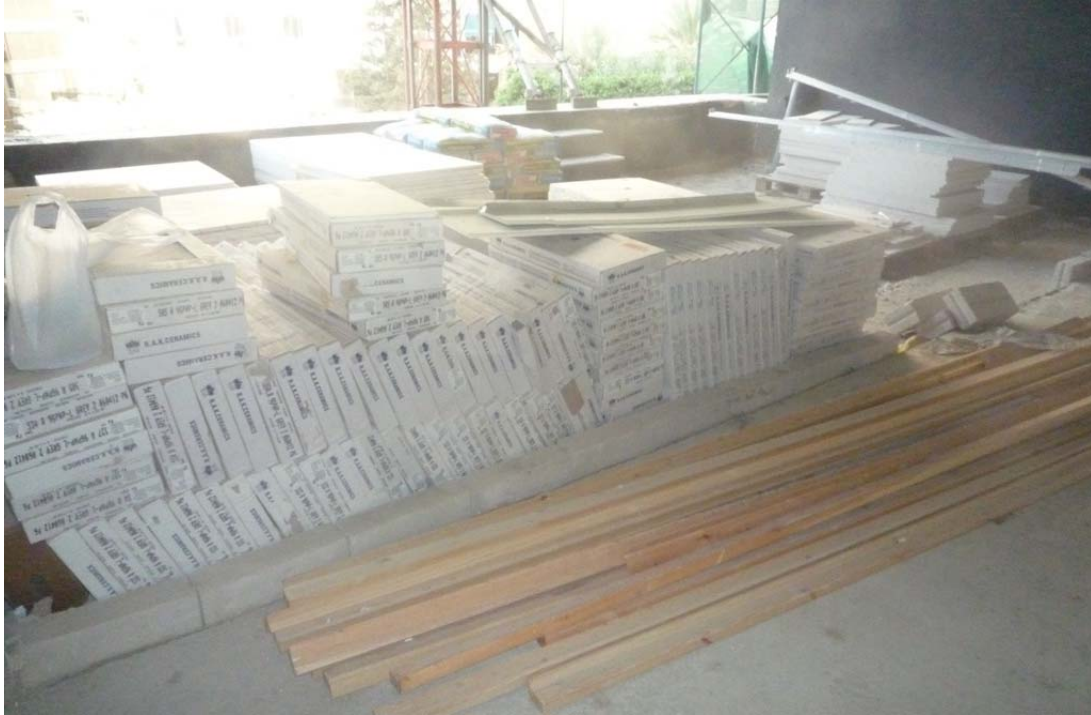
Figure 24: Ceramic and marble material ready on site for installation
