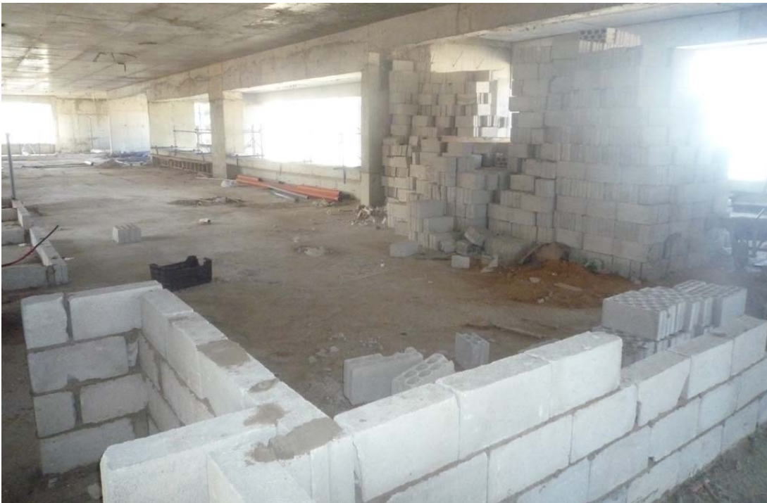
Figure 39: Blockwork initiation @ 10th floor
