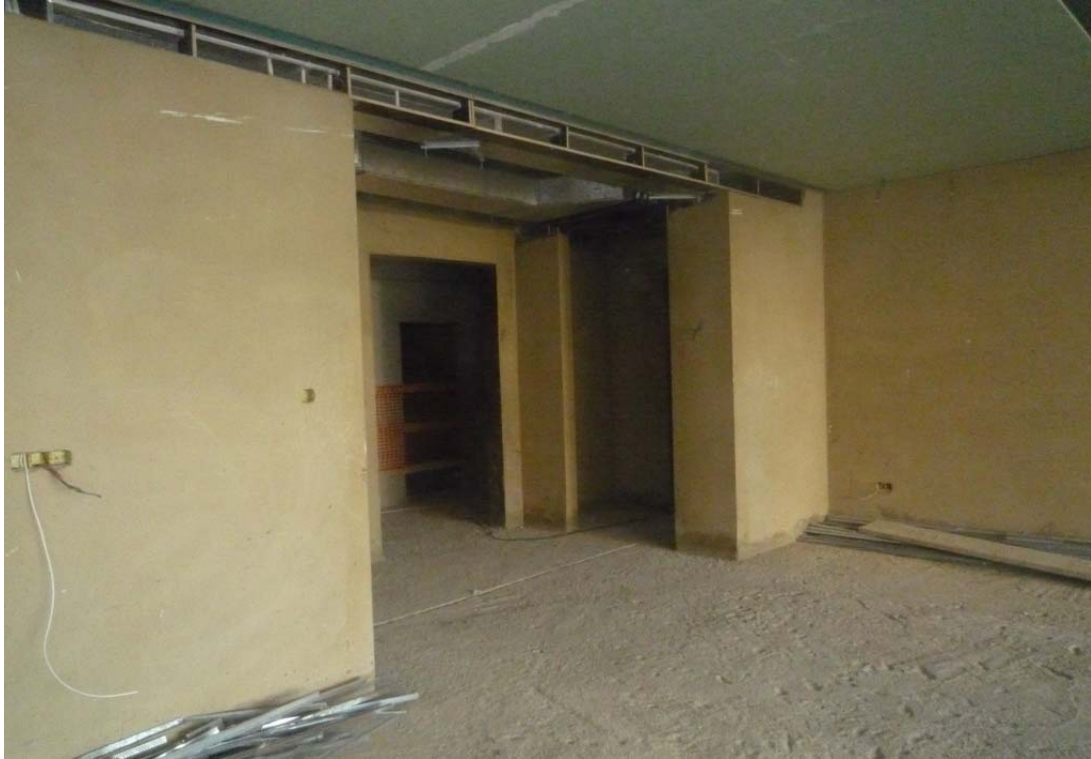
Figure 18: Screed poured @ 1st floor - ready for floor tiling
