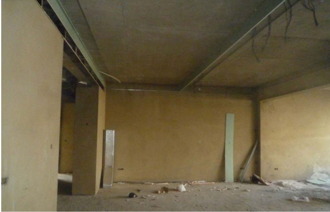
Figure 26: False ceiling works @ 2nd floor
