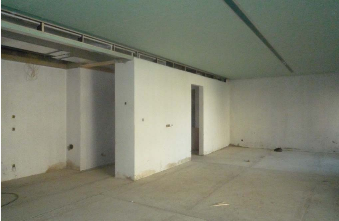
Figure 22: Screed poured @ 1st floor - ready for floor tiling
