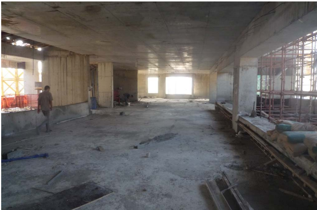
Figure 41: Concrete works @ 14th floor
