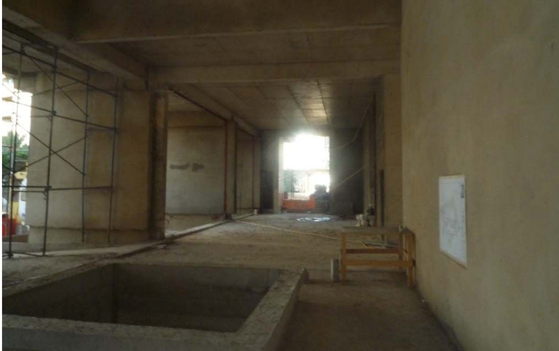
Figure 14: Blockwork and plastering complete @ GF
