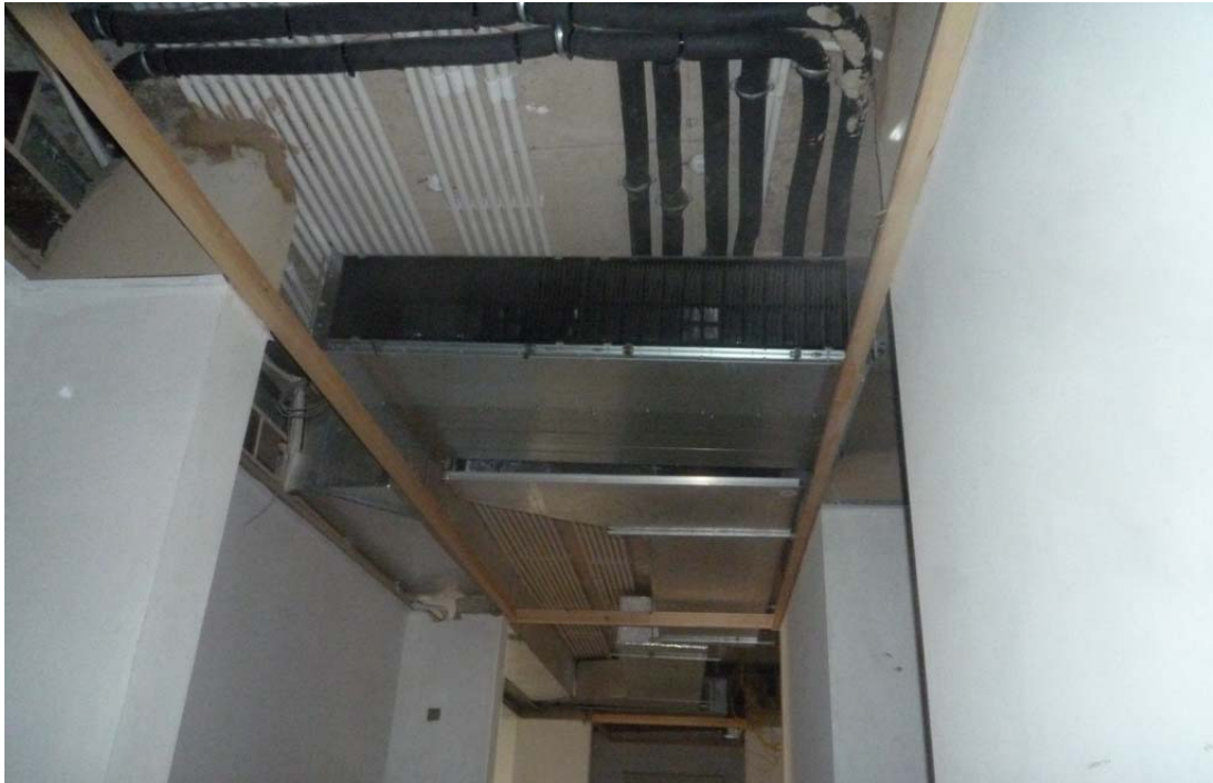
Figure 25: Wood access panels being finalized @ 1st floor
