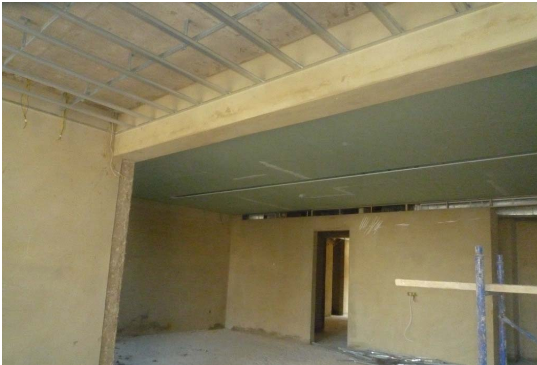
Figure 21: Ceilings works @ 1st floor
