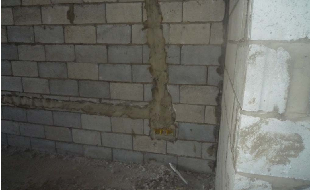
Figure 34: Electrical works @ 9th floor
