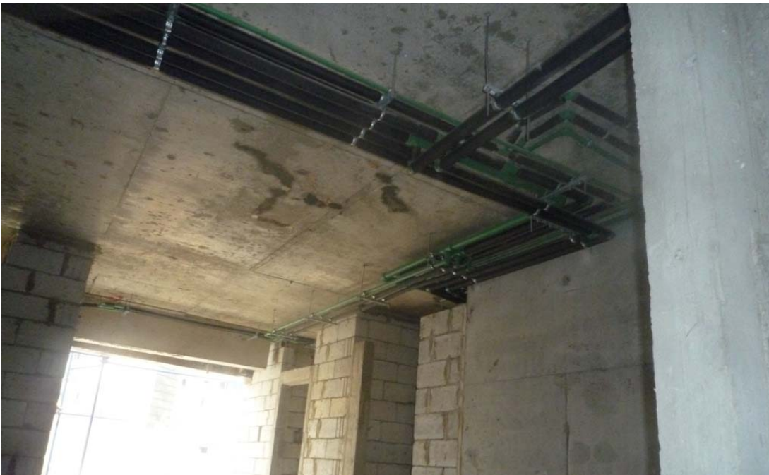
Figure 37: Plumbing works @ 9th floor
