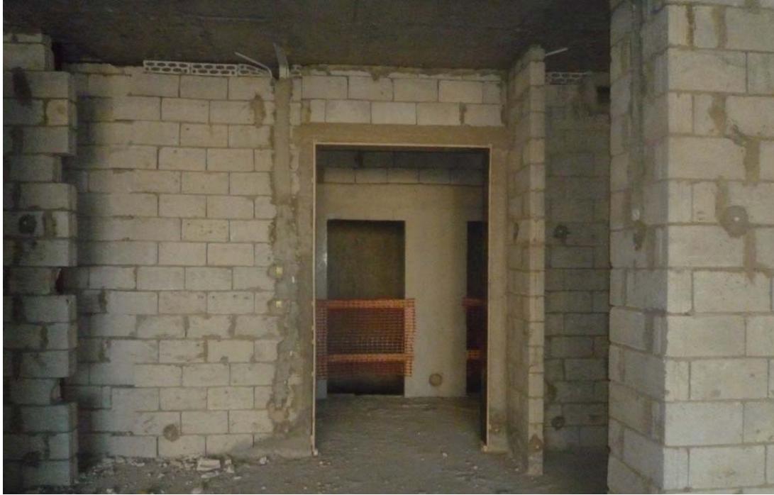
Figure 30: Blockwork @ 6th floor
