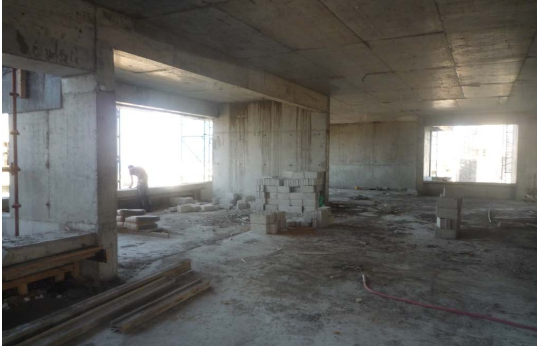
Figure 40: Concrete works @ 13th floor
