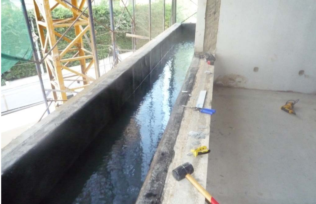
Figure 16: Waterproofing test @ 1st floor – flower beds
