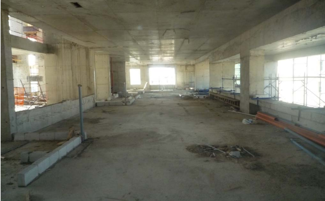
Figure 38: Blockwork initiation @ 10th floor
