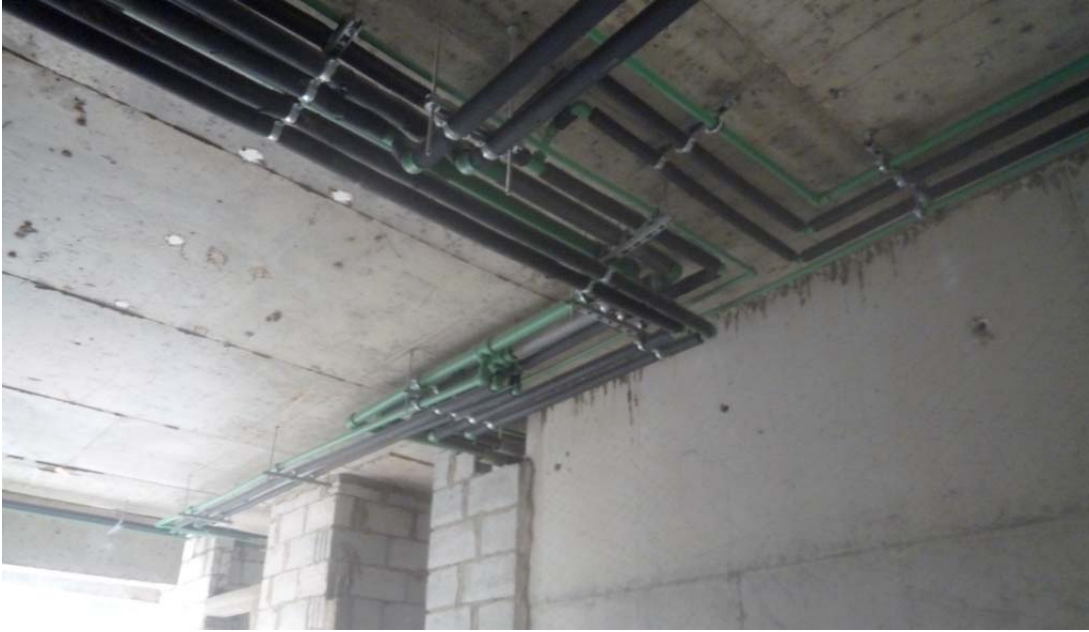
Figure 19: Mechanical works @2nd, 3rd and 4th floors
