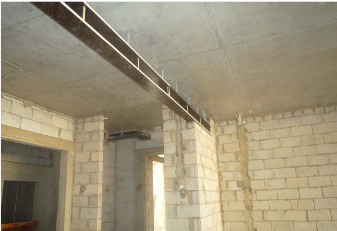
Figure 18: Duct openings complete @ 2 nd , 3 rd and 4th floors
