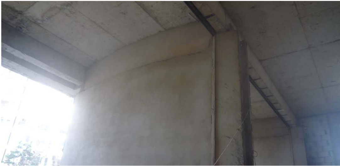
Figure 10: U-Channels installed in curved walls @ entrance
