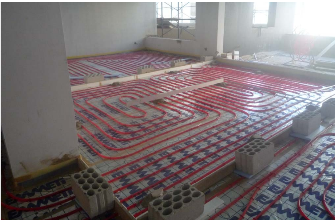
Figure 14: Underfloor heating installation @ 1st floor / reception and dining
