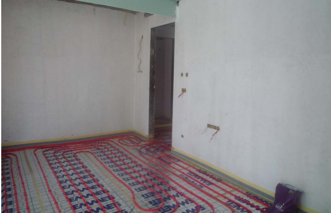
Figure 15: Underfloor heating installation @ 1st floor / bedrooms
