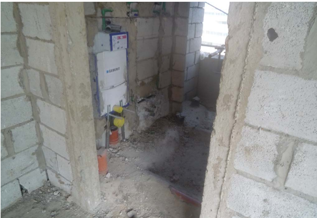
Figure 22: Sanitary works @ 7th floor
