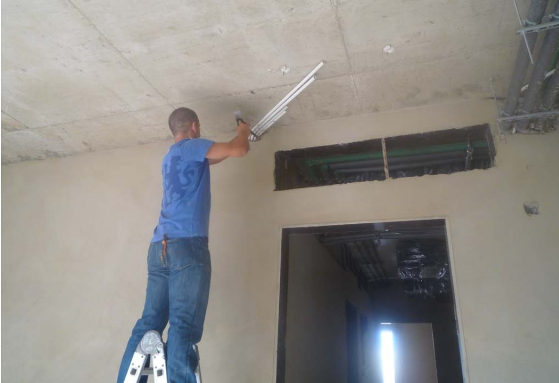
Figure 17: Plaster works being completed @ 2nd floor
