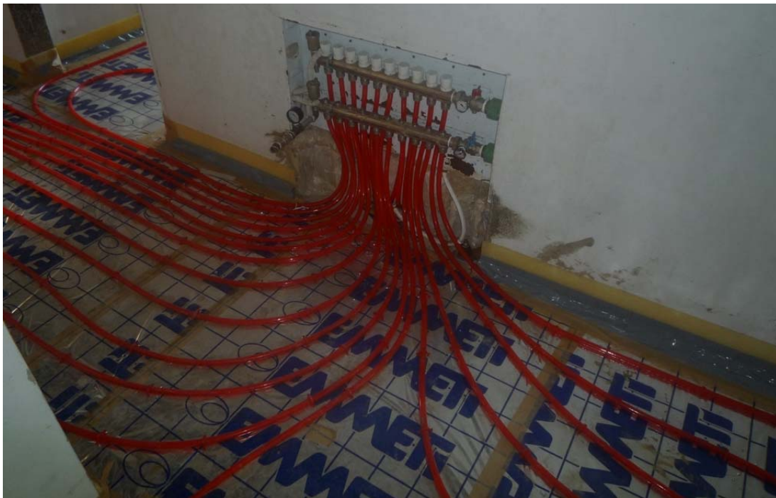
Figure 16: Underfloor heating installation @ 1st floor / corridor
