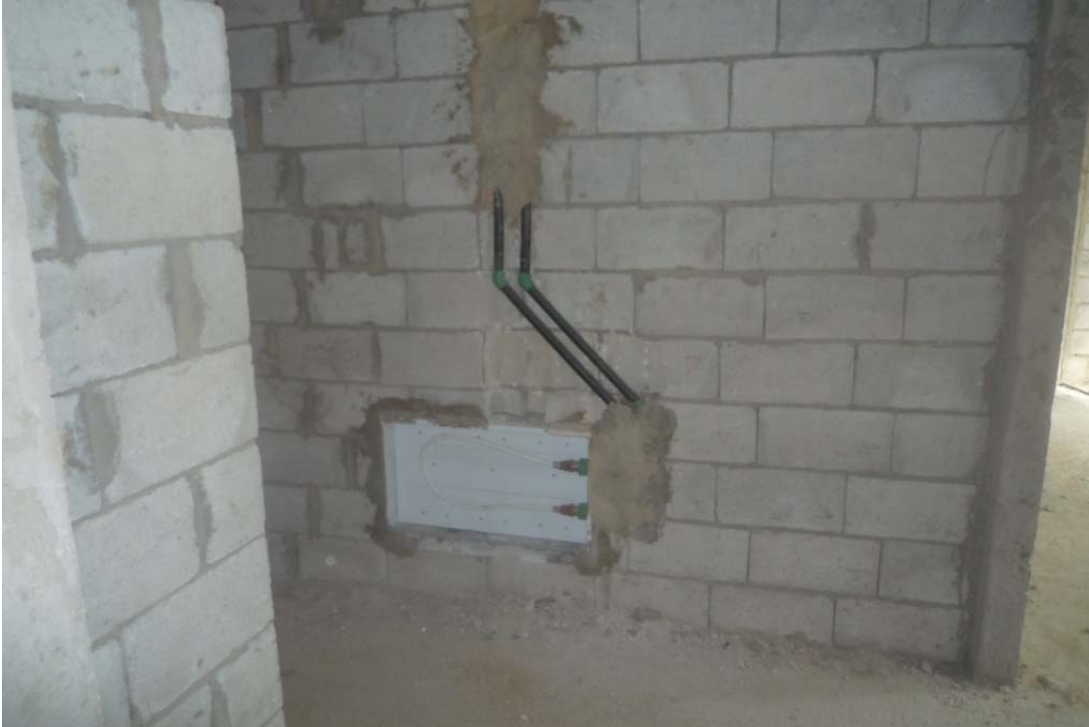
Figure 21: Electrical works @ 5th floor
