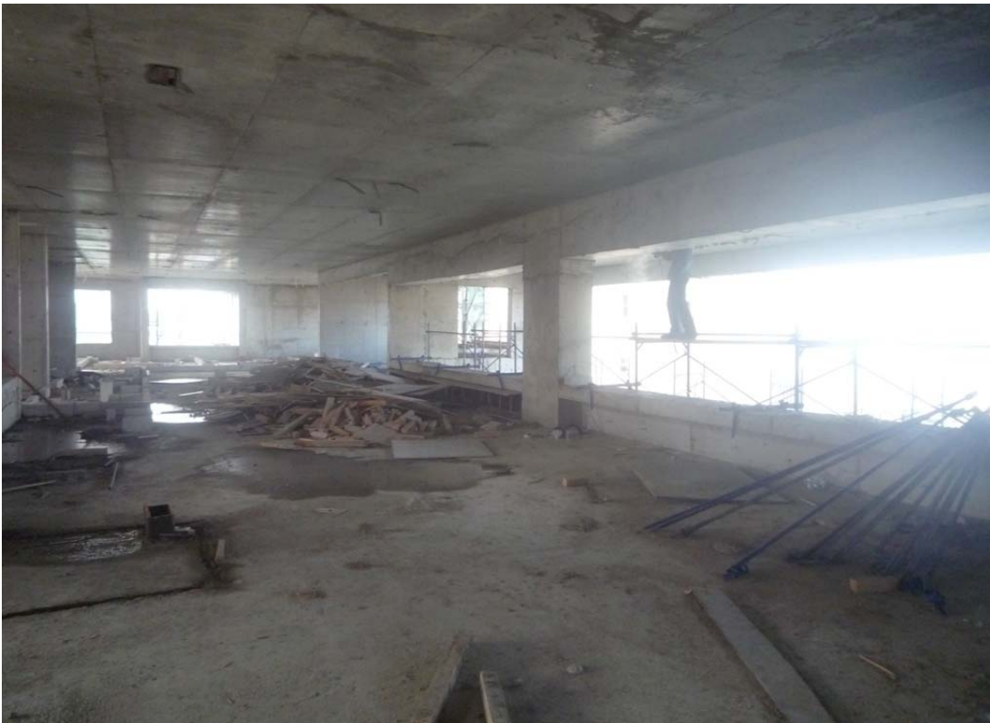
Figure 24: Concrete and block work @ 11th floor
