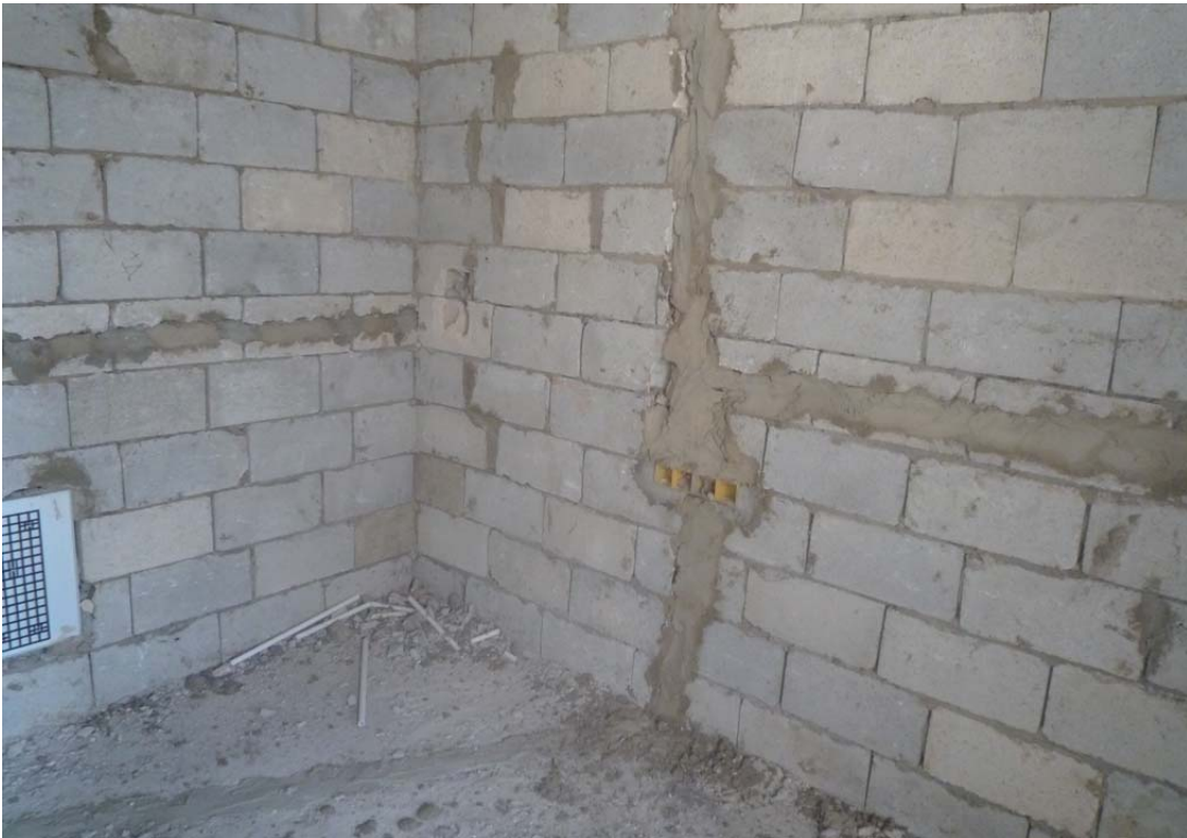
Figure 20: Electrical works @ 5th floor
