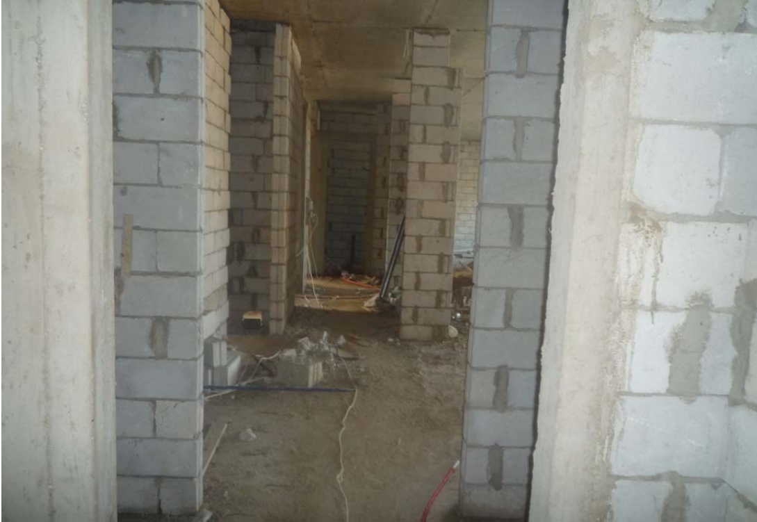
Figure 23: Blockwork @ 8th floor
