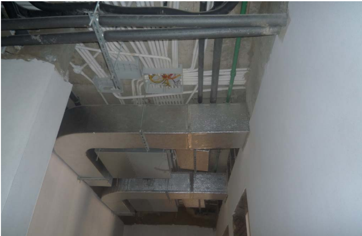
Figure 12: Ducting works complete in 1st floor
